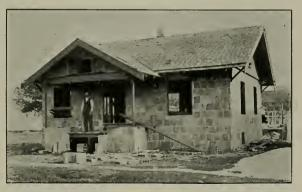
This Socramento bungalow was built of their hollow tile at the same cost as ils equivalent in wood. In a hundred ways it is superior to a wooden structure
