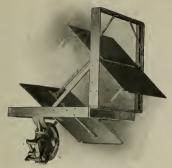
Mixing Damper with Attached Motor
