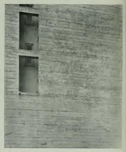
Reinforced Concrete Wall on Steel Frame Nine-Story Building. Wall Six Inches Thick. Cost to Owner 35 Cents a Square Faot of Surface.
