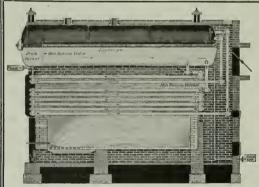
WITH many tubes in one header, the unequal expansion causes leaky joints. Rerolling thins the tube ends and means new tubes. In the design of a header holding but two tube ends each tube can expand without strain on header or joints. This is another feature of the
