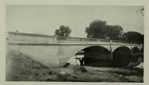
Three-Span Concrete Bridge at Plainfield Designed by Daniel B. Luten, C. E.
