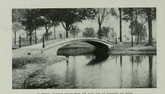
An Attractive Reinforced Concrete Bridge with 40 foot Span and Ornamental Iron Railing Designed by Daniel B. Luten, C. E.
