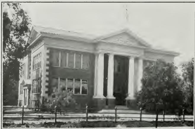
Lincoln Park Grade School, Los Angeles Norman F. Marsh, Architect
