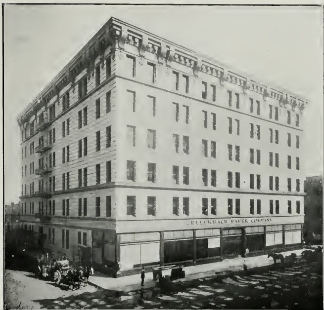
Zellerbach Warehouse, San Francisco
