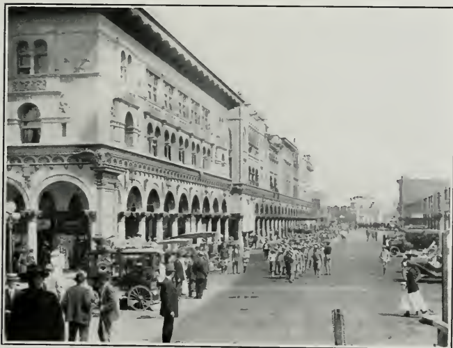
Winward Avenue, Venice, Southern California Norman F. Marsh, Architect
