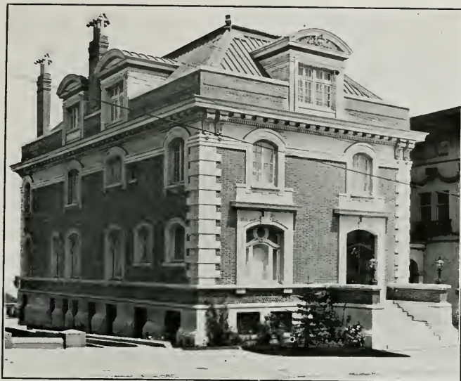
House of Dr. H. Kugeler, San Francisco T. Paterson Ross, Architect. A. W. Burgren, Engineer
