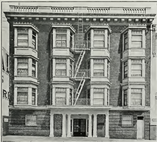
T. Paterson Ross, Architect Chatham Apartments, San Francisco A. W. Burgren, Engineer
