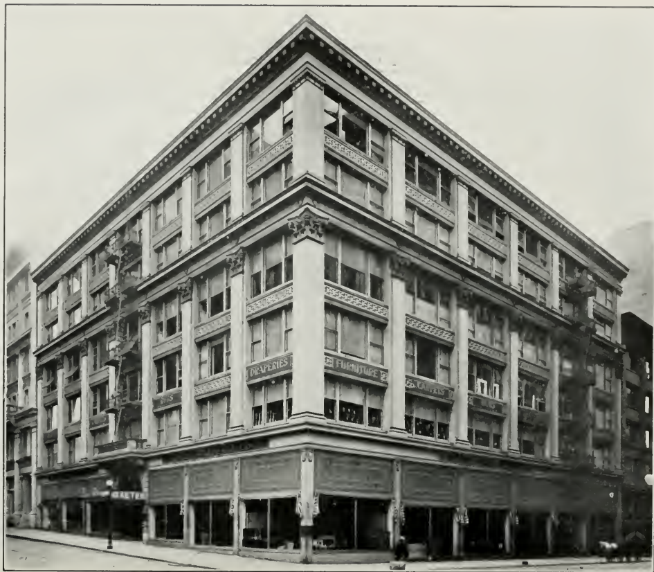
Shiel Estate Building, San Francisco
