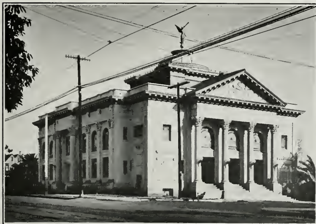
Park Place Methodist Church, San Diego Norman F. Marsh, Architect
