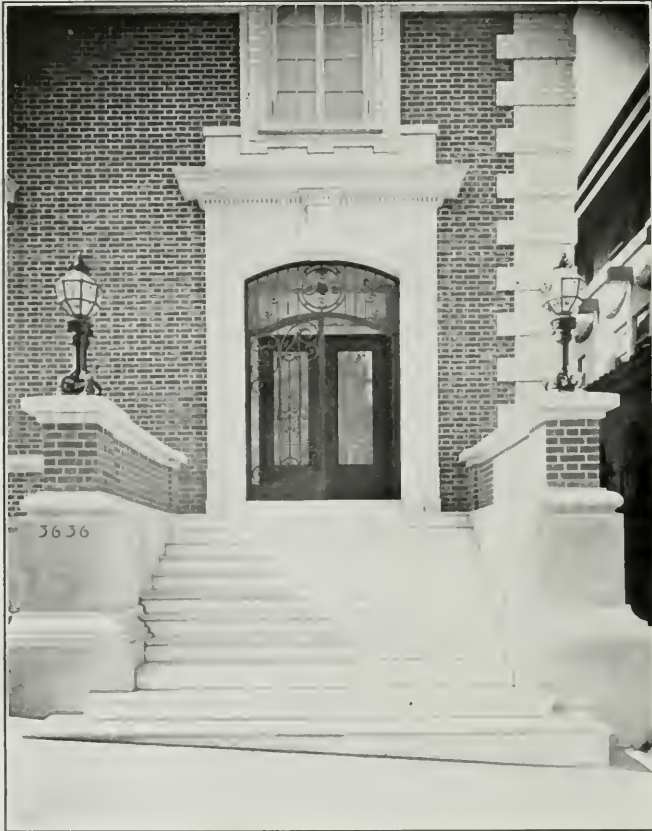
Entrance to Dr. Henry Kugeler's Residence, San Francisco. Ross & Burgren, Architects Bronze Standards and all Interior Lighting Fixtures Designed and Manufactured by Adams & Hollapeter, San Francisco
