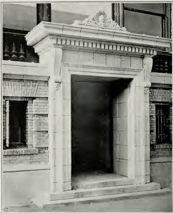
Entrance Girls' High School Building San Francisco Terra Cotta by Steiger Terra Cotta & Pottery Works
