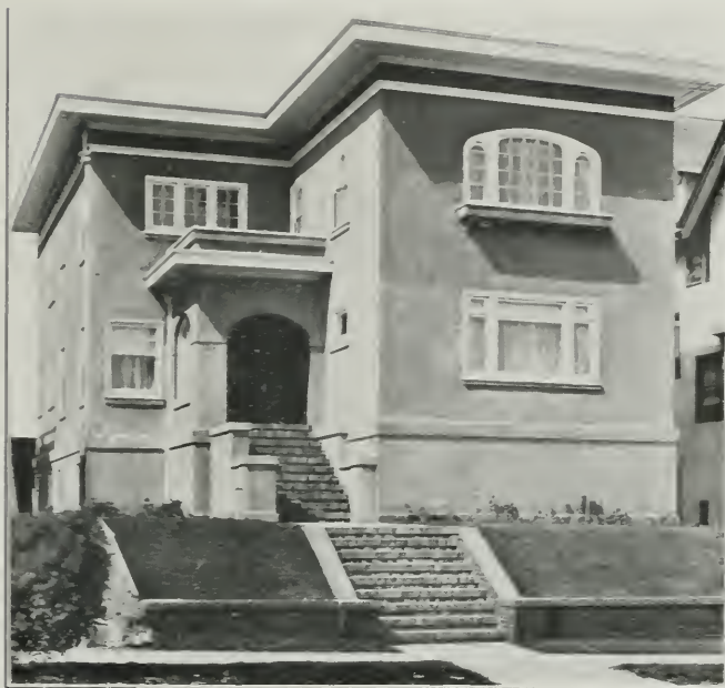
House of Mr. H. H. Young, San Francisco. T. J. Fisher, R. St. Anthony, Architects. A. H. Burgin, Engineer. Wiring by American Electrical Eng. Co.
