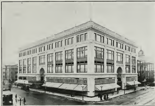
Capwell Department Store Building, Oakland C. W. Dickey, Architect
