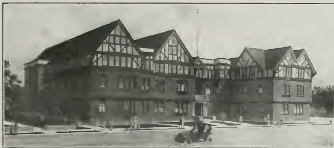
Anstone Apartments, Oakland, Cal. Louis S. Stone and Henry C. Smith, Architects
