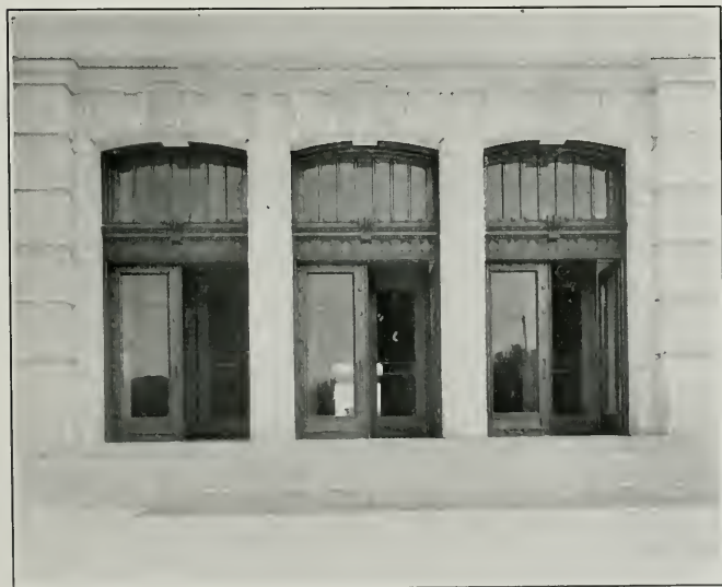
Entrance, Kern County Court House
