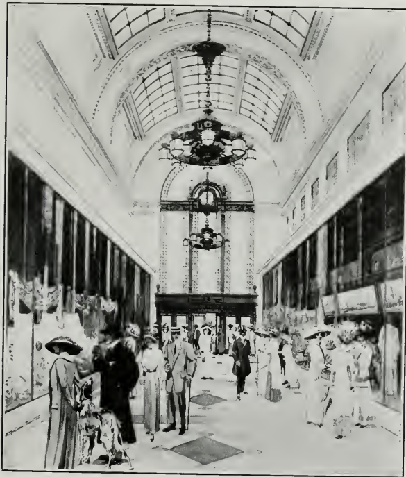
Arcade in Kahn Department Store, Oakland C. W. Dickey, Architect
