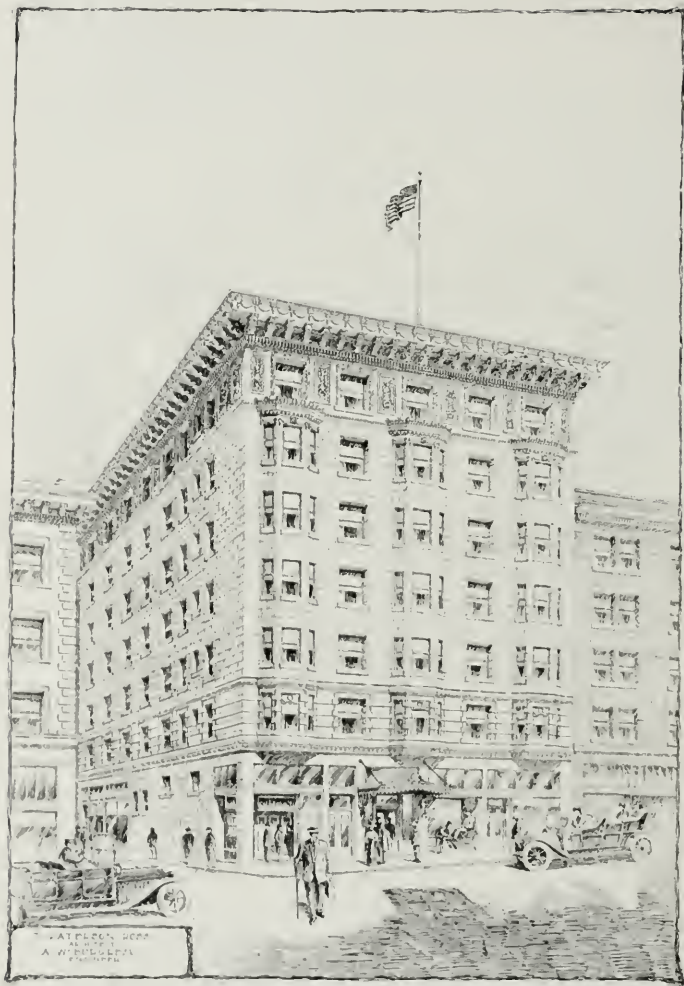
Berg Hotel, San Francisco J. Paterson Ress, Architect. A. W. Burgren, Engineer
