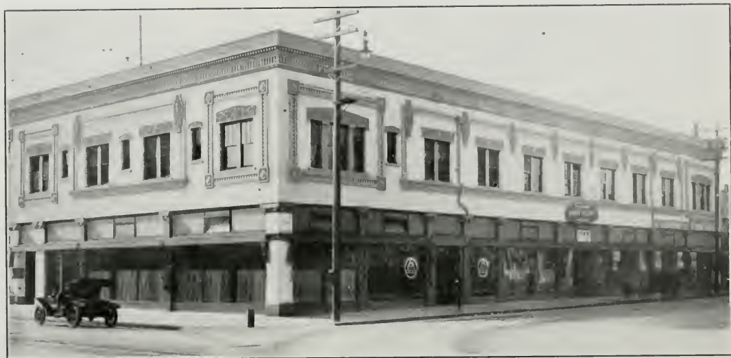
Stores and Apartments, San Jose
