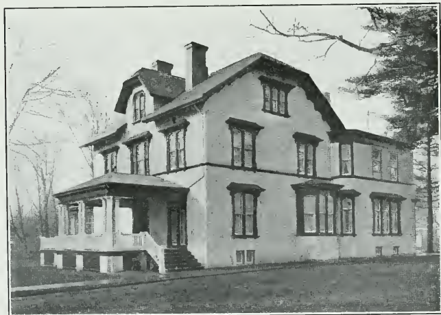
The Same House After Receiving a Coat of "Gunit"
