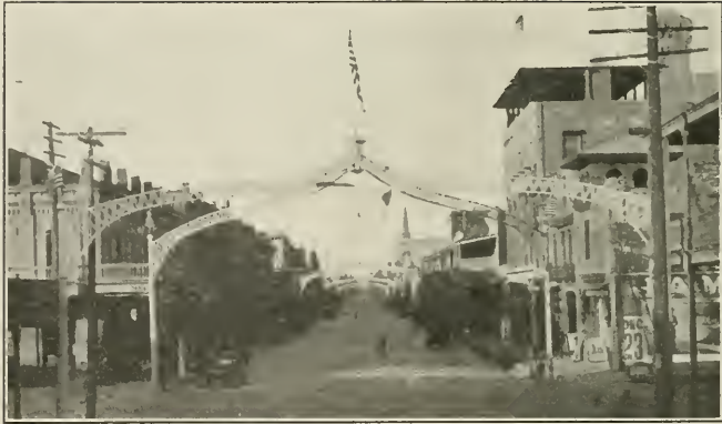
Steel Arches for Street Illumination, Marysville, California
