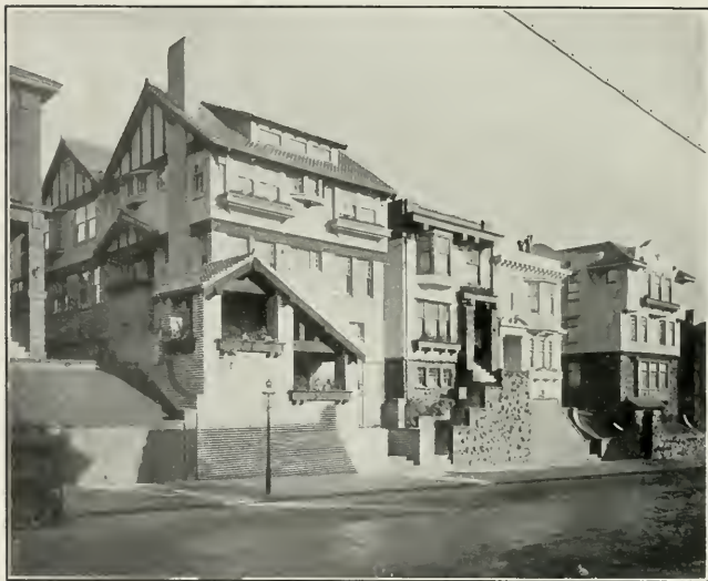
A Row of High Class City Flats, San Francisco Henry C. Smith, Architect
