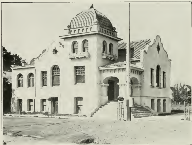
Carnegie Library, Haywards, California Designed by Henry C. Smith, Architect
