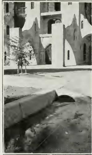
Corrugated iron culvert at Riverside, California, installed in front of famous Glenwood Mission Inn
