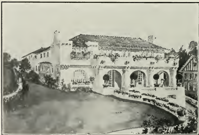
Residence of Mr. E. D. I. Johnson, Presidio Terrace, San Francisco Henry C. Smith, Architect Geo. W. Boston, Contractor
