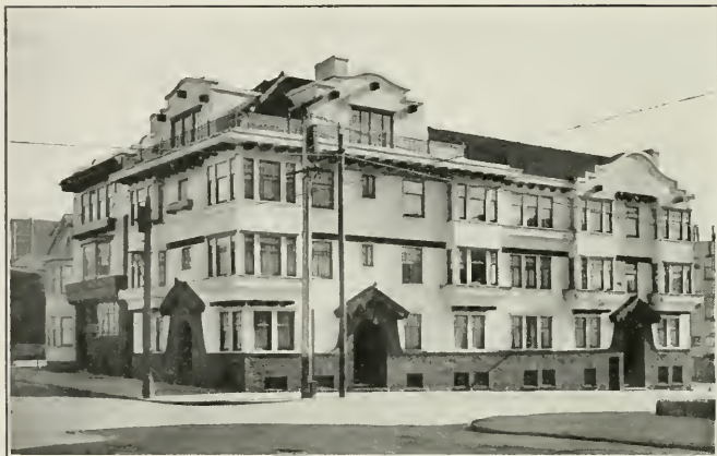
The Lackmann Apartments, San Francisco
