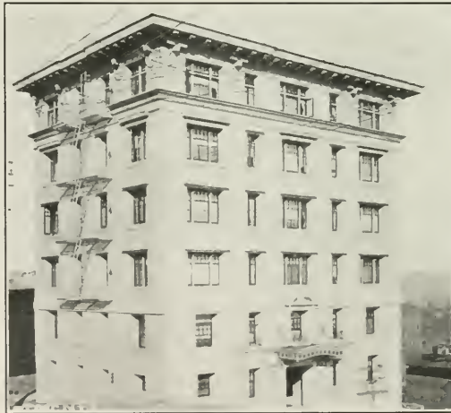
Leesmont Apartments, San Francisco Henry C. Smith, Architect
