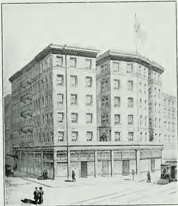
Apartment House for Marion Leventritt, San Francisco G. A. Lansburgh, Architect
