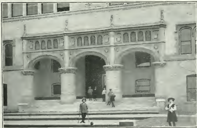
Entrance to Franklin School Building, Oakland, California. Designed by Henry C. Smith, Architect
