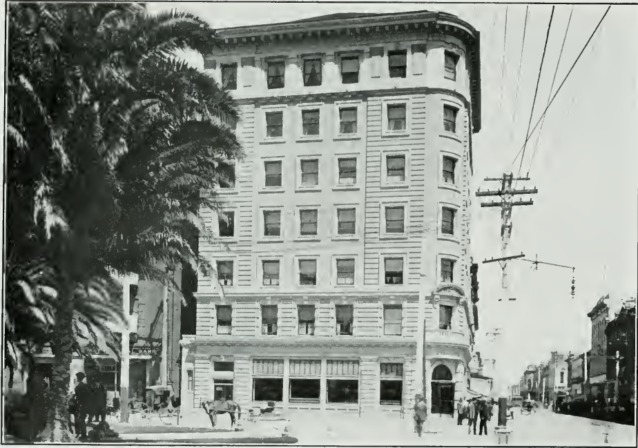
Savings and Loan Society Building, Stockton, California
