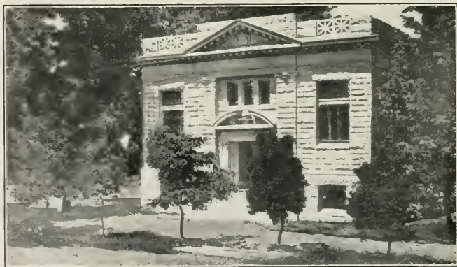
Colusa Library Building, Colusa, California Designed by Henry C. Smith, Architect
