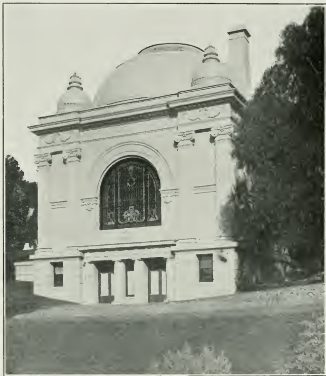
Remodeled Crematory at Cypress Lawn Cemetery, San Francisco Henry C. Smith, Architect
