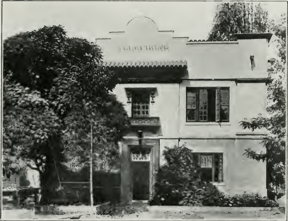
Exchange Building at San Bernardino, California
