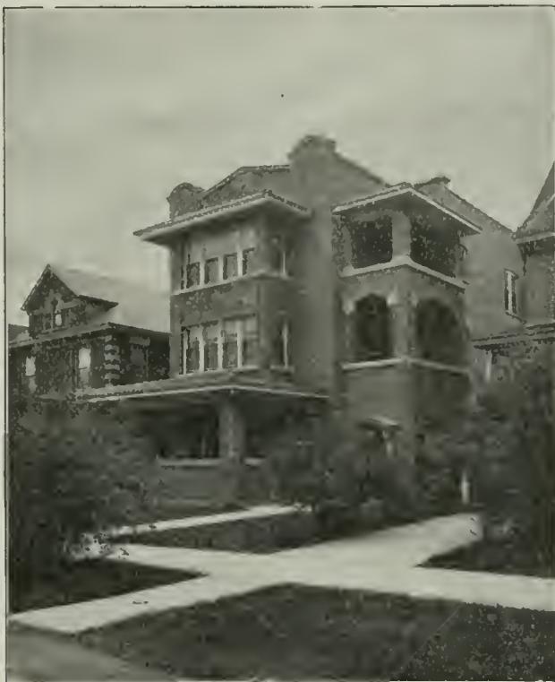
Ceresit Waterproofing was used in this Apartment Building 4639 Beacon Street, Chicago
