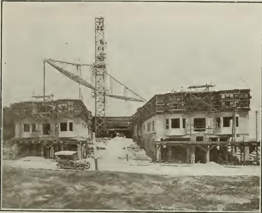
Construction Work on the Barlow Building, Los Angeles
