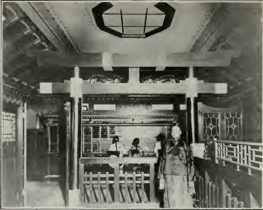
Interior of Chinatown Telephone Exchange, San Francisco, California
