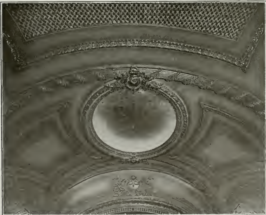
Detail of Ceiling, Orpheum Theater, Los Angeles
