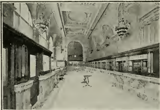
Interior of Banking Room, London Paris National Bank, San Francisco Albert Pissis Architect
