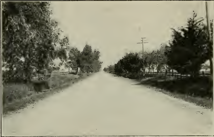
Lower Sacramento Road, Paved under County Bond Issue
