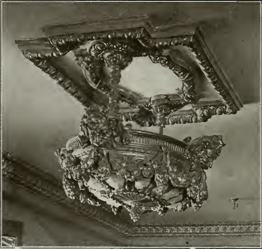
Indirect Lighting Fixture in Main Lobby, Orpheum Theater, Los Angeles All Fixtures Manufactured and Installed by Thomas Day Company, San Francisco G. Albert Lansburgh, Architect
