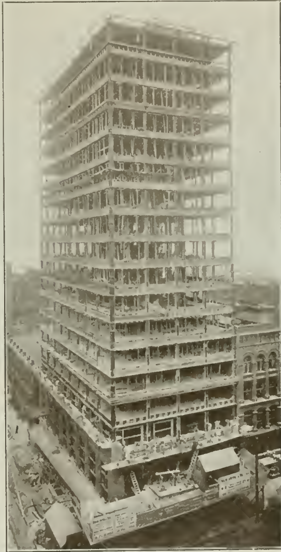
Hogue Building, Seattle, Wash. Thompson Starrett Company, Contractors.
