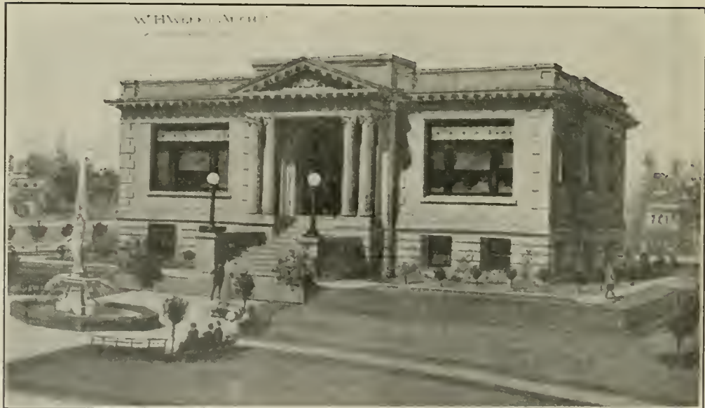
CARNEGIE LIBRARY, LIVERMORE, CALIFORNIA William H. Weeks, Architect
