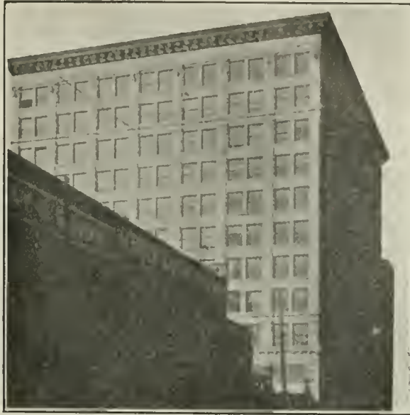
Higgins Building, Los Angeles. A. L. Haley, Architect. A. C. Martin, Engineer. A. Barman, Contractor
