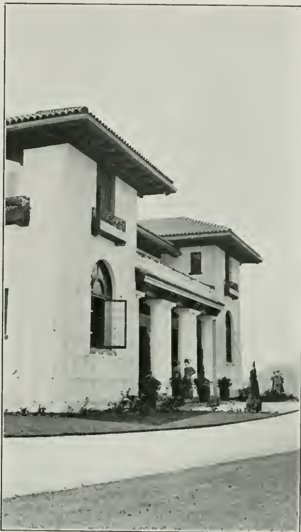
Driveway and Front Entrance to Mr. Wm. T. Sesnon's House, Aptos, California
