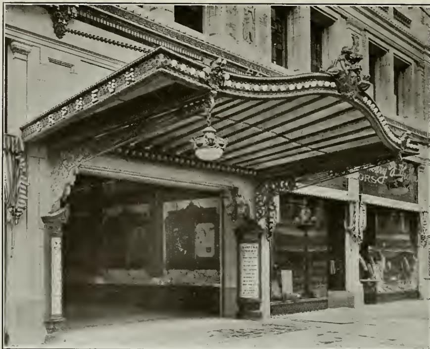
Marquise of Orpheum Theater, Los Angeles Executed in Cast Iron by California Artistic Metal and Wire Co., San Francisco G. Albert Lansburgh, Architect
