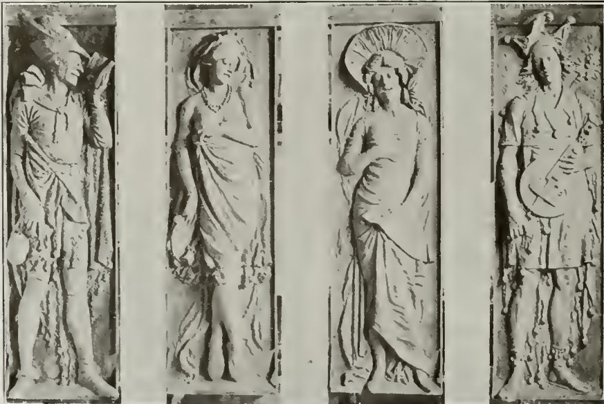
Comedy Dance Song Music Four Panels on Exterior of Orpheum Theater, Modeled by Domingo Moro, and Executed in Architectural Faience by Gladding, McBean & Company G. Albert Lansburgh, Architect
