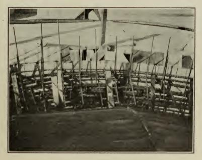
Reinfercing Rods for Concrete Water Tower, Palo Alto, California
