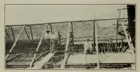
Another View Showing Steel Reinforcement of Reservoir Walls
