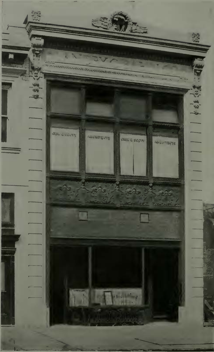
Landry C. Babin Building, San Francisco Crim & Scott, Architects
