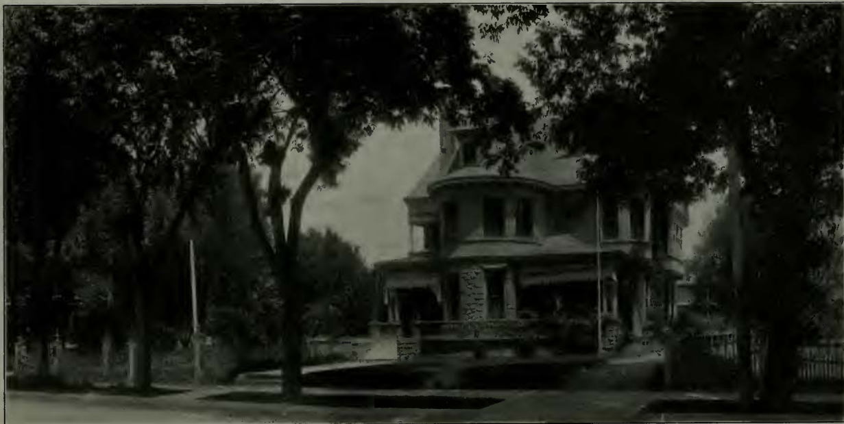
Former Residence of Judge M. E. Hyland, San Jose, Cal. Wolfe & McKenzie, Architects
