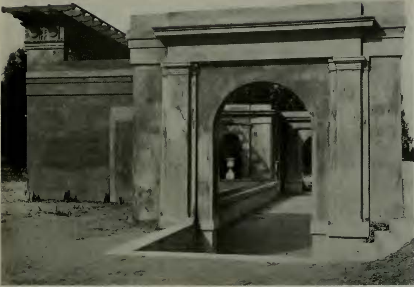
Detail of Entrance, Open Air Theater for Mr. Truxton Beale
