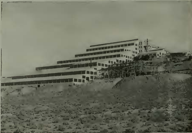
New 100 Stamp Mill of the Goldfield Consolidated Mines Company, Goldfield, Nevada. Entire roofing and siding of ASBESTOS PROTECTED METAL Corrugated Sheets. Duckback Brand
