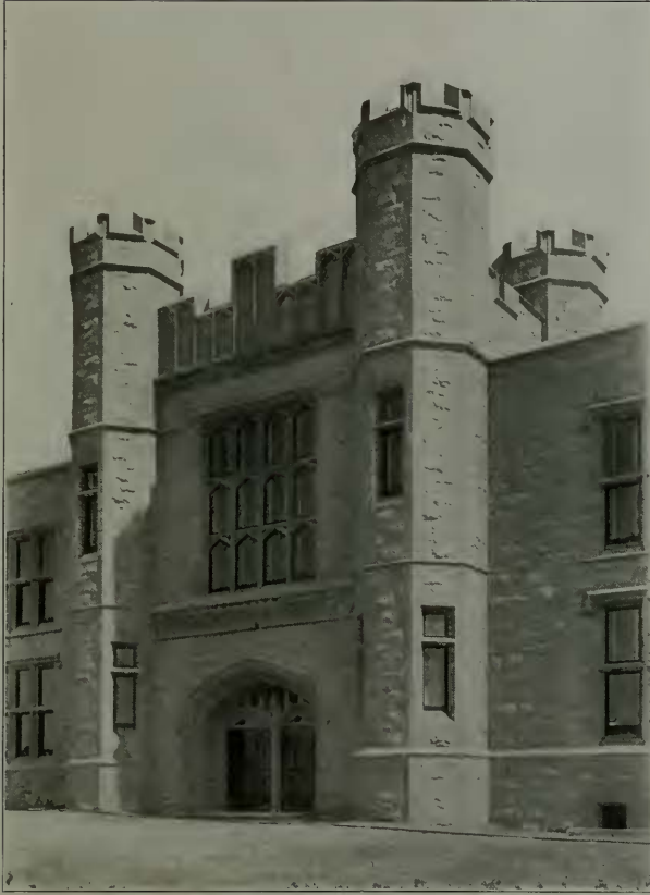
High School, San Diego, West Tower F. S. Allen, Architect
