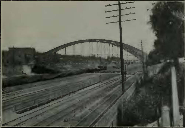
New Type of Bridge in Which the Concrete Floor Is Suspended From the Arch
