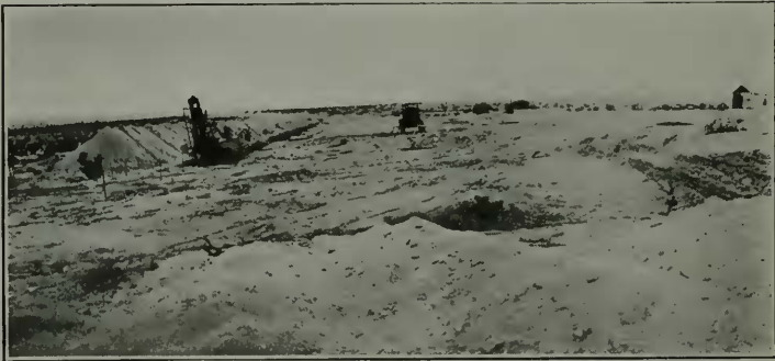
II. Los Angeles Aqueduct—Excavating Aqueduct Channel by Steam Shovel
