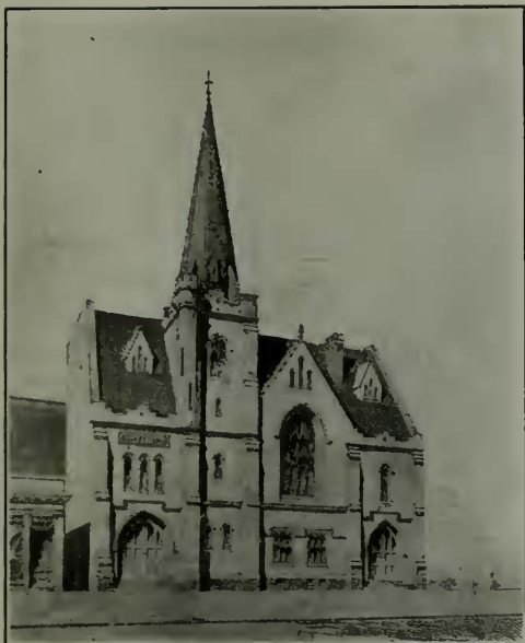
Green Street Congregational Church, San Francisco
