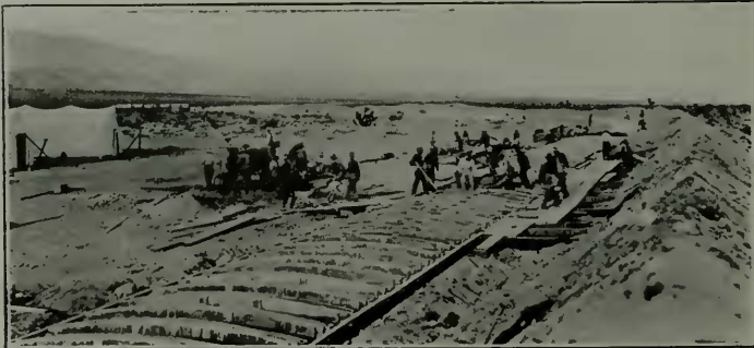
I. Los Angeles Aqueduct—Putting Concrete Cover on Excavated Channel
