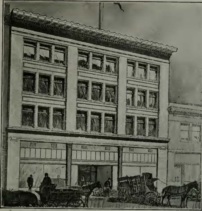
Building for Archbishop Riordan, Mission Street, San Francisco Steel Work by the Brode Iron Works Smith O'Brien, Architect
