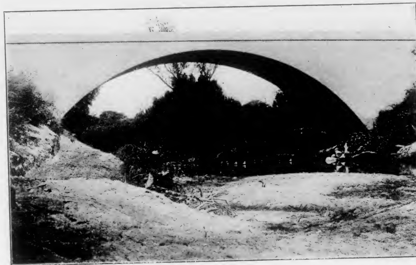
Dry Creek Bridge, Stanislaus County, Cal. Span 112' Ry. 26' Pacific Construction Co., Contractors Jno. B. Leonard, Engineer
