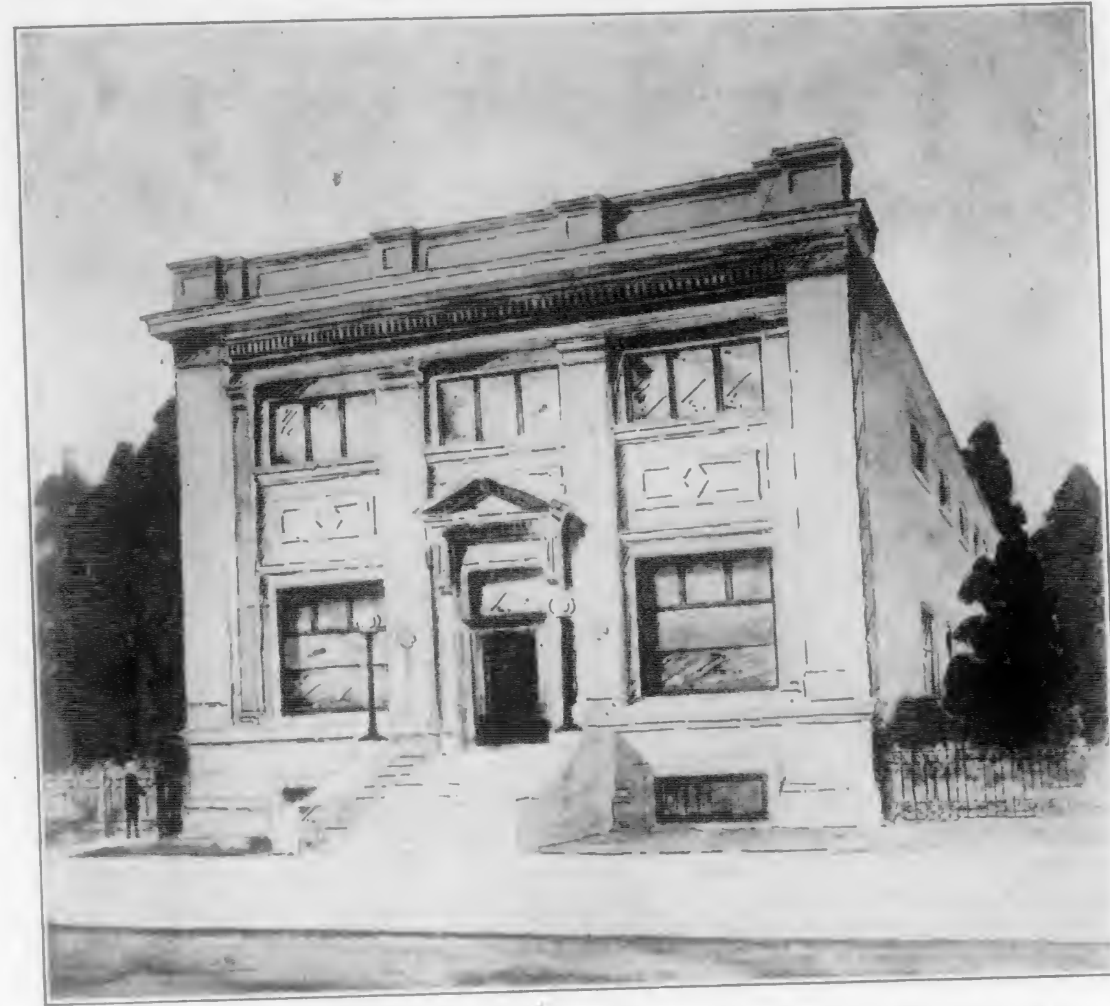
Telephone Building, Oakland
