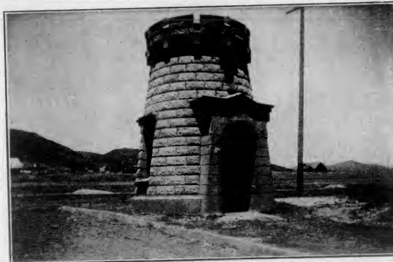
One of Eighteen Towers erected in Hollywood by T. A. McMurtrie from stone made by his latest model machines, capable of adjustment for any size or style of stone.
