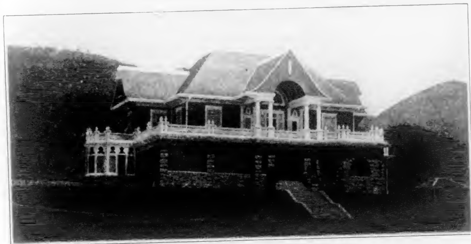
Residence of J. P. Cook, Honolulu
