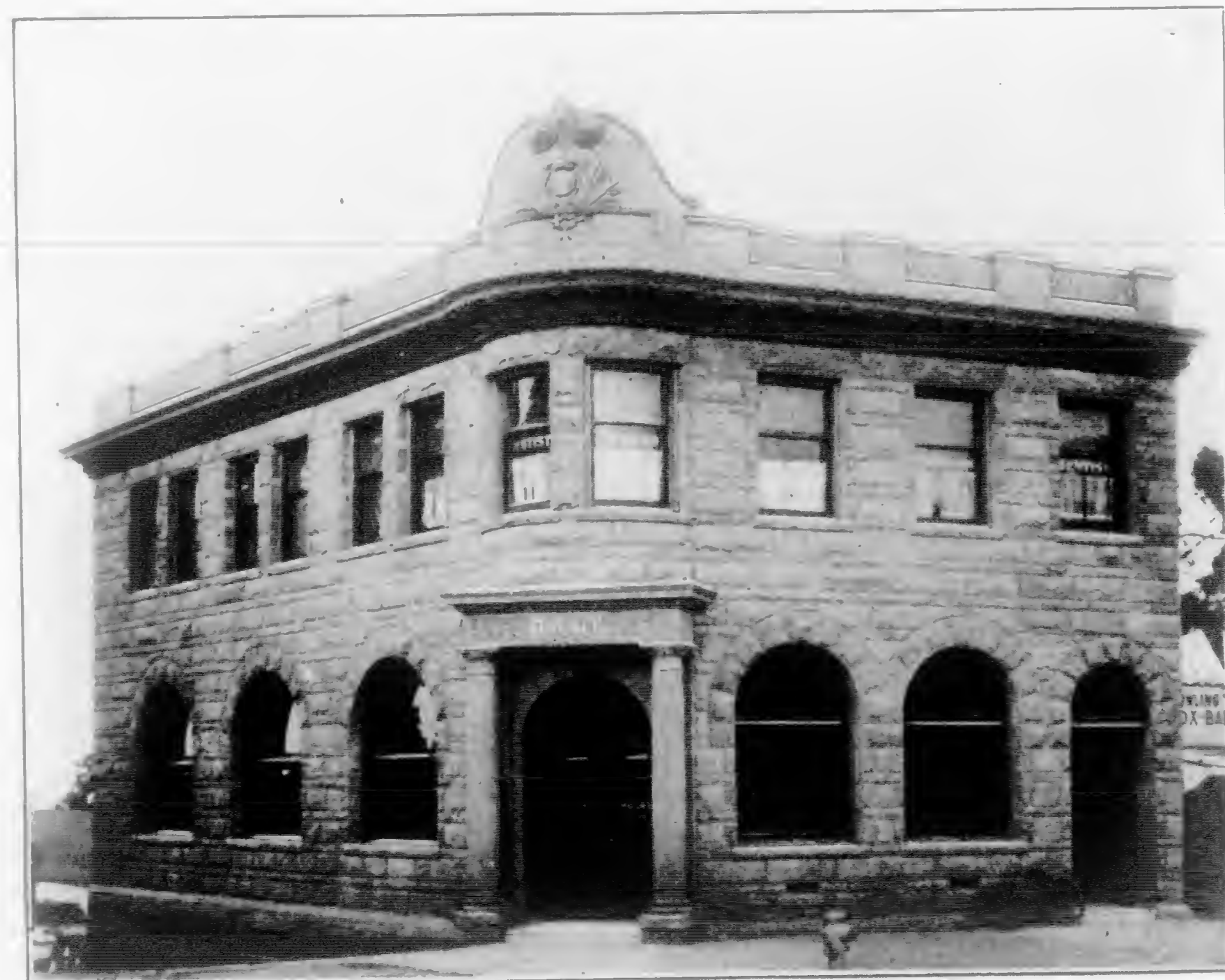
Bank of Pacific Grove, Pacific Grove, Cal. W. H. Weeks, Architect
