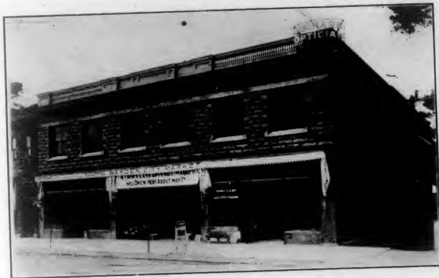
The T. A. Work Building, Pacific Grove, Cal., built of concrete blocks W. H. Weeks, Architect
