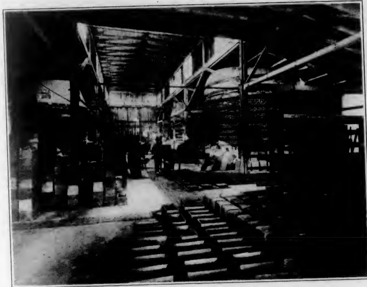
The Kiln Room
