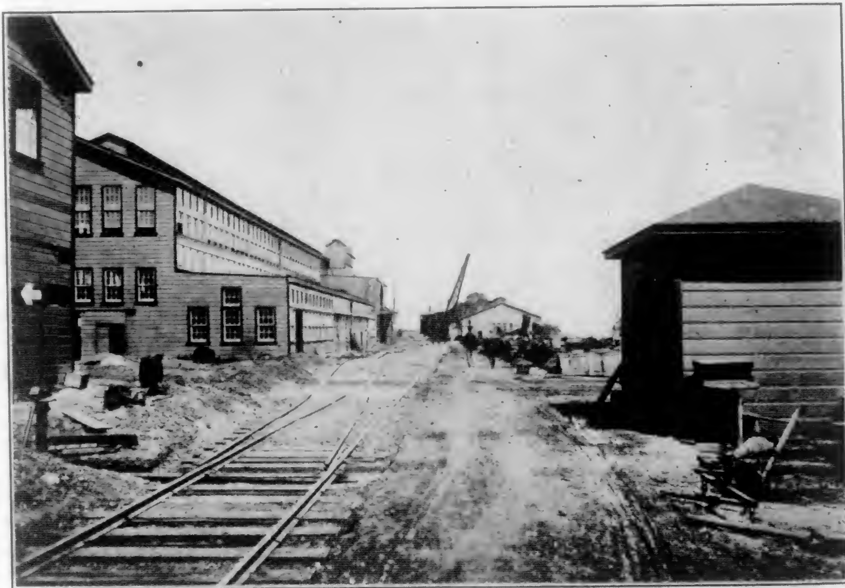
Showing Switching Facilities and Portion of Main Foundry, Joshua Hendy Iron Works, Sunnyvale, Cal.
