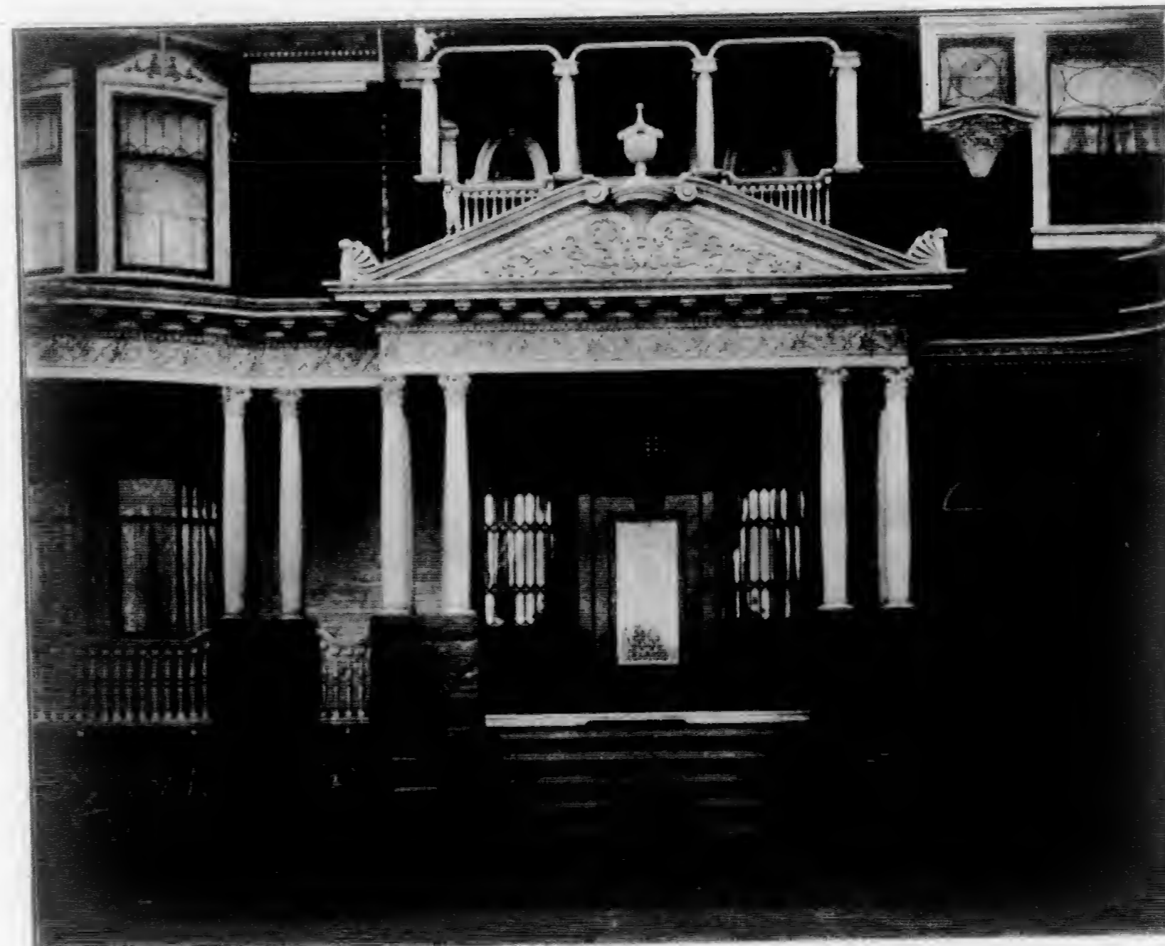
Entrance of Tuttle Residence. Watsonville Cal.
