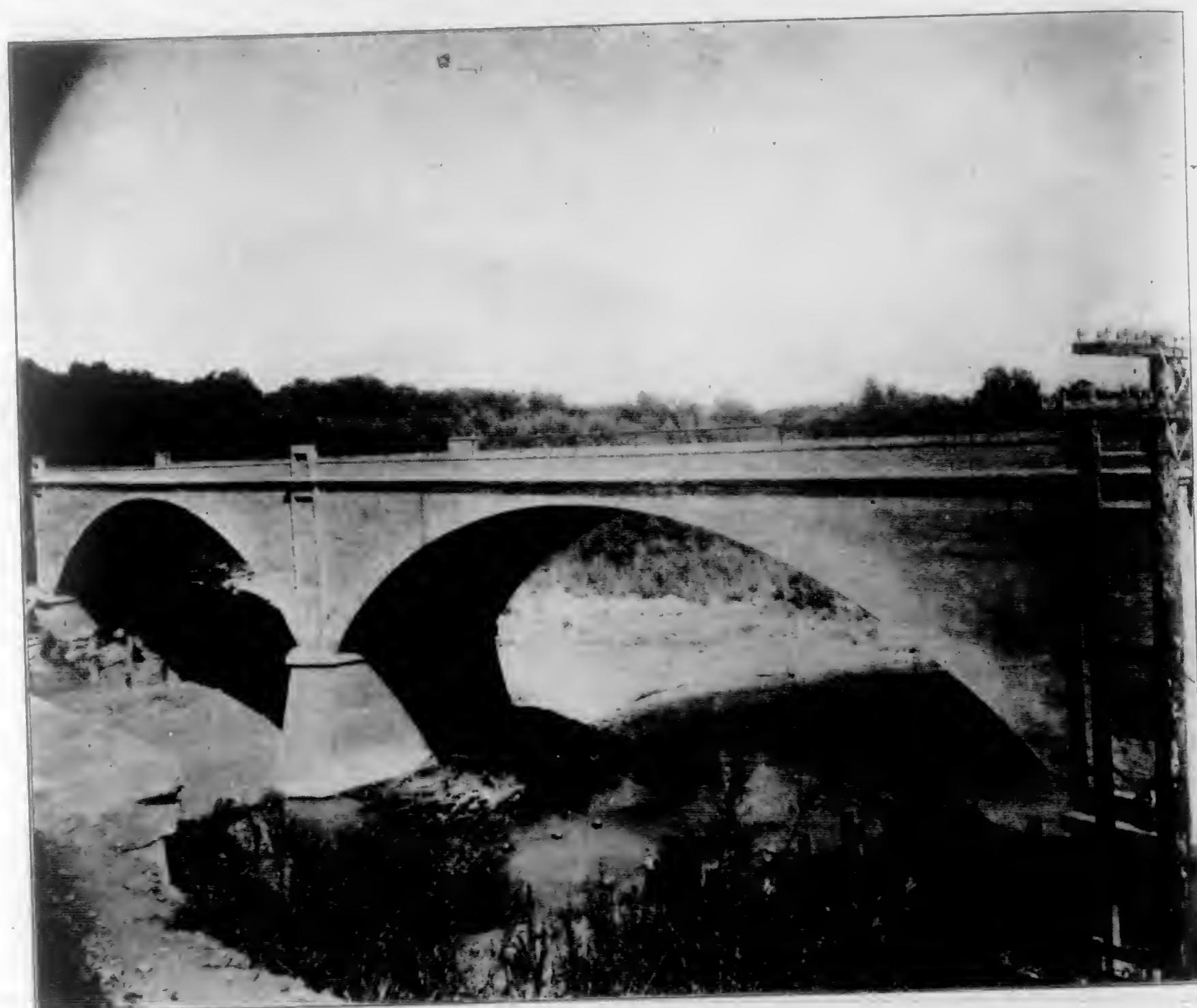
Two One-Hundred Foot Reinforced Concrete Arches, crossing the Stanislaus River, near Rippon, California. Designed by Jno. B. Leonard, C. E.
