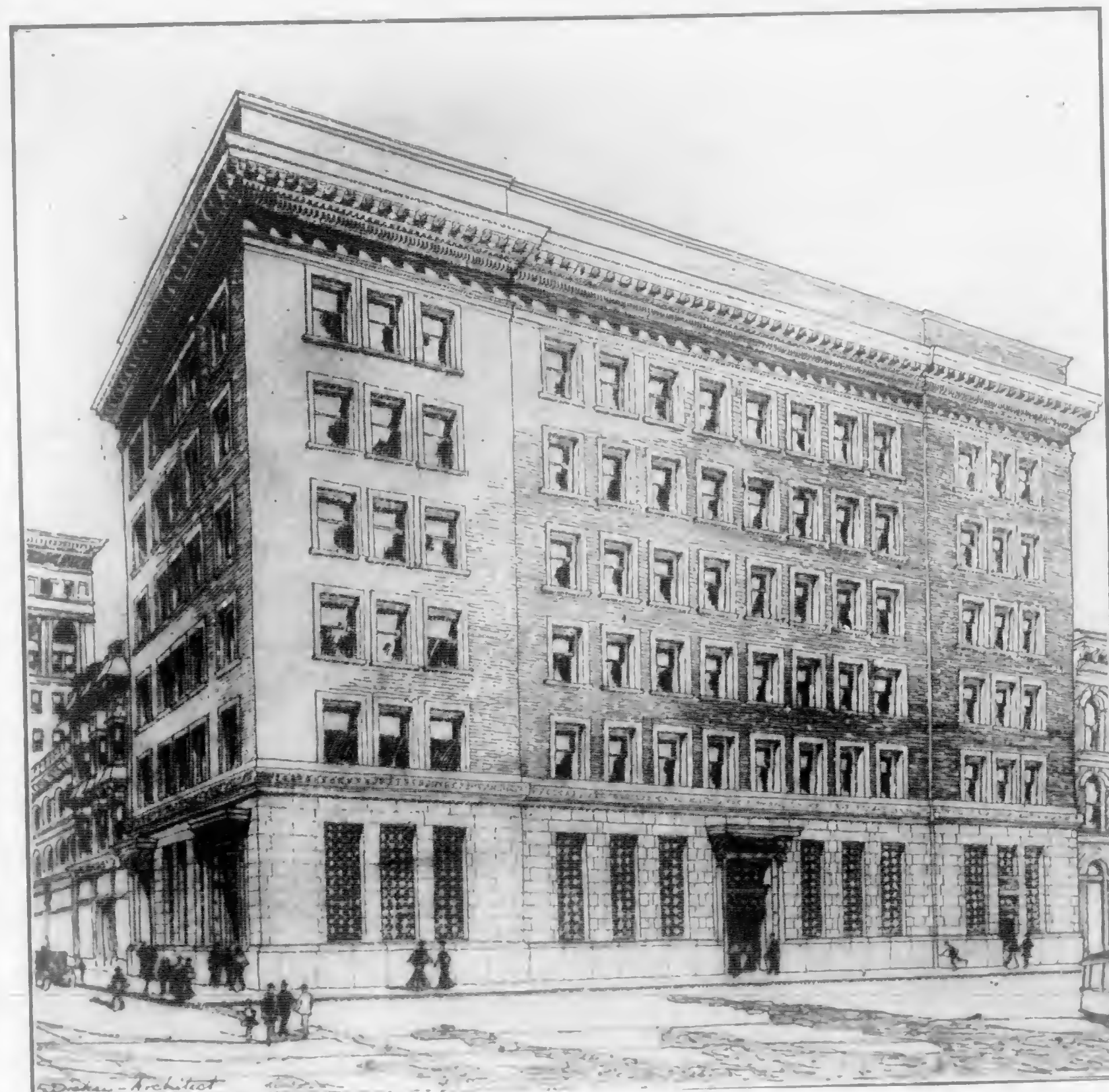
Equipped with Otis Elevators Oakland Bank of Savings Building C. W. Dickey, Architect
