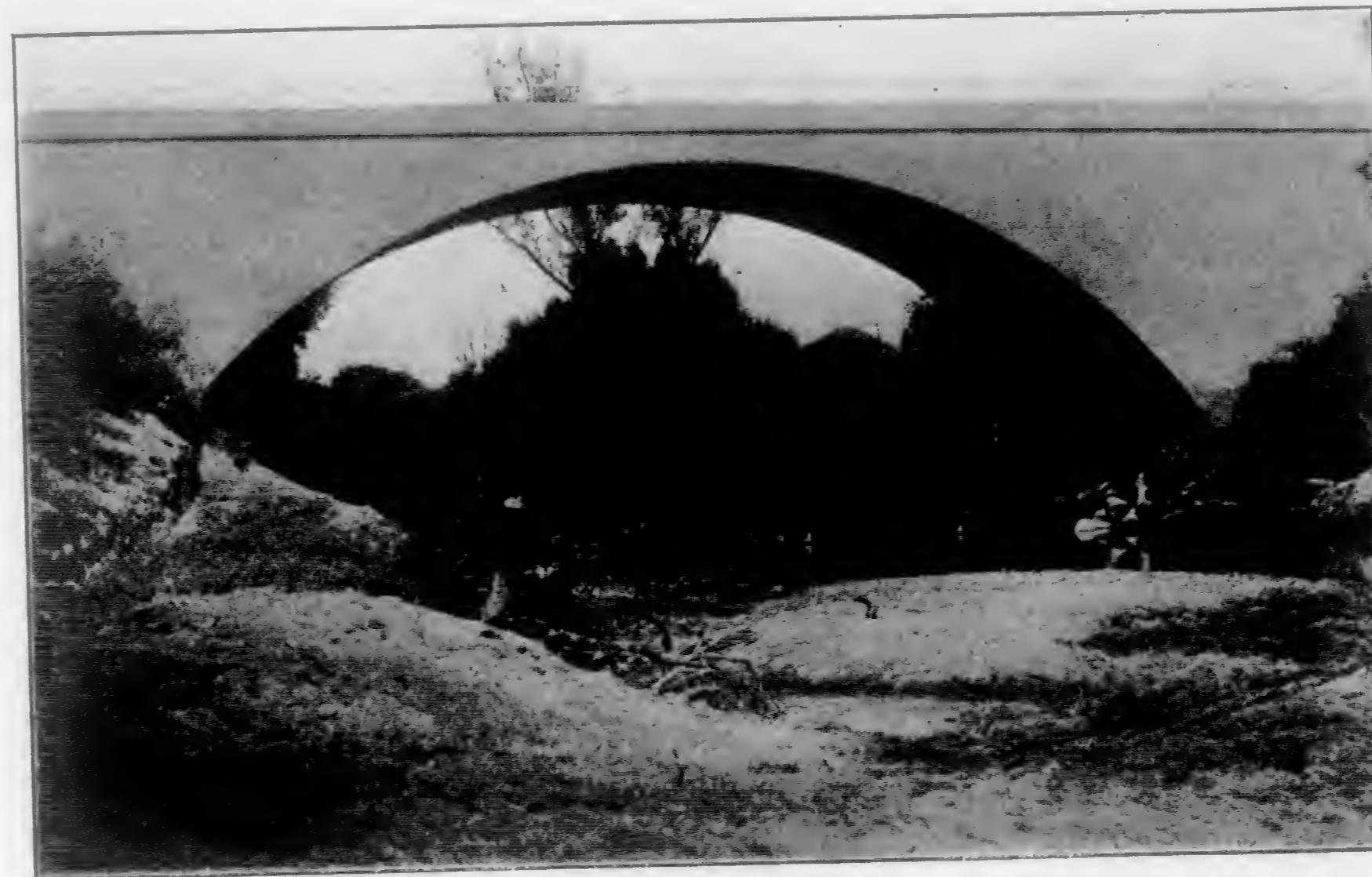
Dry Creek Bridge, Stanislaus County, Cal. Span 112' Ry. 26' Pacific Construction Co., Contractors Jno. B. Leonard, Engineer
