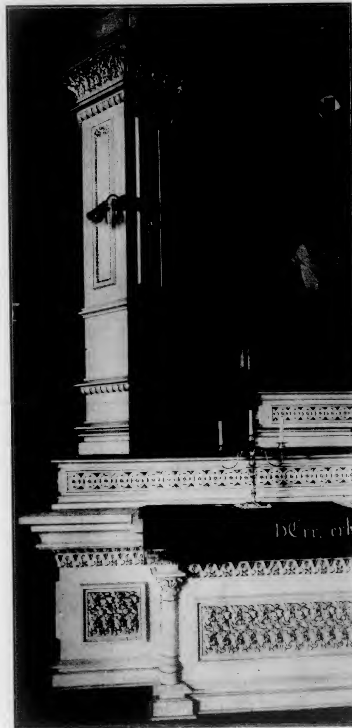
Detail of Interior of Zion Evangelical Lutheran Church, Oakland, Cal. Robert Morgeneier, Architect
