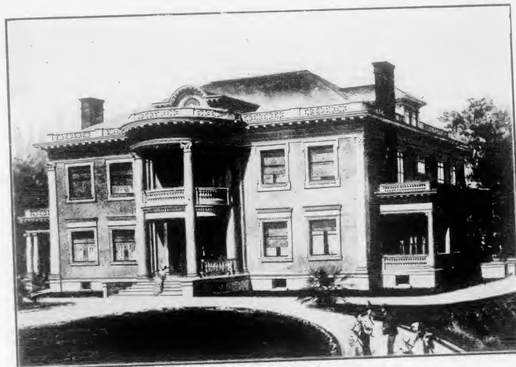
Wash Drawing of House for Mrs. W. P. Dougherty, San Jose, Cal. W. H. Weeks, Architect Mill-work by Santa Clara Valley Mill and Lumber Co.
