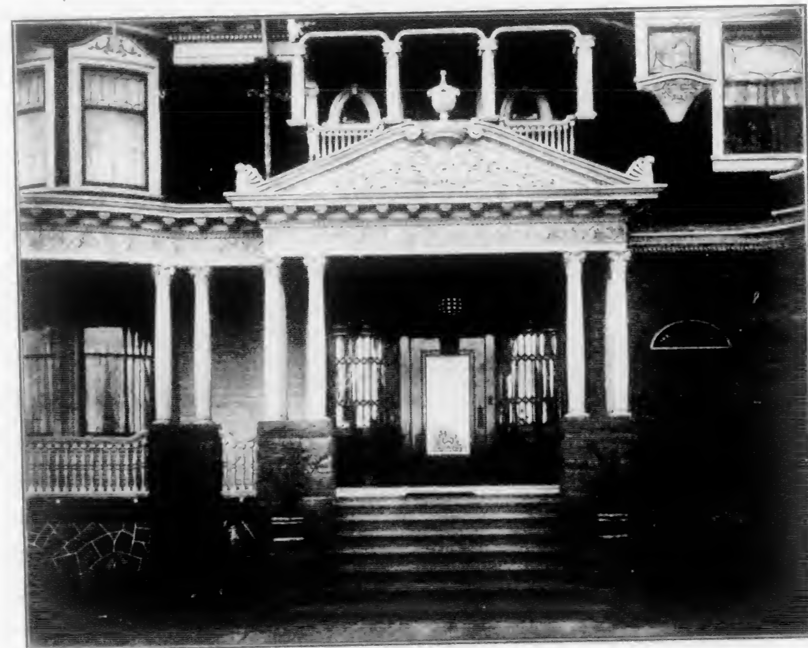
Entrance of Tuttle Residence, Watsonville, Cal.
