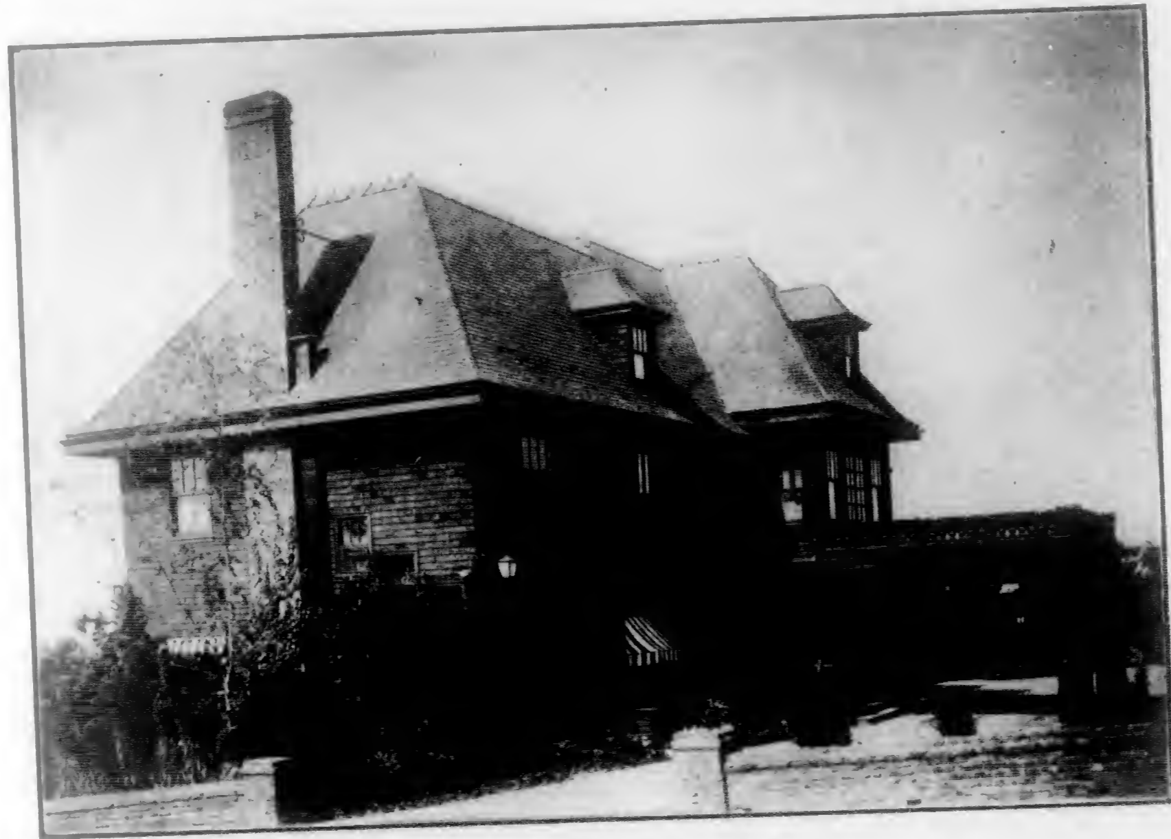
Residence of Wickham Havens, Piedmont C. W. Dickey, Architect
