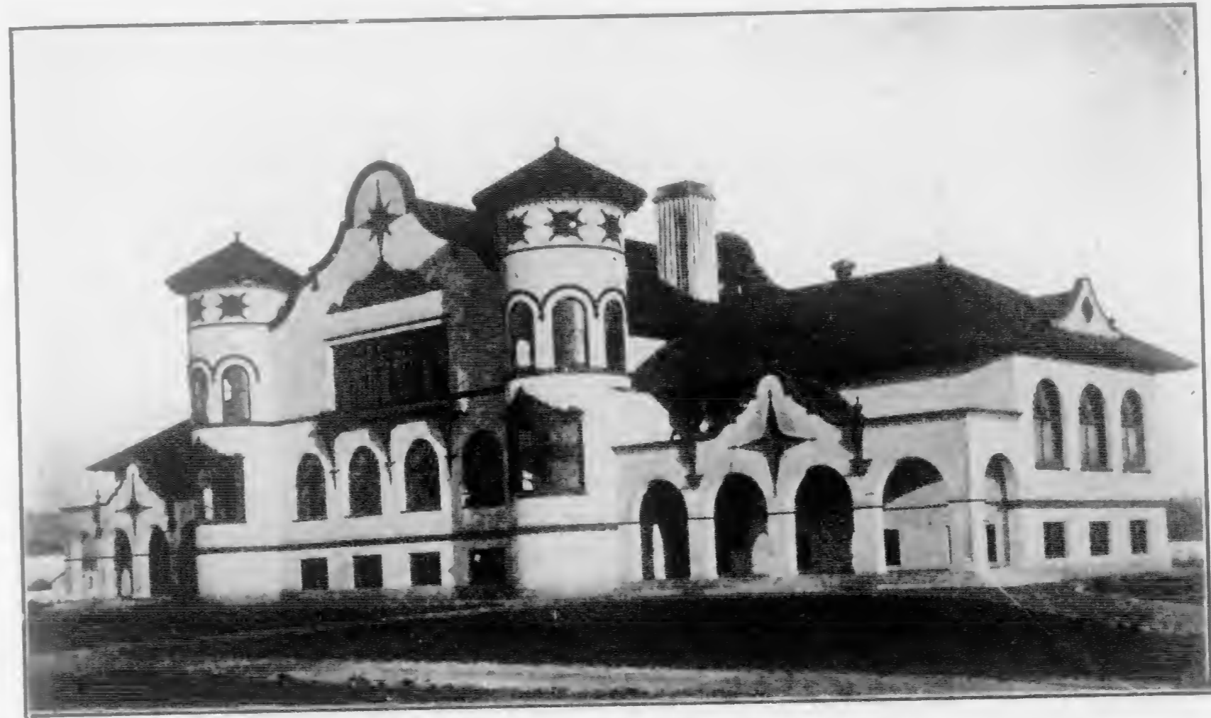
High School, Watsonville, Cal. W. H. Weeks, Architect
