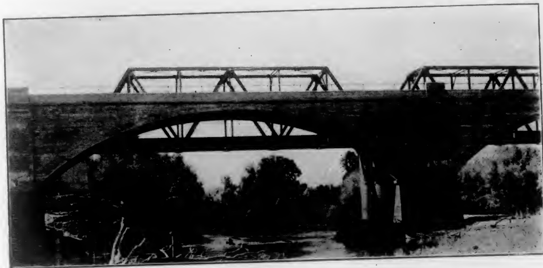
Ripon Bridge between Stanislaus and San Joaquin Counties. Two 100' Spans Pacific Construction Co., Contractors. Jno. B. Leonard, Engineer.
