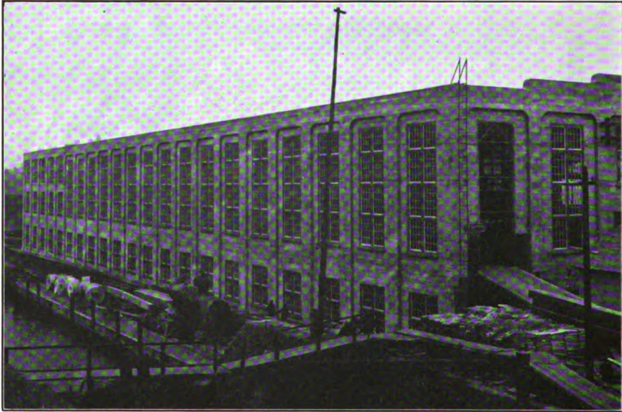
Paper Mill of Reinforced Concrete at Willamette, Or., built by Pacific Construction Co.
