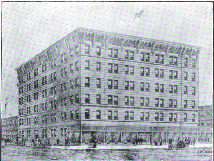
Zellerbach Building Now Under Construction, San Francisco Ross & Burgen, Architects
