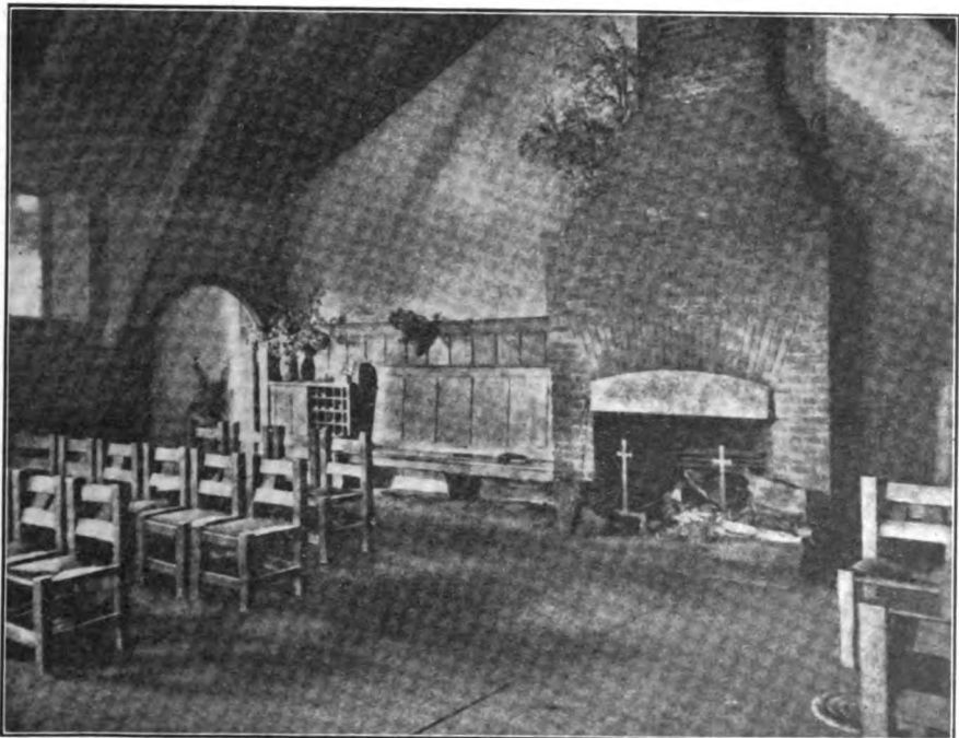
Interior of New Jerusalem Church, San Francisco Page Brown, Architect
