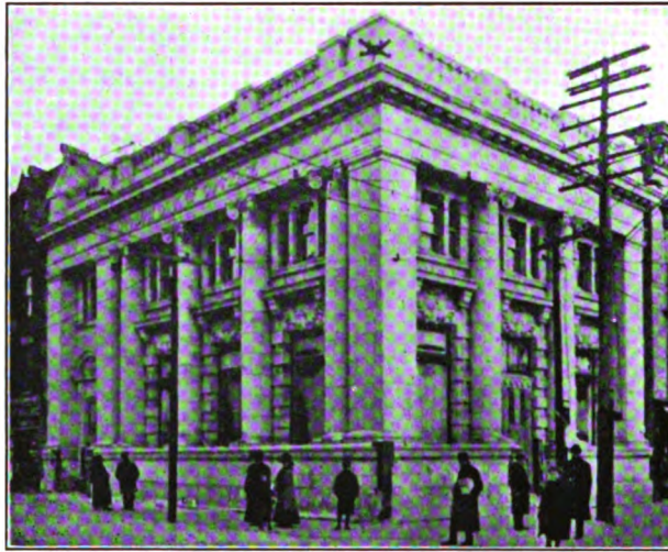
Canadian Bank of Commerce, London, Ontario. Artificial Stone Block Construction
