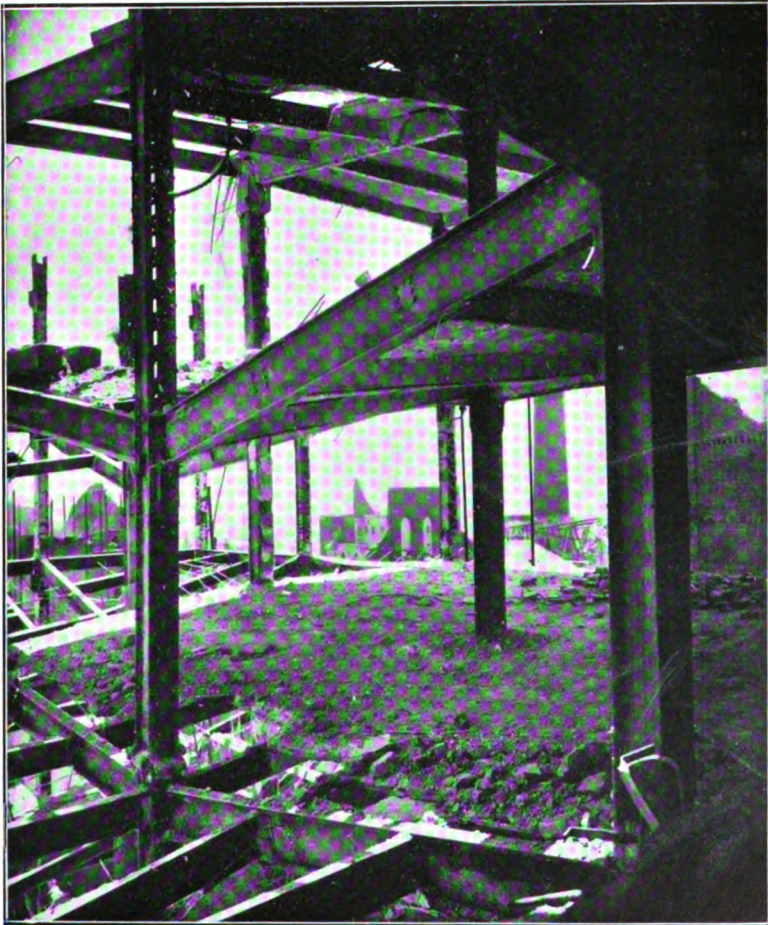
Showing Steel Girders on the Fifth Floor, Kamm Building, San Francisco
