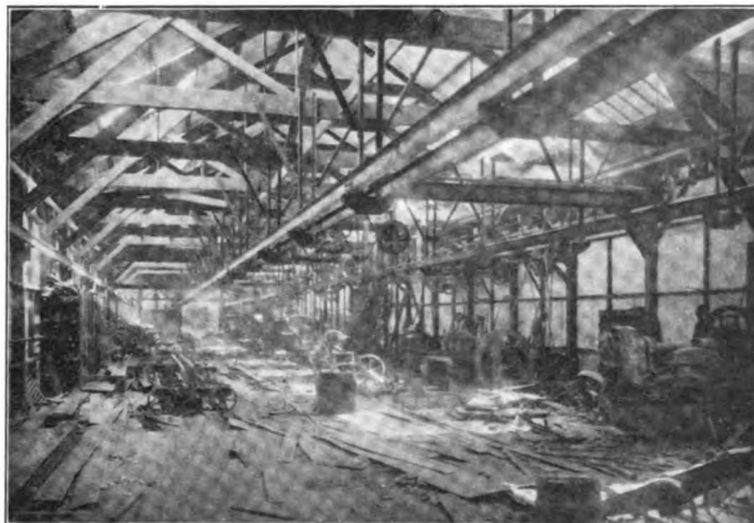
Interior of Western Iron Works Mammoth Machine Shop
