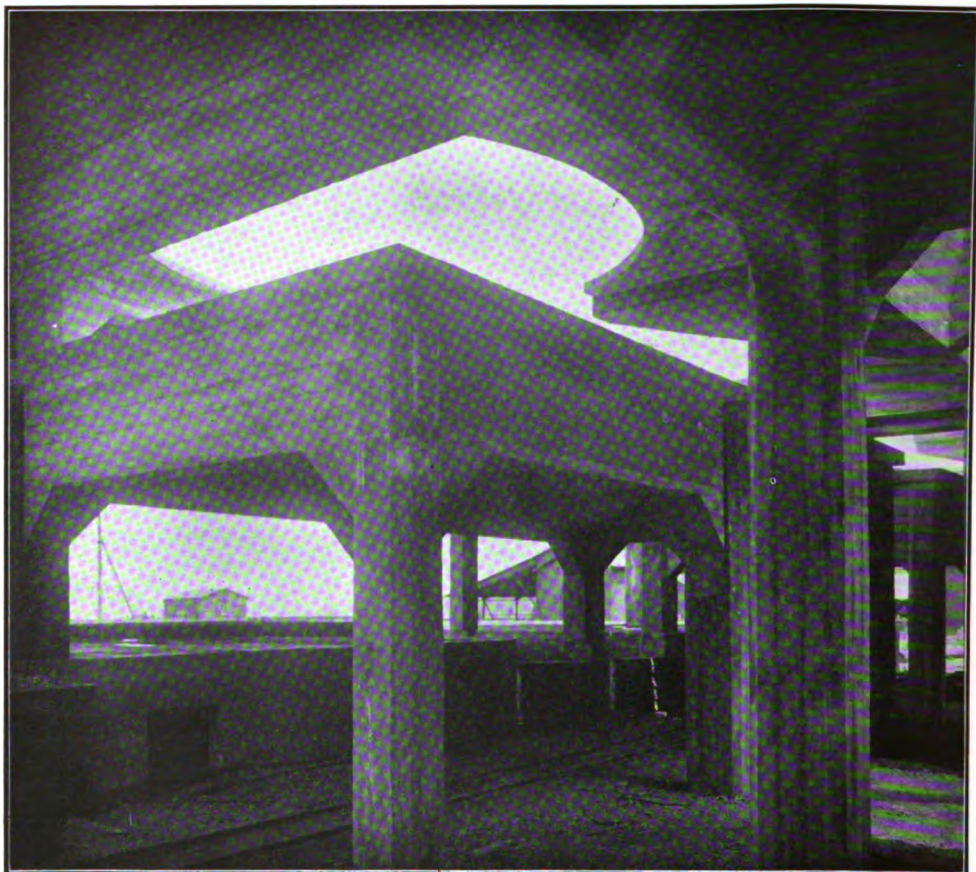
Concrete structure at Selby supporting 60 ton lead ladle reinforced with Corrugated Bars. Lindgren-Hicks, Contractors
