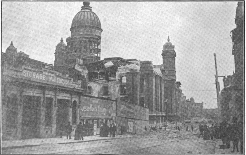
City Hall Before the Fire. An Example of Poor Construction.
