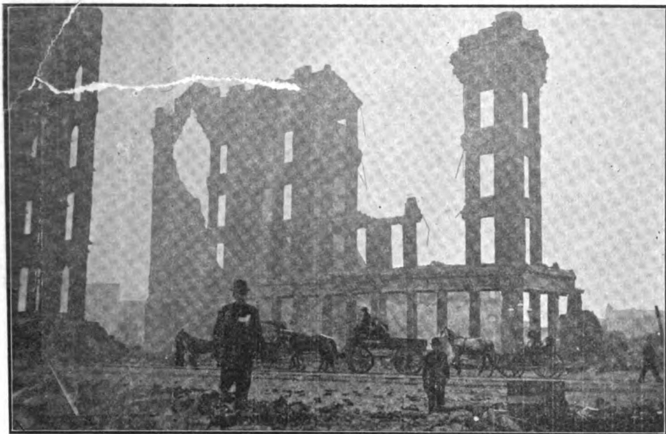
The Baker and Hamilton Building. Typical Example of a Class "B" Building After the Fire.
