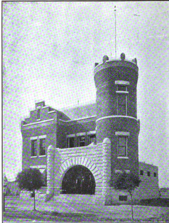
Madera Jail, Built of Brick and Stone Brickwork by F. J. Craycroft & Son
