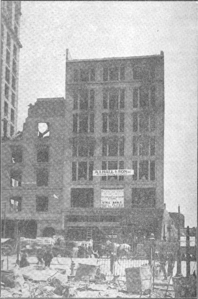
Fig. 3. The Kann Building Having Reinforced Concrete Floors. This was the First Building on Market Street to Be Re-occupied After the Fire
