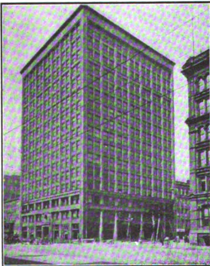
Rockefeller Building, Cleveland, Thompson-Starrett Co. Builders
