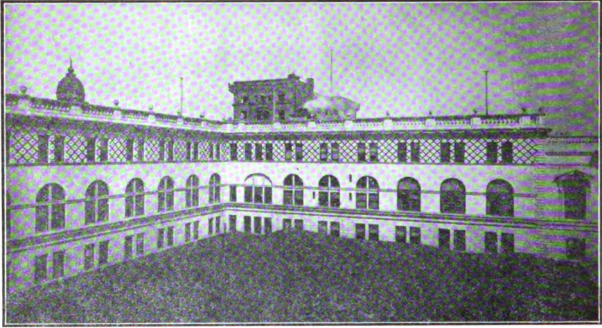
Showing Perfect Condition of Brick Court of Postoffice Building After the Earthquake and Fire
