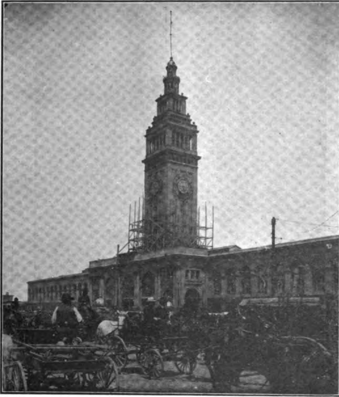
Fig. 8. Ferry Building, the Tower of Which Was Badly Strained by the Temblor and Is Now Being Reconstructed of Reinforced Concrete by the Pacific Construction Company
