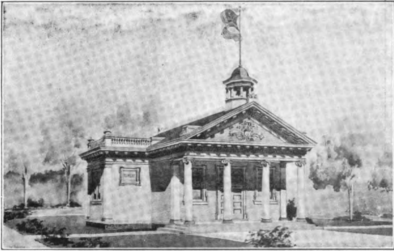
One-Room School in Classic Style—Built of Wood
