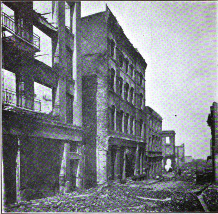
Sub-Treasury Building, San Francisco, Gutted by Fire
