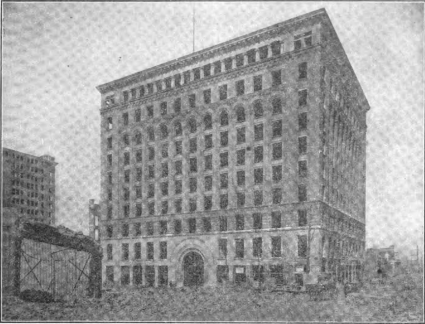
Mills Building. The First and Second stories of Stone Are Badly Damaged. Upper Stories of Brick Not Seriously Damaged — Jean Galen Howard, Architect —
