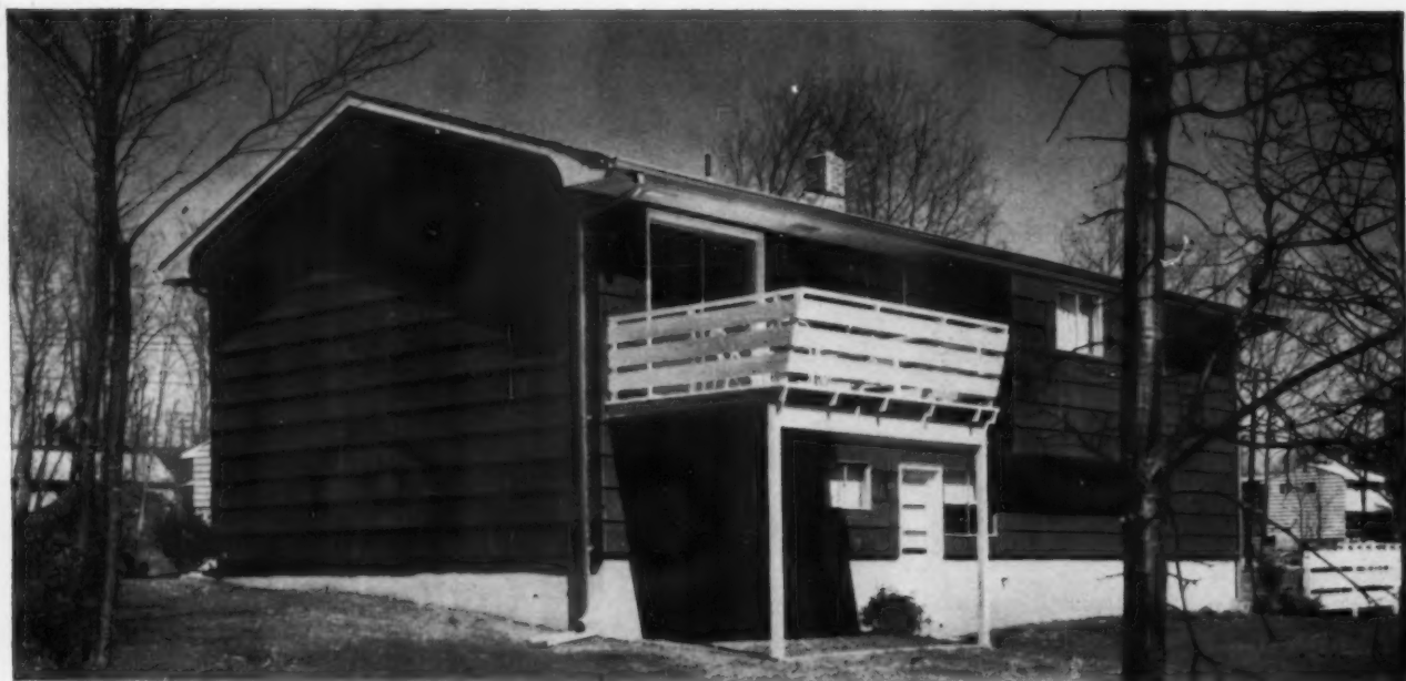
REAR VIEW shows upper sun deck, covered terrace and door leading into large utility room. Bay extends third bedroom.
