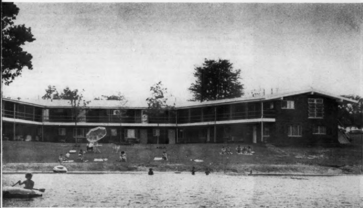
EVERY TENANT HAS A BEACH —Shape of building creates a private beach for all tenants living in apartment house. Sand dredged from lake gives beach ocean-like flair. Builders do not
