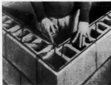
Two engineered products that meet a need. Dur-o-wal reinforcement, shown above, and Rapid Control Joint, below. Weatherproof neoprene flanges on the latter flex with the joint, simplify the caulking problem.
