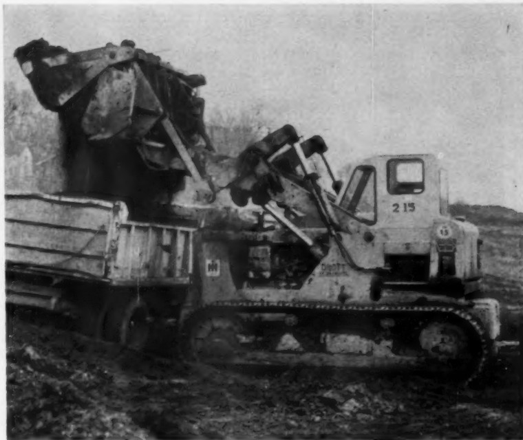
Loader-truck team moves earth speedily and efficiently
