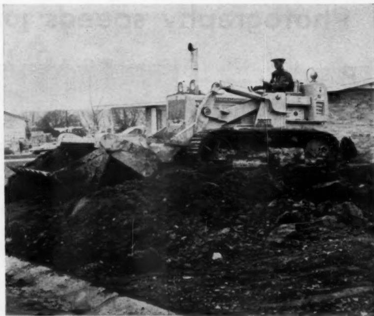
Combination bucket makes four earthmoving machines from one
