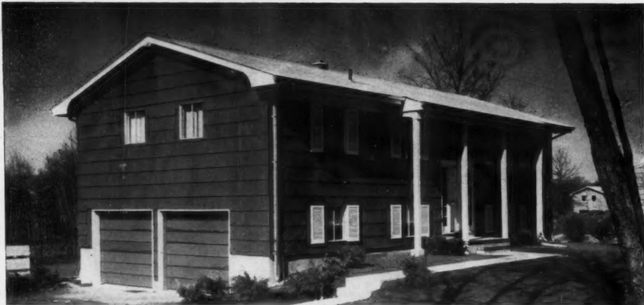
TWO-STORY PORCH adds classic dignity to front elevation; traditional details add nostalgic touch. Lower floor has two-car garage.
