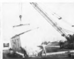
No. 3—8:00 A.M. Section #1 placed
