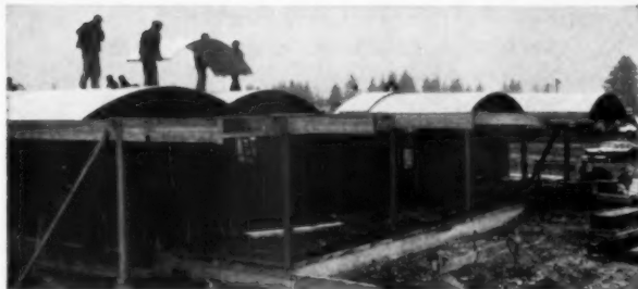
Cutaway shows construction of stressed skin roof panel at left
