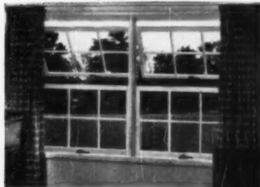
Malta "Town and Country" units, with two fully operating awning-type sash, let in more sun... permit up to 100% ventilation.
