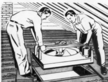
Step 2 Place R&M-Hunter Fan on attic floor or joists over ceiling opening. Easily wired at fan junction box.
