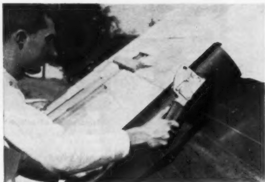
Stapling hammer is more efficient for large areas
