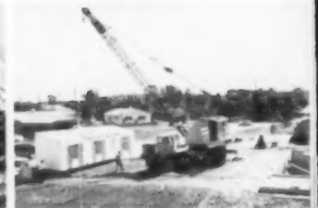
No. 5—9:30 A.M. Section #3 being picked up
