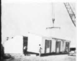
No. 6—10:00 A.M. Section #3 being placed
