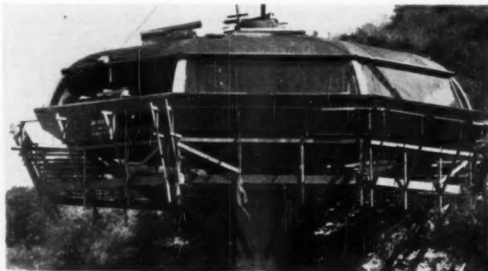
FUTURISTIC octagonal house has large glass areas that give a view of surrounding area. Catwalk is for window washing. Cable car will give access.
