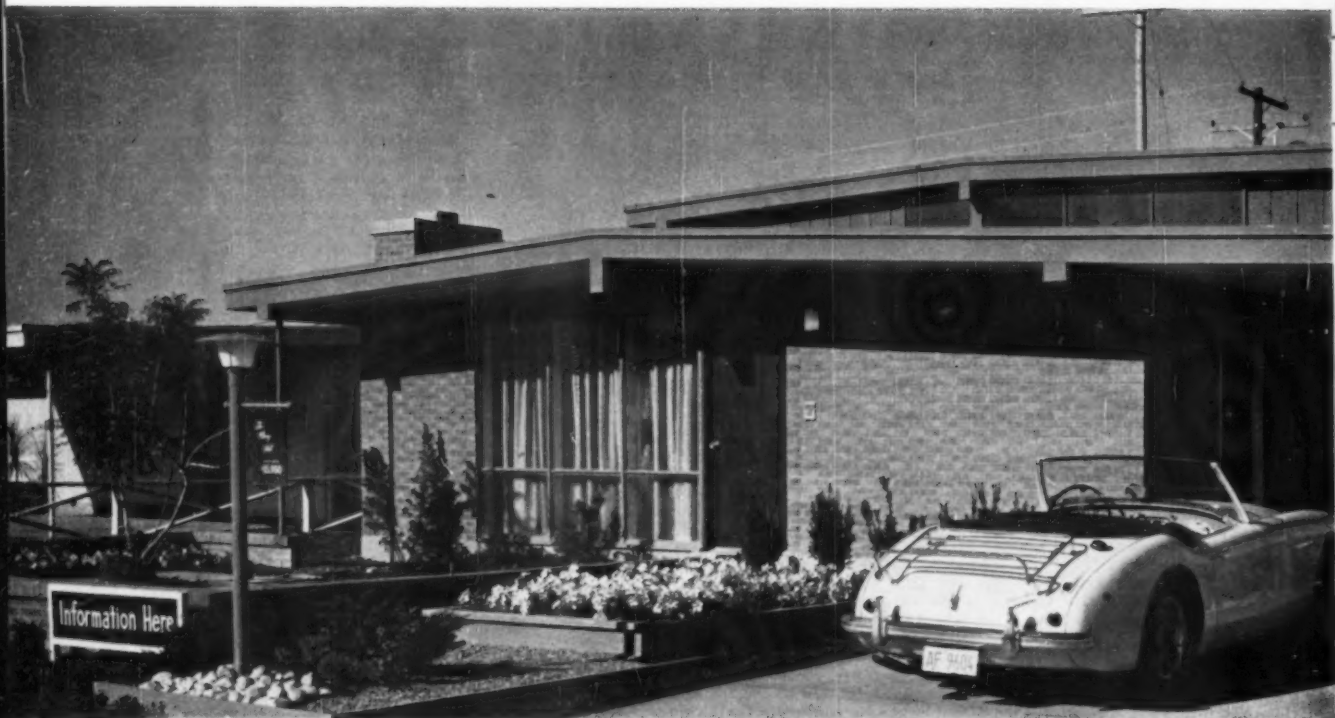
BRICK-WOOD-GLASS combination gives split a custom look. Alternate walk-in basement design is available, with well-
