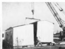
No. 4—8:45 A.M. Section #2 placed
