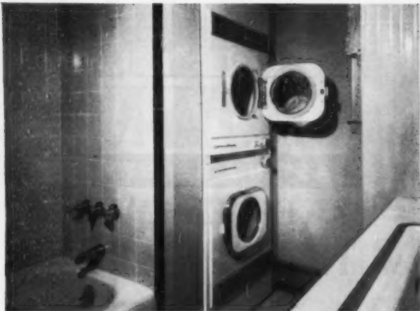
HOUSEWIVES appreciated having the washer and dryer in the bathroom. Stacked as shown, the Westinghouse Space-Mates fit in a space only 25 inches wide. A removable panel in a closet provided access for servicing.
