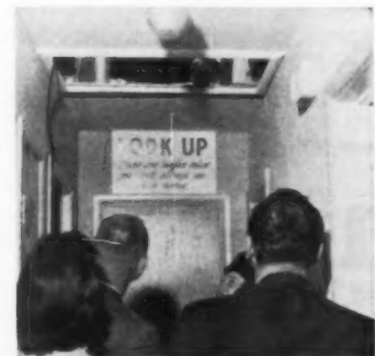
MIRRORS reflect roof, ceiling construction, show type of insulation used.
