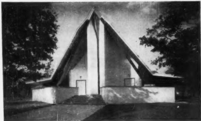
THREE-HINGED ARCH dominates this exterior view of the Grace Church in Massapequa, L.I., N.Y. Laminated members are ideal for such applications, in which they easily support combined roof-sidewall loads.
