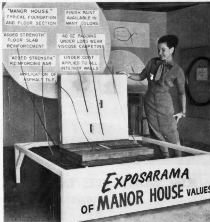
CUTAWAY of foundation, floor and wall section of model home follows scientific theme. All building materials used in construction are keyed to signs.
