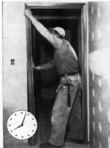
8:03 a.m. Now strike jamb is placed into starting position and rotated to vertical position. Beveled profile of E-Z Frame harmonizes well with contemporary decor.
