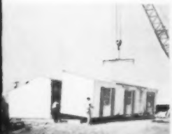
No. 6—10:00 A.M. Section #3 being placed
