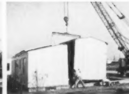
No. 4—8:45 A.M. Section #2 placed
