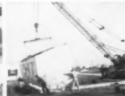
No. 3—8:00 A.M. Section #1 placed
