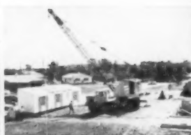
No. 5—9:30 A.M. Section #3 being picked up
