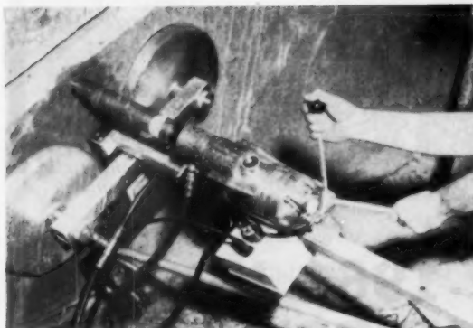
Masonry drill is held by vacuum rig
