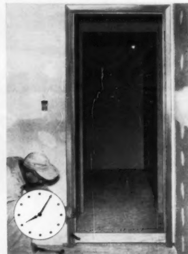
8:05 a.m. Base anchors at bottom of jambs are nailed and the strike plate and rubber bumpers installed. No nail holes to fill . . . anchors covered by base molding.
