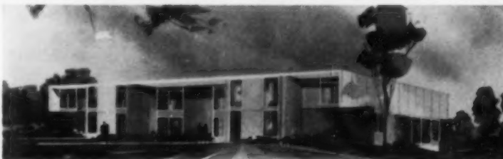
TWO-STORY UNITS of brick, and "Glasweld," have ample fenestration.
