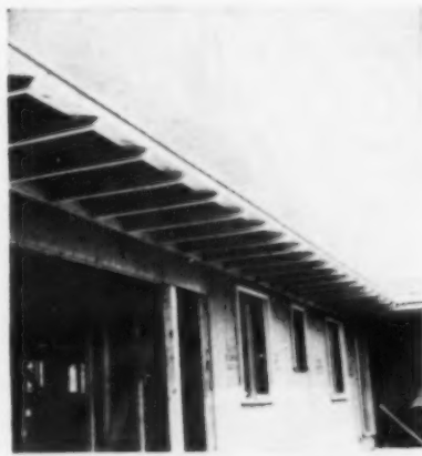
COMPLETED GUTTER installed ready for redwood fascia board to be nailed in place (it will be nailed in usual manner), with fascia in place, gutter is hidden, roof appearance is improved.
