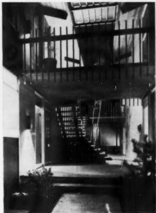
INTIMATE SCALE , for which the project was cited by the AIA, is apparent in the entry stairs. Translucent stairwell roof, shoji entrance doors, rail detailing put a luxury stamp on each unit (see details below).
