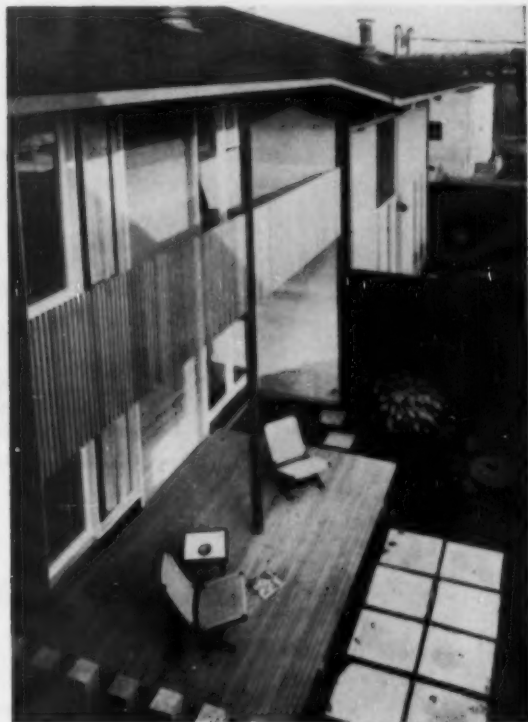
FIRST-FLOOR SUN DECK is laminated 2x4s on edge with \frac{1}{8} " spacing. Entire deck is raised, supported by concrete pedestals. Fence rails and bamboo blinds on second level add to over-all textural effectiveness.
