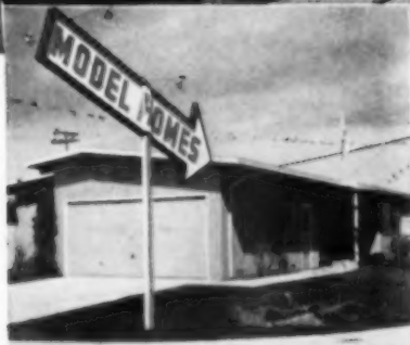
Richard Grant used Texture One-Eleven® combined siding-sheathing, saved 18 man hours on wall construction, plus materials.
