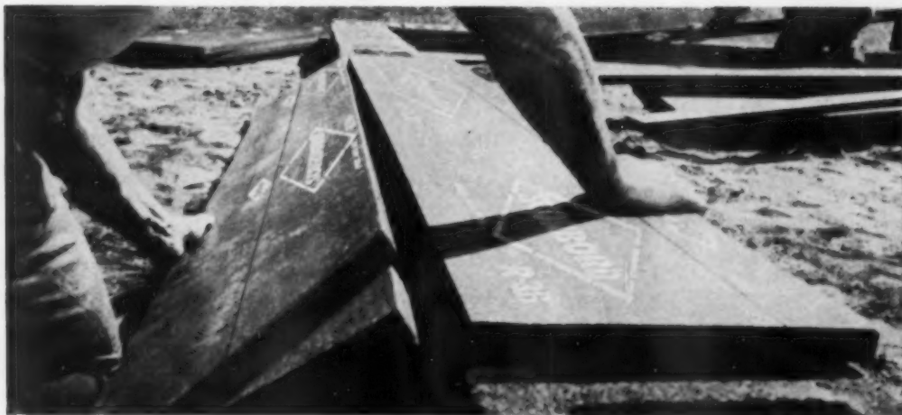
Scorbord snaps off at convenient pre-scored intervals, saves installation time and labor.
