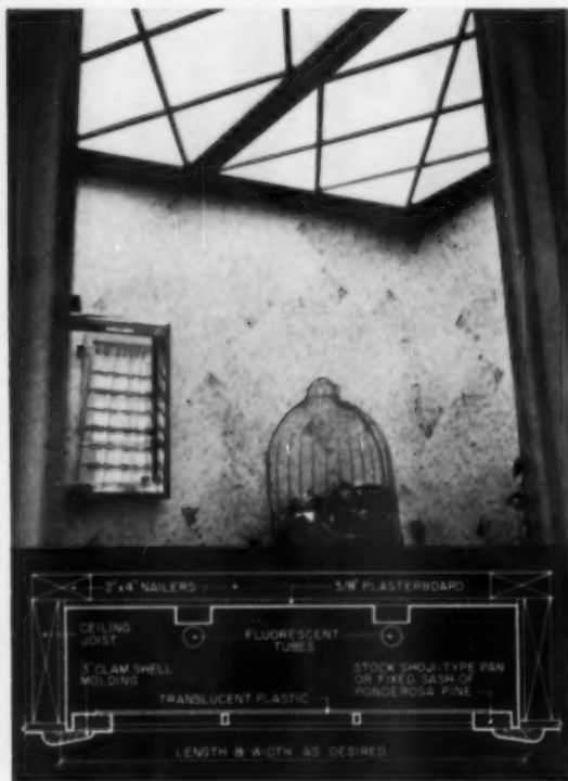
POWDER ROOM ceiling has translucent glass panels covering recessed fluorescent lighting. Frames and diagonal muntins are of ponderosa pine.
