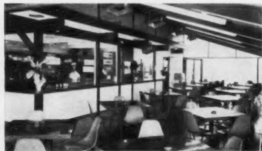
PLACEMENT inside the restaurant. Units are over the service windows and the eating area. Dining "patio" is half closed, has steel-framed glass panels on wheels at each end to close against wind or cold.
