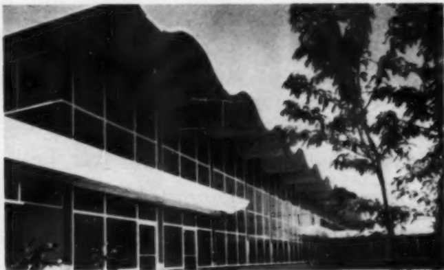
THE CONTOUR-FOLLOWING SPRAYED ASBESTOS provides soundproofing and insulation, in an attractive, fireproof finish.
