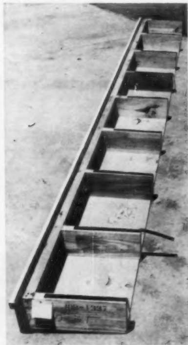
BASIC GABLE RAKE design. Four rakes like these can be installed by four men in 30 minutes. Steel straps fasten the as-
