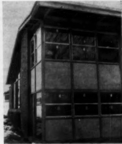
BACK VIEW shows attractive result of adapting curtain-wall method to this house.
