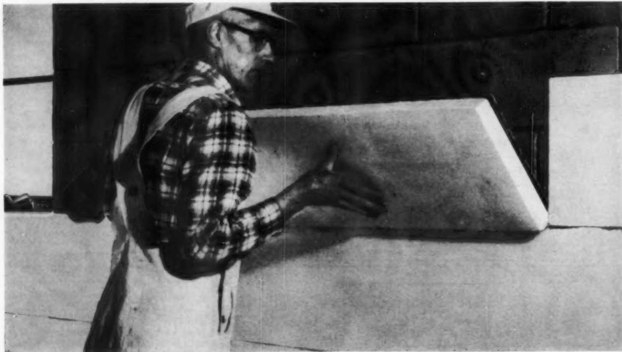
Styrofoam can be bonded directly to masonry walls, eliminating furring and lathing.
