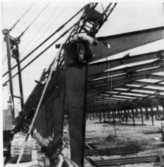
RIGID FRAME —Inland Steel's rigid frame building comes in clear-span widths up to 120 ft. Clear span gives low, spacious appearance to building. Other Inland designs: arch type, post and beam, and slope-beam buildings.
