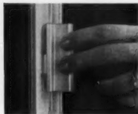
3. Pawler-proof latch with positive locking pin design.
