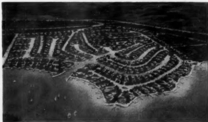
BY 1964: Venice-in-Seattle. Some 200 acres of marshland is under development on Lake Washington. Result will be 350 home sites on the lake or on 20,000 ft. of canal frontage. Development is 15 min. from Seattle.
