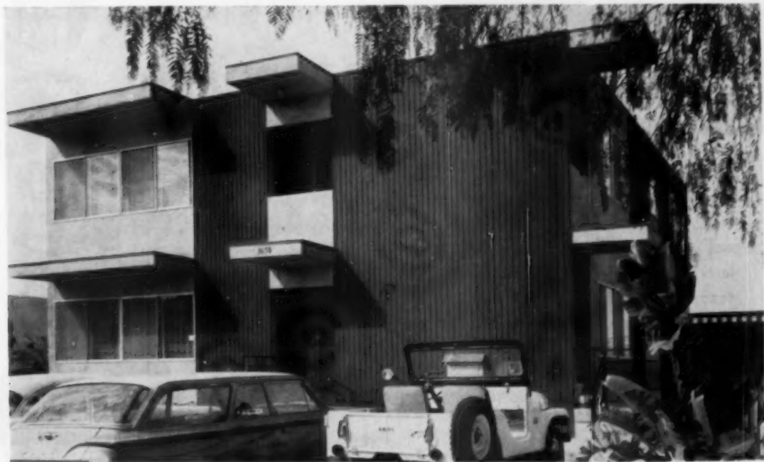
Unit B, above, is placed at front of lot in side of hill; has three floors; contains three 2-bedroom and two
