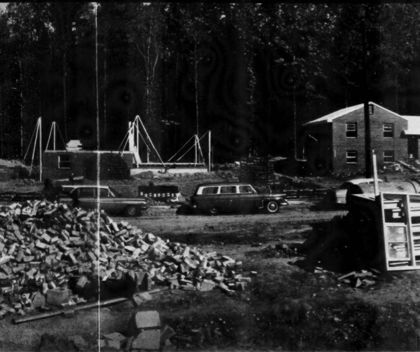
of the largest project converted to the new "SCR masonry process." Dominant feature is the corner pole or coursing scale. Thanks to the new system, builder
