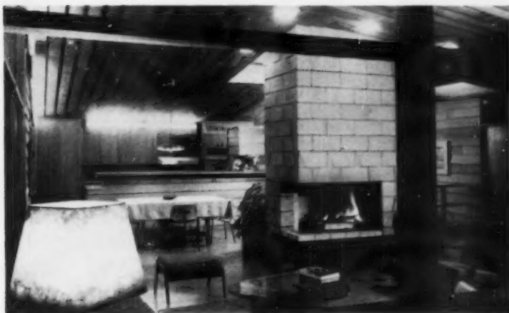
FIREPLACE CORE —Sculptured Shadowal concrete block make up fireplace core through both levels.
