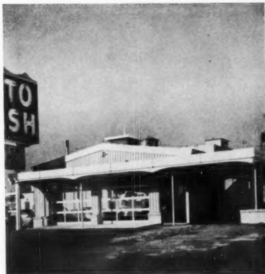
SMALL BUILDING —Stran-Steel's Stran-Master serves as the core of this 32x102-ft. Auto Wash in Robbinsdale, Minn. The building is completely insulated. Progress drawings (right) show rapid step by step of erection.
