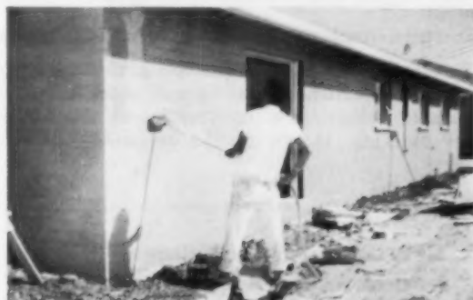
"Hose-fed roller applies outside paint"
