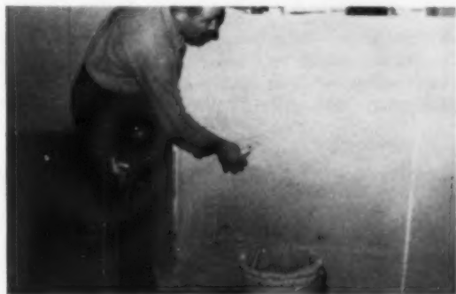
"Gypsum board applied with mastic"
