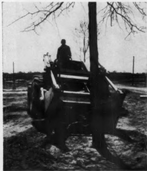
MACHINE UPROOTS TREE —Large bucket blade of Michigan tractor cuts the earth on either side of the tree.
