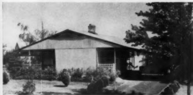
BEFORE —Typical 1,000-sq.-ft. ranch built by Levitt in 1954. It sold for $10,000. It boasted two bedrooms, had a sliding wall permitting den to convert to third bedroom. Fireplace separates dining and living areas.
