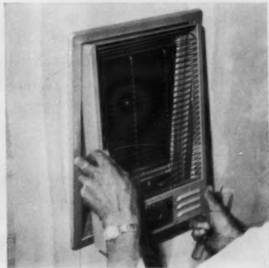
Inner frame consists of two buss bars with multiple carbon contacts fastened to stainless steel springs that provide electrical contact. Generally, frame is steel, has built-in heat deflector. Controls can be built in, too.
