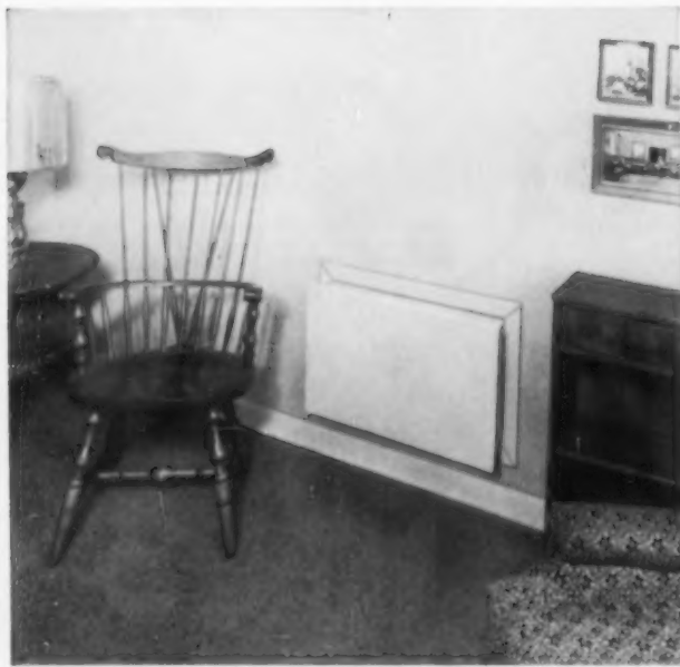
In the living room of a model home, the baffle of the Built-In Thinline Air Conditioner is painted to match the walls.
