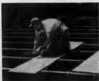
FORMING —K-Clip, (cast iron) fits to upper flange of joist, provides seat for forms. Breaking it releases form.
