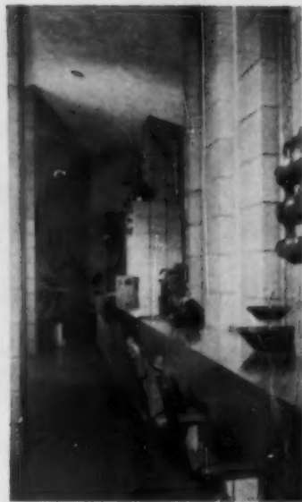
SLOTS 16" wide, with jalousies or fixed glass, alternate with 16" concrete blocks. Narrow counter provides kitchen eating space.
