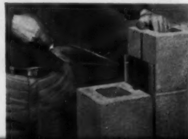
Two engineered products that meet a need. Dur-o-wal reinforcement, shown above, and Rapid Control Joint, below. Weatherproof neoprene flanges on the latter flex with the joint, simplify the caulking problem.
