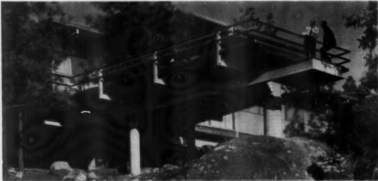
DECK IS SUPPORTED BY frame of 16 WF 36 beams. Frame extends 40 ft. out from house, rests on concrete pylons.
