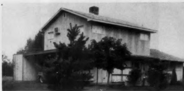
AFTER —2nd story addition is built on top of 1-story ranch house (see drawings below). Addition includes: two bedrooms; ceramic tile bath; new stairway; radiant hot-water heat. Total cost of the new work: $4,700.
