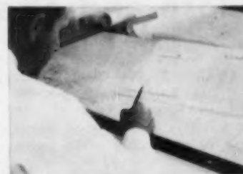
12. Plans are drawn; architect applies for building permit.
