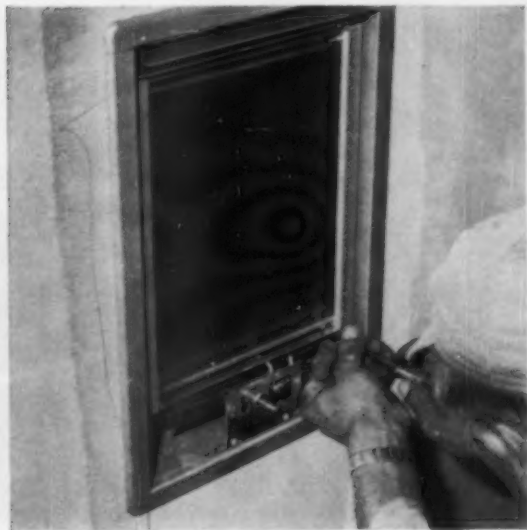
RADIANT HEATERS —Surface-mounted heater proves ideal for laundry, bathroom, ticket offices, other small rooms. No recessing is required for simple installation. These heaters usually supplement existing heating systems.
