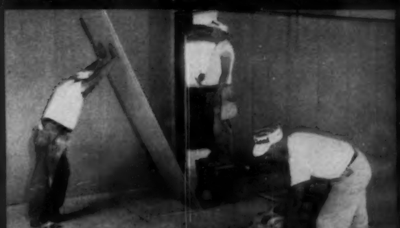
3. 1" core of laminated long-length gypsum lath erected
