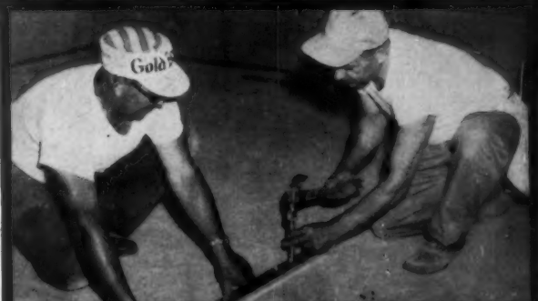
1. 2" channel is nailed in position
