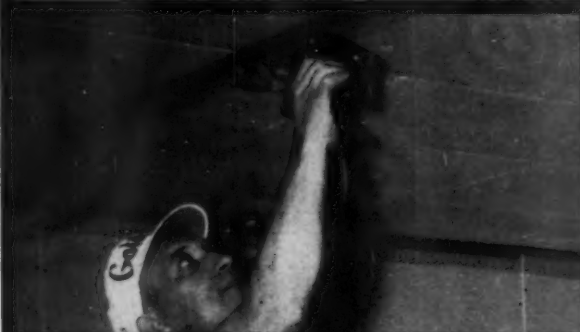
2. Safe-Edge® Cornerite stapled to ceiling
