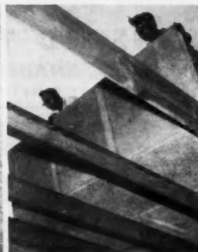
High insulating Cemex panels sheath roof quickly and acoustical ceiling is "free."
