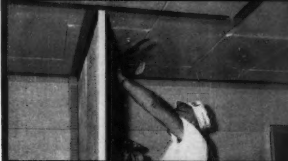
4. Safe-Edge® Cornerite stapled to other side
