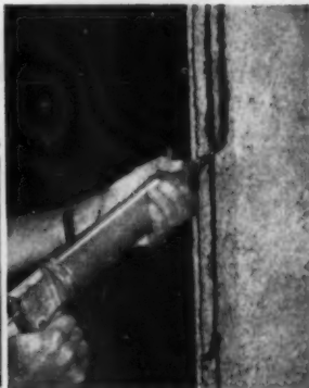
Double bead of Miracle mastic gives joint that is stronger than the Cemex itself.
