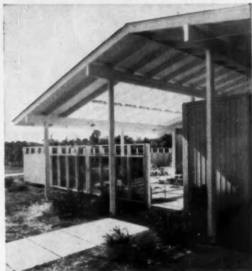
PLANTS on near side of walk are a Spreading Cotton-caster, a Weeping Evergreen Privet, and a Gold Dust Plant. Shrubs beyond walk are Evergreen Privets.
