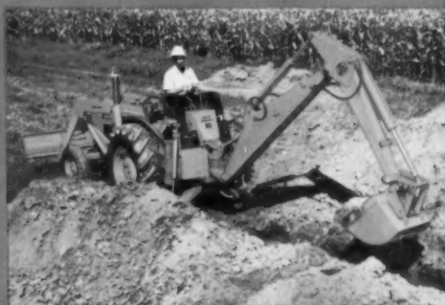
Working depth of the 50 Backhoe is 13 feet 6 inches.
