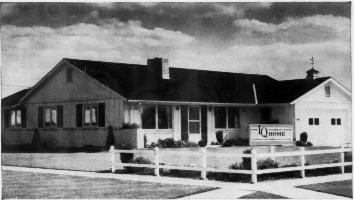
Bob Schmitt of Bob Schmitt Homes, Berea, Ohio, uses Curtis windows to vary proportions of masses and styling with one basic plan.
