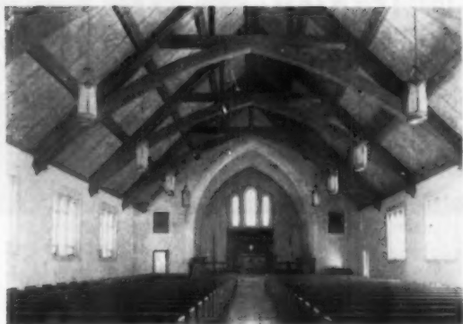
CEMEX installation in St. Olaf's Lutheran Church, Fort Dodge, Iowa. Architect, Frank W. Griffith; contractor, Glenn Walker & Co. Slabs were left exposed to take advantage of their decorative and acoustical qualities.
