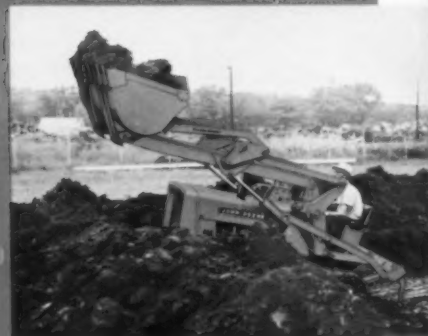
Self-leveling bucket has a full-height dumping angle of 50 degrees.
