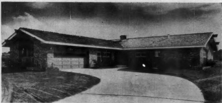
23 LOOK OF THE RUGGED RANCH is achieved in this model through use of cedar roof shingles, board-and-batten touches, and extended roof beams at the gable ends. McCune Homes, Inc., of Tulsa, Okla., are the builders. Price of the house is $24,800 without land.
