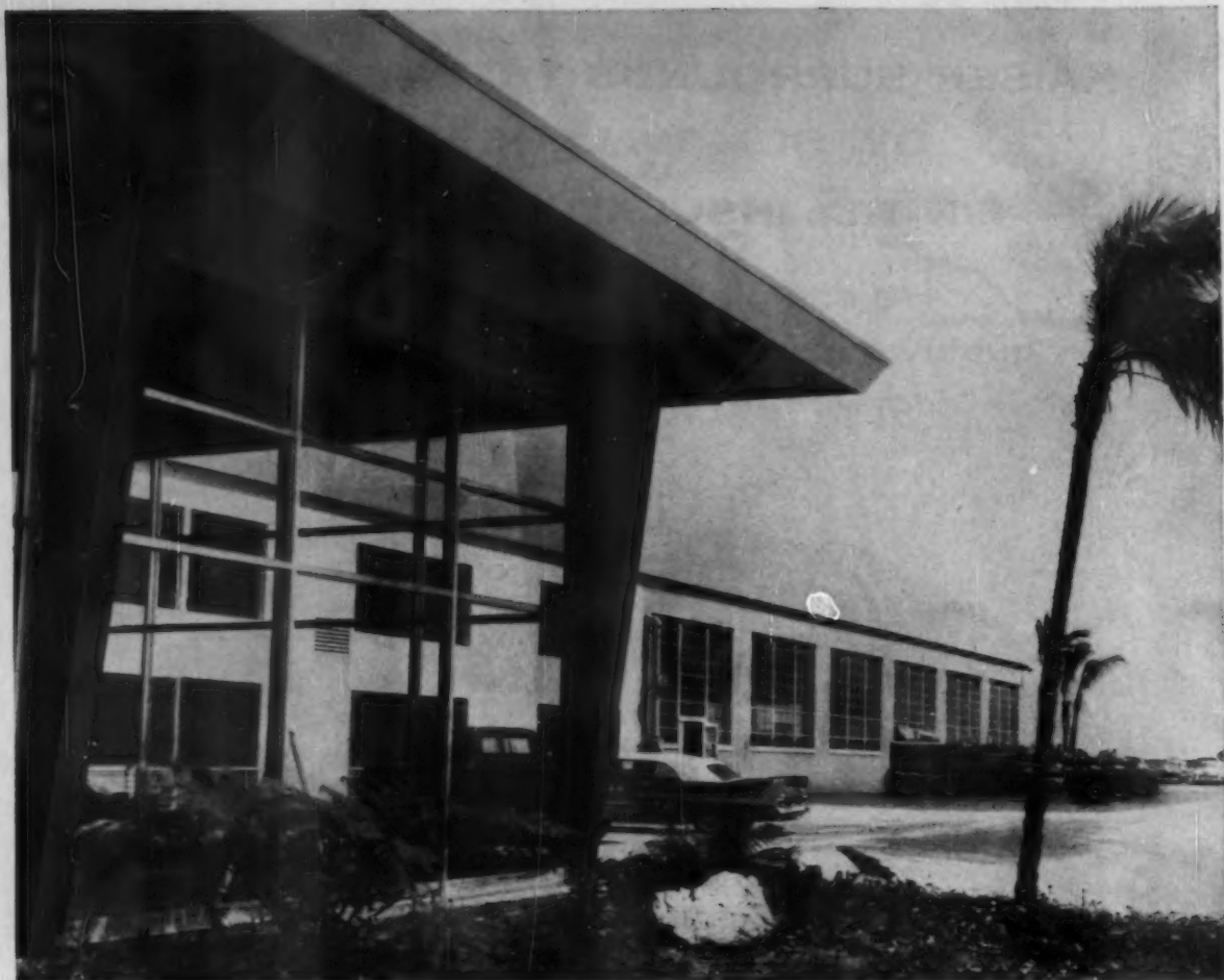
Steel building by Pascoe Steel Corp., Pomona, California
