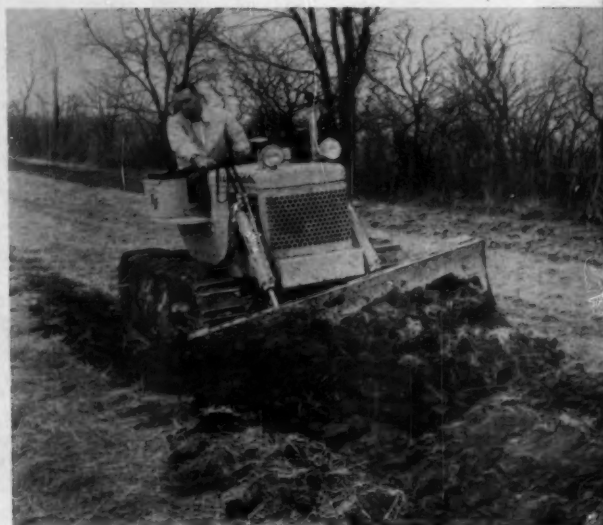
POWER TILTING of the bulldozer blade is a feature of this Case Model "320" Terratractor crawler. Also available is another unit which permits power angling of the blade. Circle No. D71, page 106.
