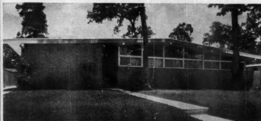
25 THIRD AWARD WINNER by the Monroe Construction Co. of Houston, Tex., is the "Caribbean." Front elevation is designed for privacy from the street, still lets in lots of light from clerestory windows. Price is $19,750 without land; $22,950 with land.
