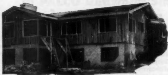
WESTERN RED CEDAR Nu-Loc board and batten siding is being used on this beautiful Wayne, Illinois home.
