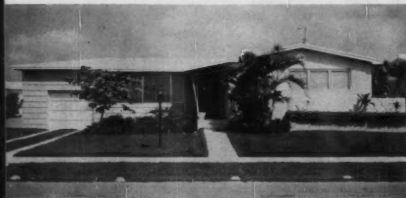
11 A HIGHLY SUCCESSFUL model in Miami's tightly competitive market is this attractive ranch built by Westchester, Inc. It sells for $19,750 including land, approximately $16,000 without. Step-down garage lets house fit slope neatly, saves excavating.
