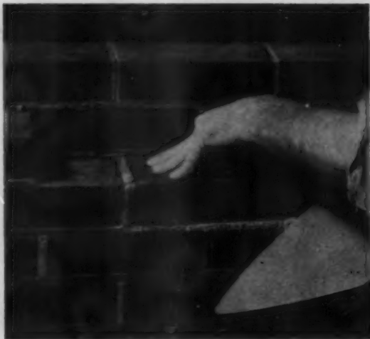
To compare the plasticity of any two mortars, try shoving a brick into place, with a full head
