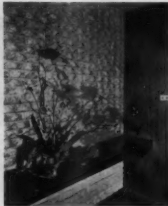
SLUMPSTONE , a specialty concrete masonry block, makes an interesting backdrop for the bench wall. Size: 4x3x24. Mfr.: General Concrete Co.
