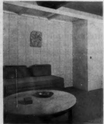
SPECIAL TREATMENT for a concrete block wall. Size: 8x8x16 with a scored line in the middle to resemble 8x8. Palmer and Krisel, architects.
