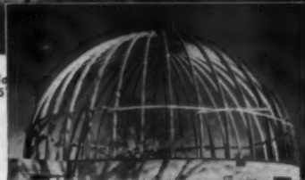
Crown connection — 1' 10 1/4" diameter plate welded to 12" diameter cylinder. Bolts through each arch pass through holes in the plate. The slotted arches abut against the cylinder.
