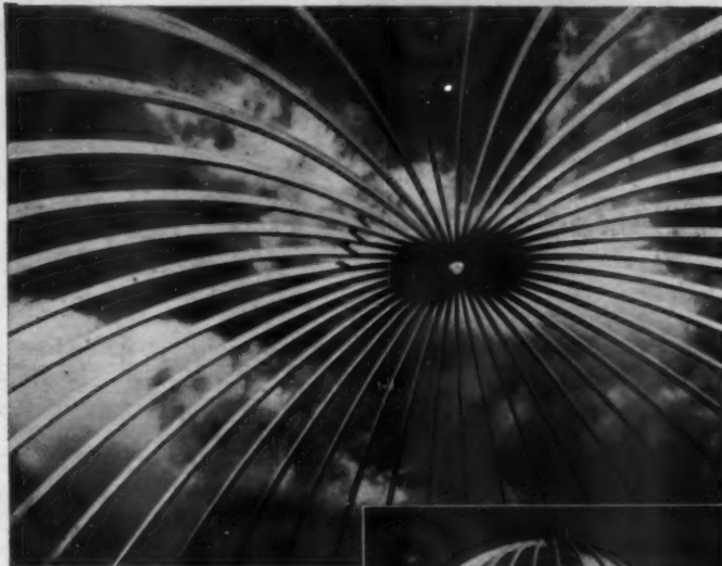
Planetarium, Yorklyn, Delaware Contractor: B. M. Wood, Avondale, Pennsylvania 44 Rilco arches: length 40' 3 1/2", radius 25' center height 25' 7-13/16"
