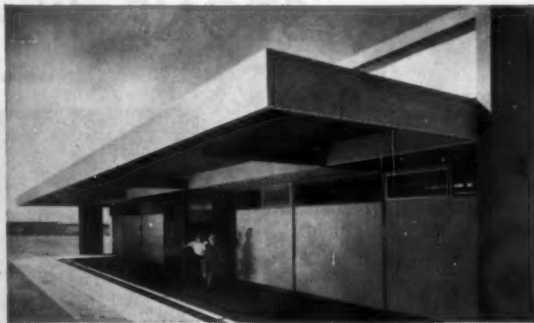
Twin steel wing walls frame the entrance and carry all utilities, hidden . . . but handy, while a floating steel marquee juts from the face to furnish welcome shade on the walkway below.
