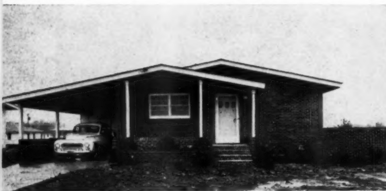
MIDDLE-PRICED MODELS , for $14,550 and $14,950, are shown by builders D. L. Stokes and Jack W. Boone. Wide patio is secluded by 4' wall and joined to living
