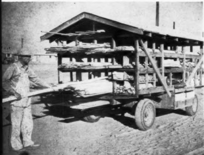
“Trim trailer carries spare parts, is headquarters for finishing crew. A real time saver.”
