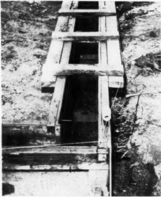
“ Footing forms like these go in fast, are easy to line up, durable, easy to remove.”
