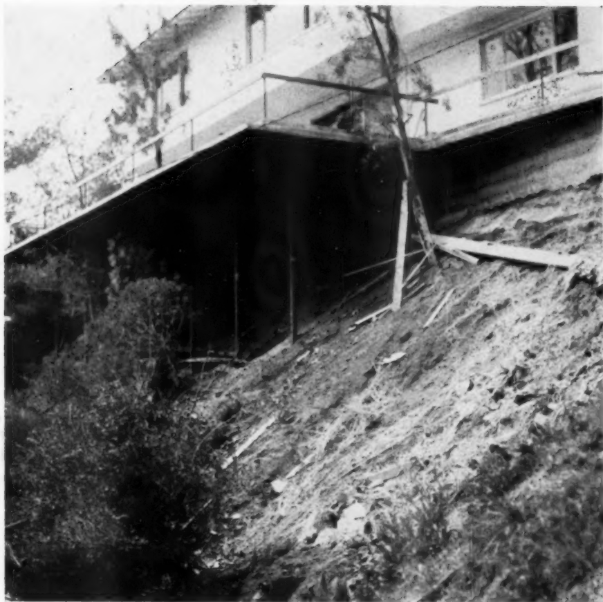
30-DEGREE slope made the adjoining lot too steep to fill. Instead, Barcus designed the house with a deck supported by lally columns. Sketch (lower left) gives him height of columns too.
