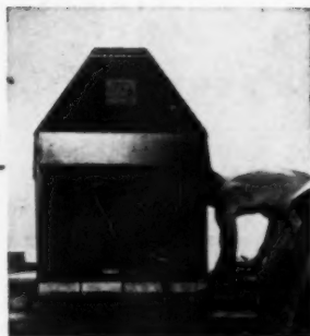
WORKER bricks in around metal form. (Bennett-Ireland)
