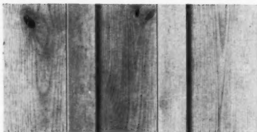
BOARDS AND BATTENS give a snug, economical exterior for cabins.
