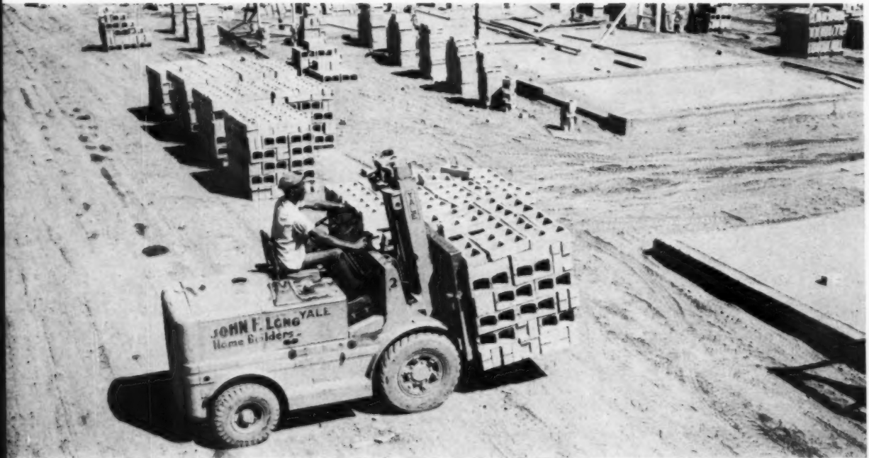
“ This fork lift is a terrific labor saver—spots block piles right where they are needed.”
