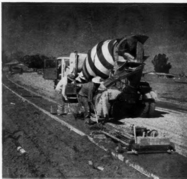
•• Our homemade sidewalk vibrator does the work of four men: handles 600' an hour. It vibrates, screeds and edges in one operation.
