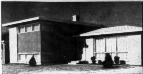
Living room features a window-wall comprised of fixed windows and sliding windows, all set in a tan brick wall. The two-story level uses a brown vertical wood area with windows turning the corner.
