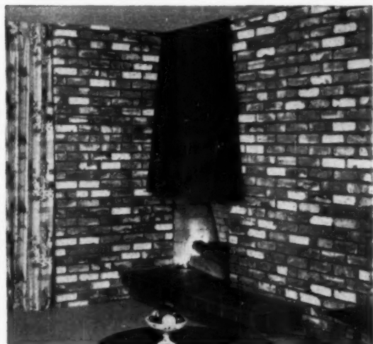
HERE'S a novel way to build a corner fireplace by cutting into only one wall. Yet, heat reflects from both.
