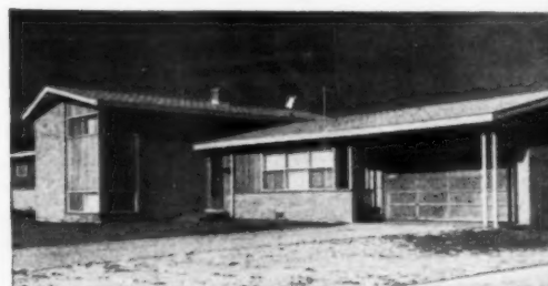
Conventional window treatment was used on the ground level over stone, with wood between door and windows. Corner of the two-story level is treated with windows set in wood, with brick completing the facade.
