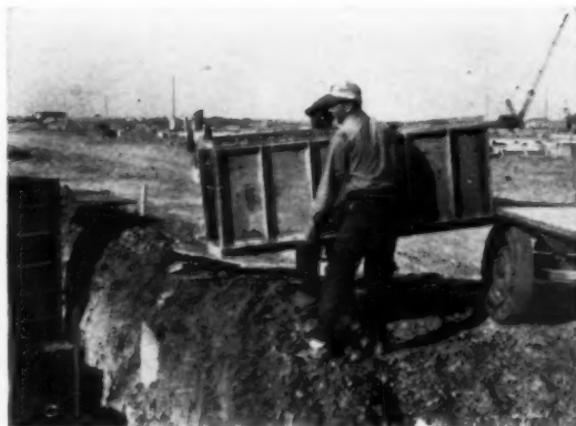
PROPER HANDLING. Careless dumping or throwing may weaken or jar panel, might even break a corner.
