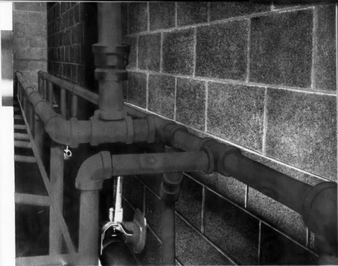
A typical installation of galvanized steel pipe drainage and vent lines in New York's Coliseum.
