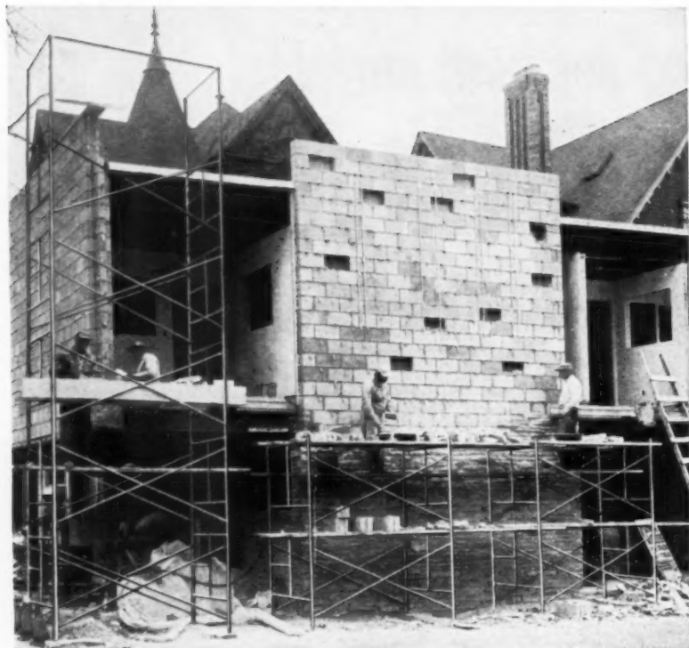
Fatigue Minimized with Waist-Level Material Platforms
