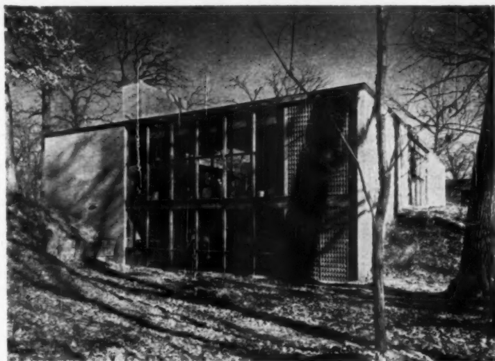
BLEND of brick, glass and louvered wood softens stark exterior.
