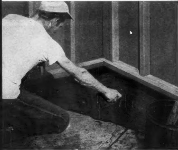
1 Spread mastic over waterproofed slab.
