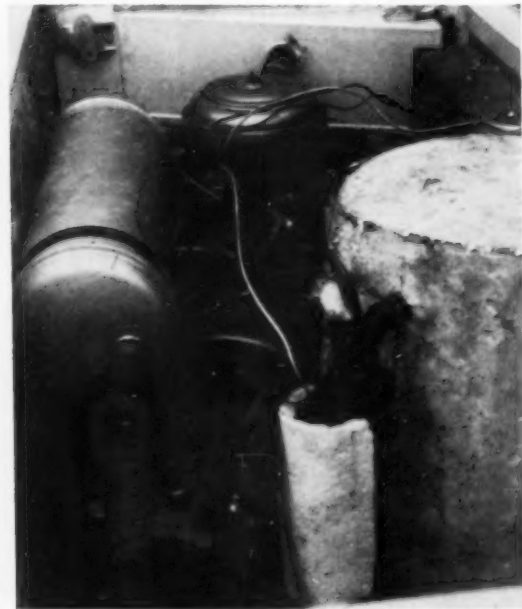
. . . insulated chiller (right), which sends water with anti-freeze to coils in basement. (Shot shows improvement on original unit at left.) Circle No. 8005 on reply card.
