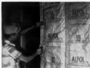
Vapor cannot penetrate the positive, unbroken Alfol seal. No possibility of moisture condensation in walls or ceiling.
