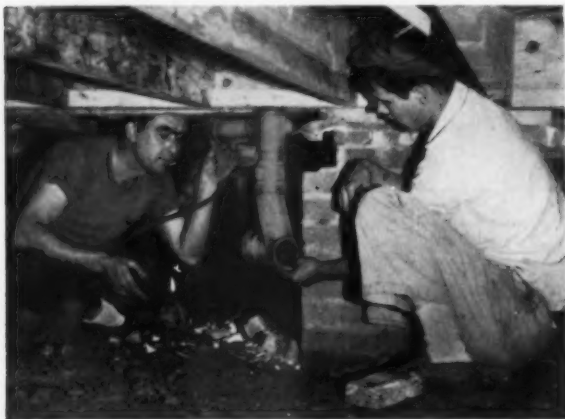
Easy to Handle —"The light weight of copper tube and fittings makes installation easy and fast even in cramped working areas. Our men like to work with copper."
