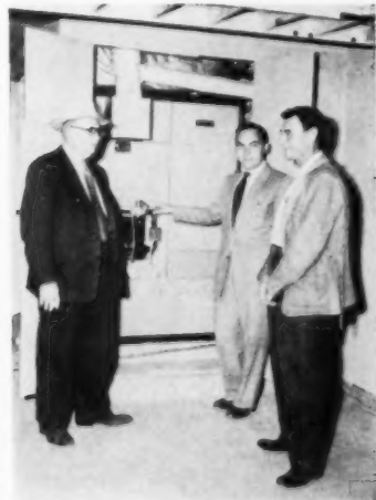
AT RIGHT of year-round Crane unit is cooling coil. Builder: Floyd Harrison (left), Okla. City. No. 8003.
