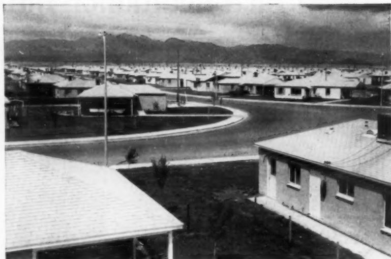
A fire-safe community of 475 homes, all built of 8" lightweight block, in Hyde Park section of Las Vegas
