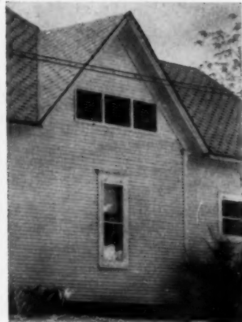
REMODELING JOB includes attic installation of all-in-one air-cooled Lennox unit. (New Products, p. 151.)
