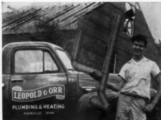
Light Weight —"The light weight of copper tube and fittings makes installation easier and faster—makes possible prefabricated sections like this, for example."
