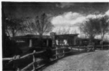
Typical Western home—a tribute to the beauty and versatility of concrete masonry.
