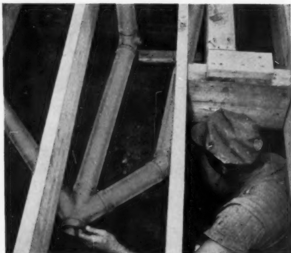
Save Space —"Preassembled sections are connected easily. Stacks with fittings were installed in standard width partitions—gave me an extra 10 square feet of useable floor space."
