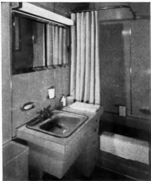
ALL-BLUE BATH off master bedroom has Panelite walls, flush-mounted cabinet with sliding mirrors, built-in lavatory. Shower fittings are made expressly for thin walls, plumbing fixtures are back-to-back with second bathroom.
