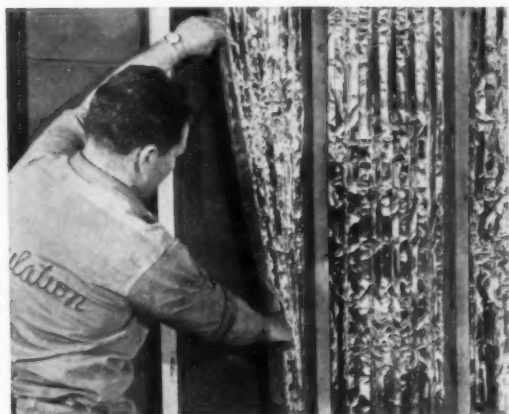
Series of aluminum sheets, with air spaces between, in Infra Accordion insulation. Check reply card No. 7020, p. 148.
