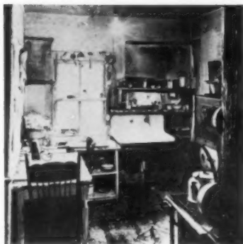
BEFORE: "Architectural guinea pig" kitchen was part of "Operation Demonstrate" program in Cleveland.
