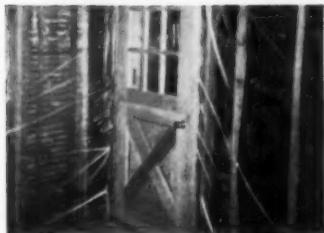
Builders find Olin Polyethylene is of great assistance in sidewall construction . . . retards paint blistering, peeling, staining and helps keep out drafts.
