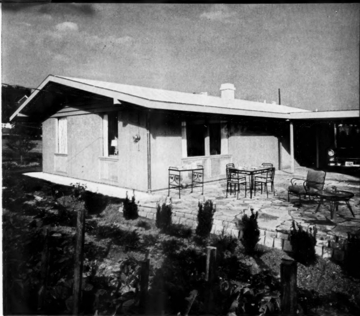
GABLE-END VIEW of house from garden. Note all-over ventilation of gable, deep overhangs above bedroom windows.
