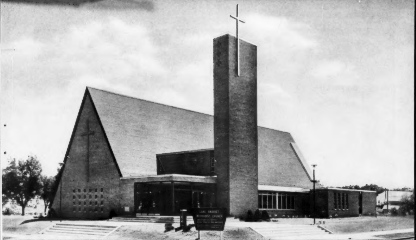
Lake Harriet Methodist Church, Minneapolis, Minn.: Architect, Loren B. Abbett, A.I.A.; Contractor, Kraus-Anderson, Inc.; both of Minneapolis, Minn.
