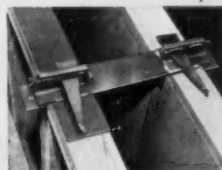
Patented wall aligners automatically give wall of uniform desired thickness and line up tops of panels.
