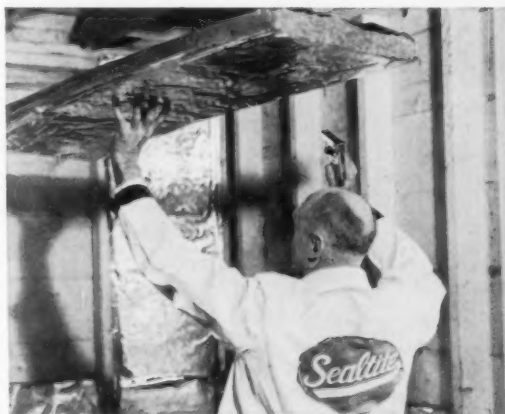
Super Sealfoil, by Sealtite, is a glass fiber blanket wrapped in aluminum. Check reply card No. 7021, p. 148.
