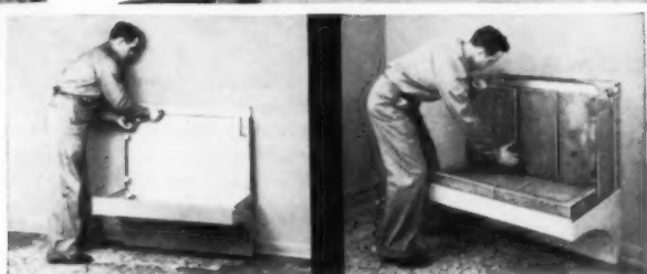
1 Frame is fastened directly to studs with lag screws.
