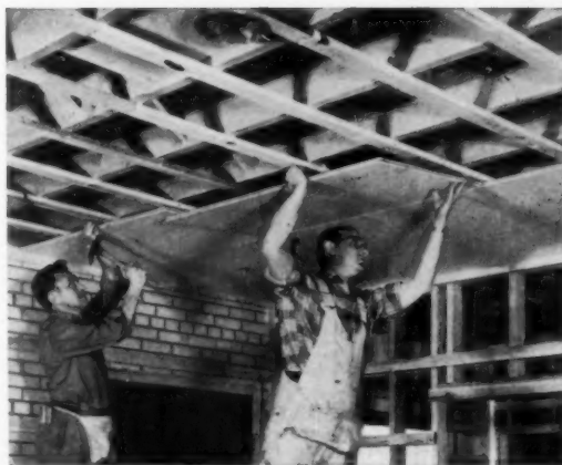
Going up here: a Marlite Korelock ceiling by Marsh Wall Products, Inc. Check reply card No. 7037, p. 148.
