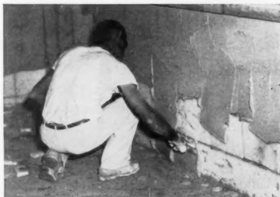
4 PLASTER keys directly to Styrofoam without lathing!
