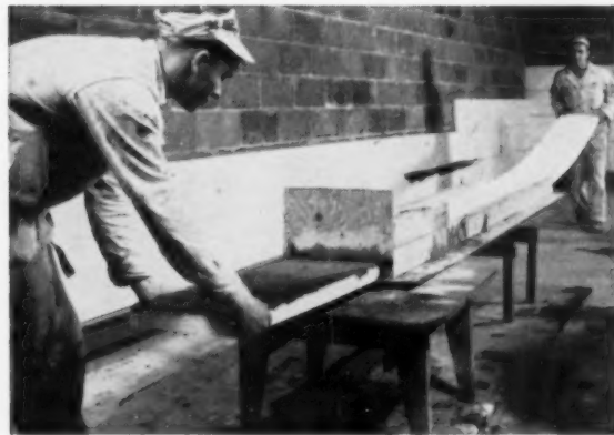
2 MORTAR of portland cement is applied to Styrofoam ...
