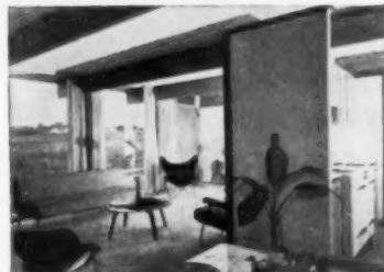
Roof deck also serves as finished ceiling eliminating purlins, joists, bridging, sheathing, lath and plaster.
