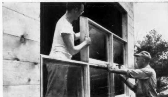
Alternate method for combining Flexivents into large window groups is to build units up right in the window opening. Flexivents come completely packaged ready for immediate assembly and installation.
