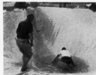
3 LINER SPREAD , the main drain to filter is filled and tested.
