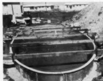
3 TESTING with water; note special backfill mix, joint seam, ribs.
