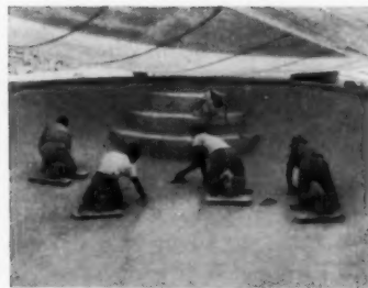
4 HAND TROWELING gives easy-to-clean surface. Shade helps curing.
