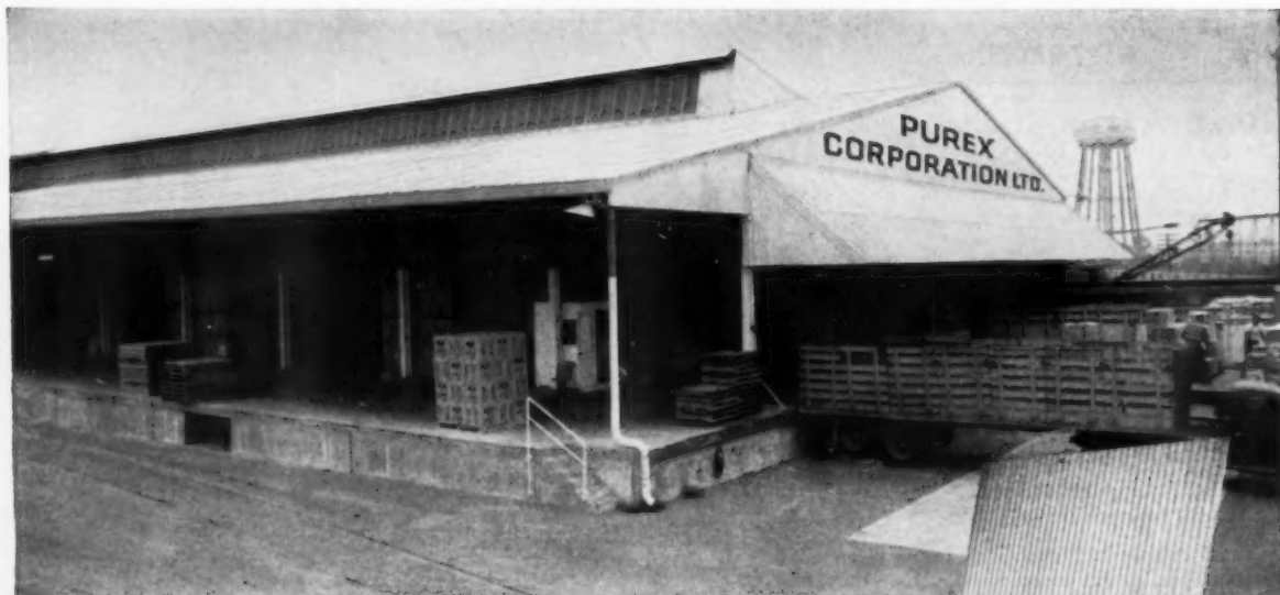
This Purex warehouse, made of Kaiser Aluminum, was designed by Dave R. Edwards Co. and erected by Columbia Structural Steel Co. Highly corrosion-resistant, it will never need painting or protective finish of any kind.
