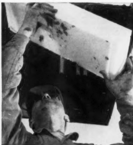
LOW-TEMPERATURE CONSTRUCTION —Unique combination of properties.
