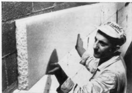
3 STYROFOAM adheres readily to masonry without furring!
