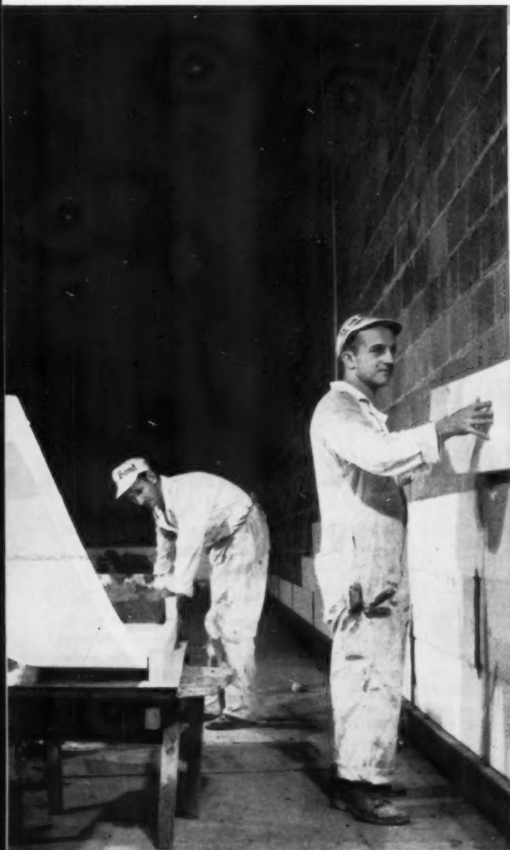
1 MASONRY wall is erected according to usual practice ...
