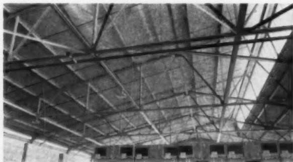
The entire warehouse is illuminated by natural light coming in through the monitor in the roof and reflected by the aluminum ceiling and walls. Note that overhead lighting is not being used.
