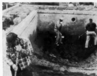
2 BLOCK WALL and coping in place, men tamp earth floor smooth.
