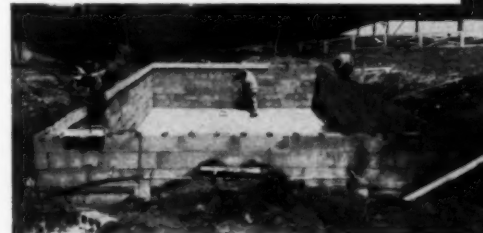
Walls being pre-stressed by tightening nuts above steel bearing plates, after concrete mixture has been poured inside pre-cast concrete sections. Prevents cracking. No forms required.
