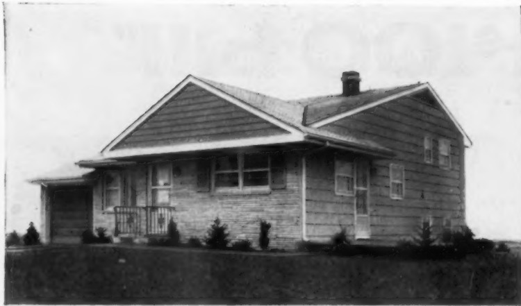
Bellcroft Estates, Bellmawr, N. J. Developed by Cardinal Homes, Inc. Attic fans by Emerson-Electric Builder: Altschuler and O'Dell Designer: Morris Altschuler Electrical Contractor: S. Peskin and Sons
