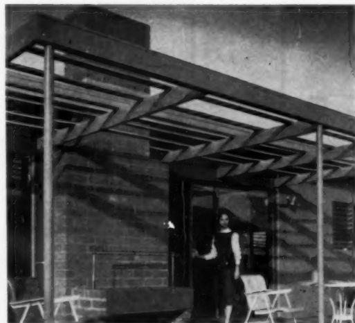
GARDEN PATIO , shown above, is provided by builder as an extra if owner wants it, including 200 sq. ft. of scored concrete and egg-crate roof. Note built-in barbeque.
