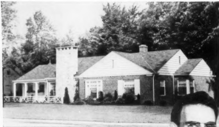
CUSTOM BUILDER —Peter Sepper, Jr., President, The Sepper Construction Co., Fairview Park, Cleveland, Ohio, builder of $25,000—$30,000 1½ story brick ranch-style homes. Plastering Contractor: Tony Delia & Son, Cleveland.
