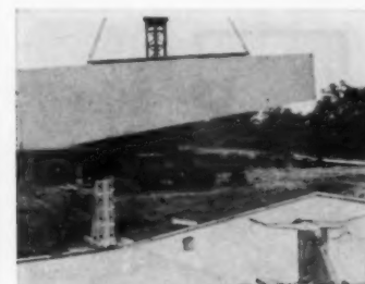
3 PRESTRESSED factory-built wall by Amcrete fits key in laid floor.
