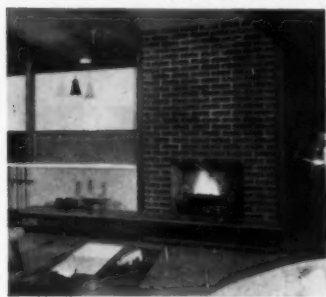
RAISED SLATE HEARTH is almost 10' in length. Angle iron support is tied to posts as well as brick fireplace.
