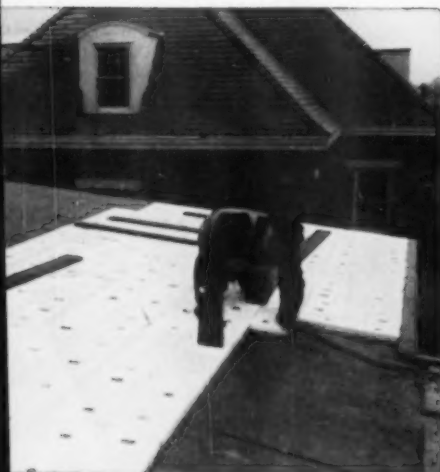
ROOFS —Exceptional strength is combined with light weight to reduce dead load.
