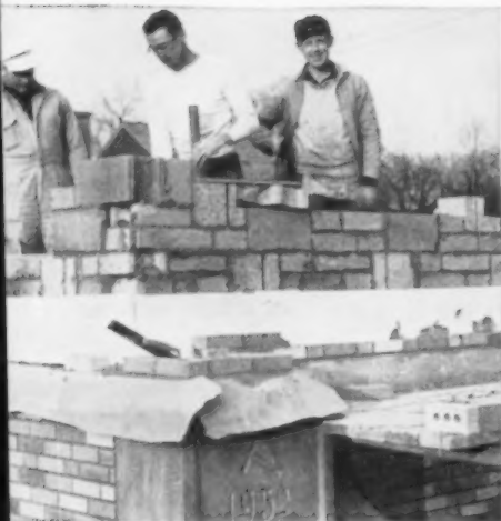
CAVITY WALLS may be constructed with air space on either side of Styrofoam.
