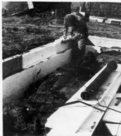
FOUNDATION AND SLABS —Unusually satisfactory with wet-proof Styrofoam.
