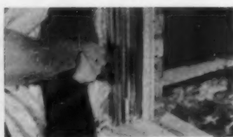
SHORT PIECE of the wood parting bead should be left in place, as a guide.
