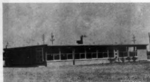
COMPLETE package for National's test project, built in Lafayette, Ind., cost $36,887 for the two-classroom unit.
