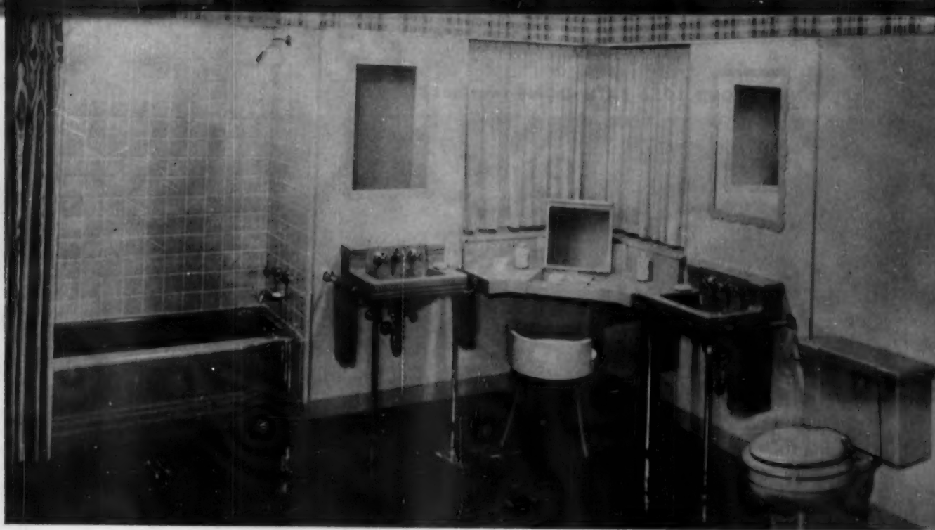
TWIN LAVATORIES flank dressing table with make-up box. For the larger room, a back-to-back arrangement is a novel way to place twin lavatories. Also in larger rooms, prefabricated countertop lavatories with cabinets underneath can effectively be installed in pairs. Or install in bedroom, backed up to bath.
