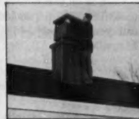
6 Attractive exterior chimney housing completes the installation.
