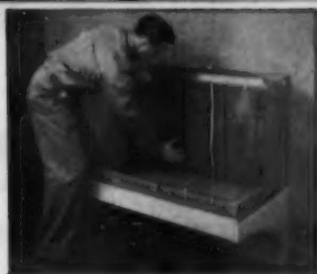
2 Hearth & firebox are formed of interlocking ceramic sections.
