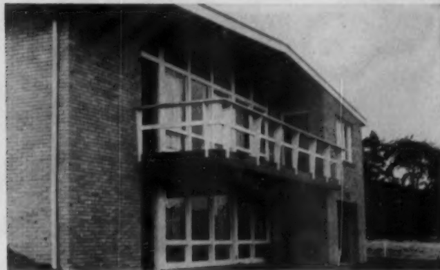
BALCONY outside living room is dominant feature of rear elevation of Pittsburgh Parade house by Amore Co. (see house front on next page), with full-length glass window walls for downstairs playroom too.
