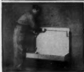
1 Frame is fastened directly to studs with lag screws.
