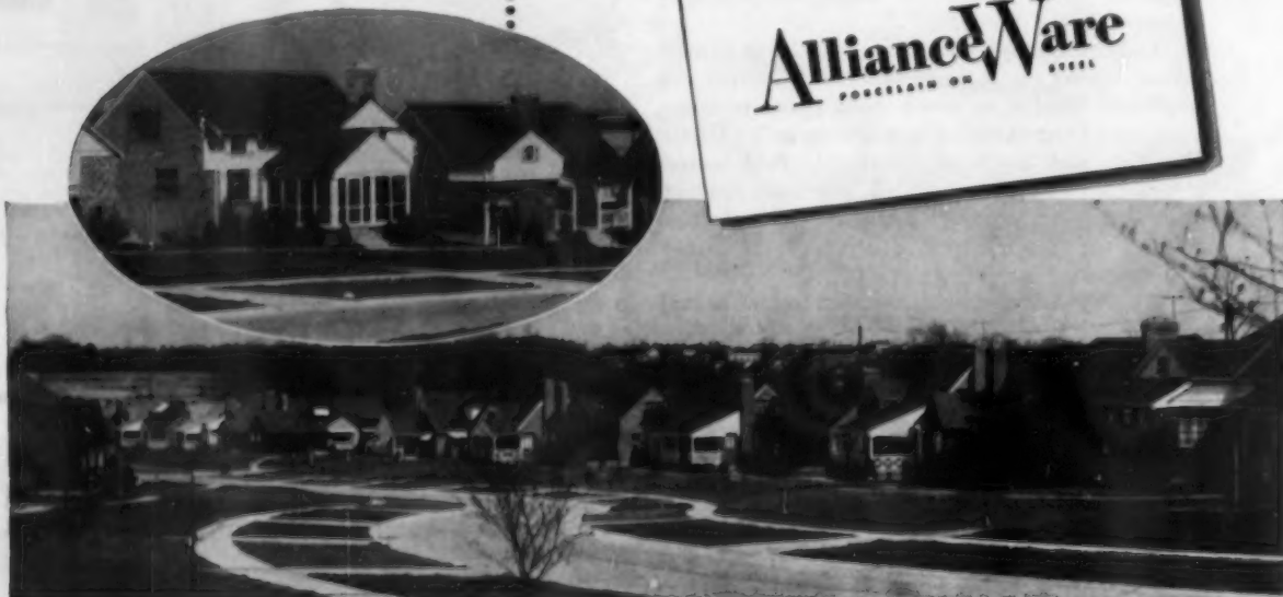
Greenfield Village — Cincinnati, Ohio; Builder: Lang Brothers, Inc.; Plumbing Contractor: Jones Plumbing and Heating Co., Inc.; Plumbing Wholesaler: Main Supply Co.; All of Cincinnati, Ohio
