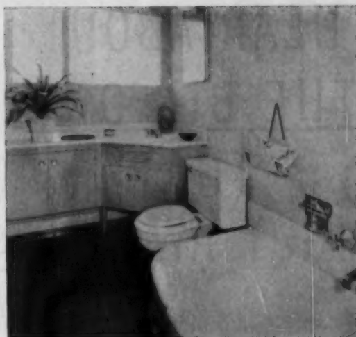
TWO COMPLETE BATHS are included, set back to back to minimize plumbing costs. Sinks are recessed into vanity counters, which extend across entire length of bathrooms.
