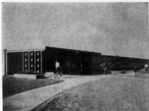
FINISHED schoolhouse is ready for use 21 working days after completion of foundation—combining beauty, economy and utility to a rapidly mushrooming community.
