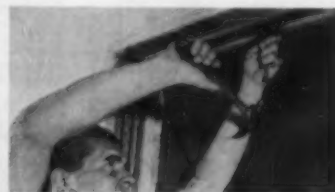
HEAD STRIP must be securely fastened. Seven nails is the absolute minimum.
