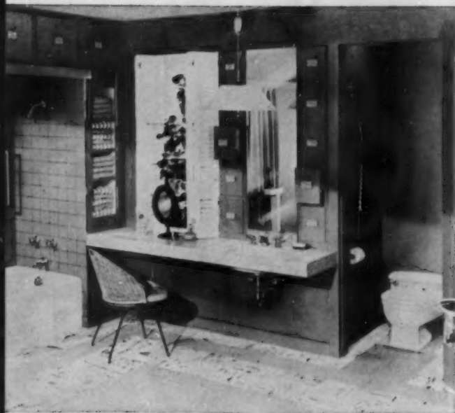
BUILT-IN STORAGE off the floor can be done with wall niches and drawers, as shown here. Then the lavatory may be installed in a running countertop without obstruction underneath. This leaves plenty of leg room under counter.
