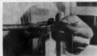
AN 8D NAIL is used in place of hook to secure balance spring to sash.
