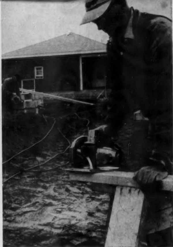
WORKING through openings as small as 6x20 in. and any angle to 70 deg., the Robinson portable conveyor handles 18 bundles of lath per minute, is 16 ft. long, 125 lbs., power supplied by K90R Kohler engine. E. C. Robinson, Dept. AB, 756 S. Broadway, Los Angeles, Calif. Circle No. 1103 on Reader's Reply Card, p. 188.
