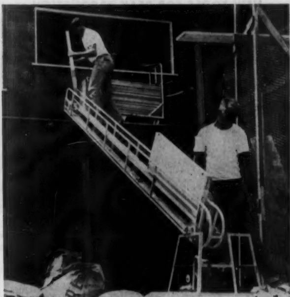
WORKING through openings as small as 6x20 in. and any angle to 70 deg., the Robinson portable conveyor handles 18 bundles of lath per minute, is 16 ft. long, 125 lbs., power supplied by K90R Kohler engine. E. C. Robinson, Dept. AB, 756 S. Broadway, Los Angeles, Calif. Circle No. 1103 on Reader's Reply Card, p. 188.
