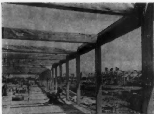
PACKAGED SCHOOL from National Homes utilized 8-ft. module bay system, using 5\frac{1}{8} in. x 6\frac{1}{2} in. laminated columns and 5\frac{1}{4} in. x 11\frac{1}{4} in. laminated beams.
