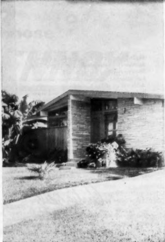
1 Center stone pier on front wall is built out to meet the sweep-back of the roof gable. The division in the use of materials is interesting
