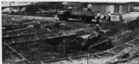
In starting the excavation, power equipment enters the swimming pool at the shallow end. Wood collar is staked in place on three sides with top set to grade, forming the top of Gunite bond beam
