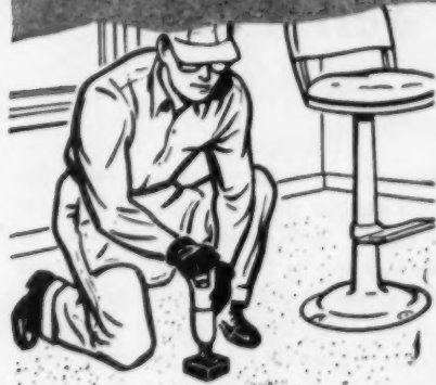
Anchoring seats, bar stools to concrete
