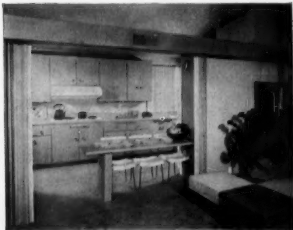
Built-in snack table and kitchen can be concealed by folding door. Note heating duct in exposed position
