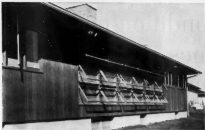
Window wall of awning-type units runs entire width of living-dining area. Each window operates individually for variable ventilation control. House has full basement with fireplace
