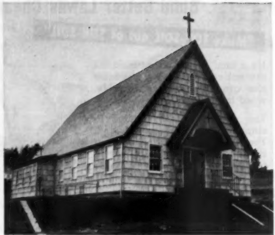
Cedar shakes form the exterior of this new Oregon church. Interior walls are of Douglas fir plywood
