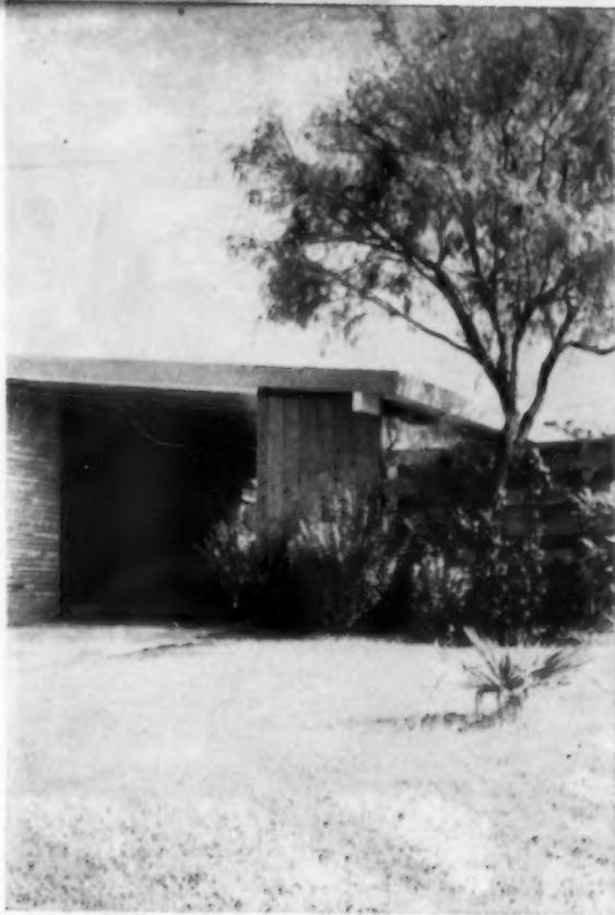
2 This front shows a leveling out of the roof sweep-back over the carport, with a wide sweep of glass across the gable front.
