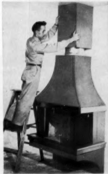
6. HOOD ASSEMBLY is set onto hood support, completing the assembly of fireplace itself
