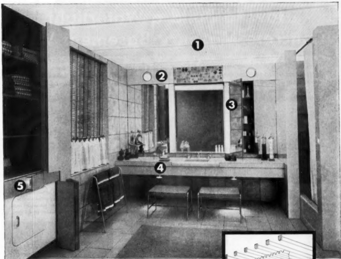
Rows of G-E Deluxe Warm fluorescent lamps are concealed behind panels of corrugated translucent plastic. Panels are lightweight, easy to install.
