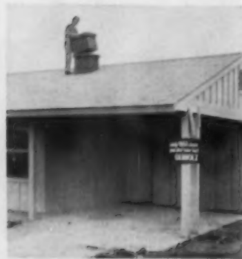
8. Well-designed chimney housing above roof completes installation
