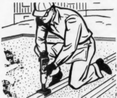
2" x 4" plates to concrete floor
