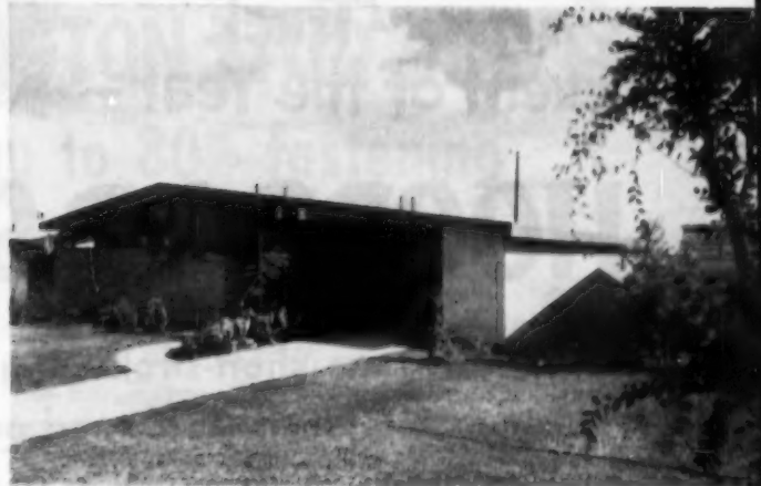
3 In this case a normal roof projection is substituted for the sweep-back. Result is good because of the high planter and the equal division of glass and wall above it.
