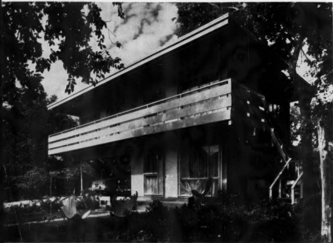
Outside stairs and cantilevered balcony provide access to upstairs units. Building is at extreme rear of 50 x 125-foot lot, has through driveway from front to alley.
