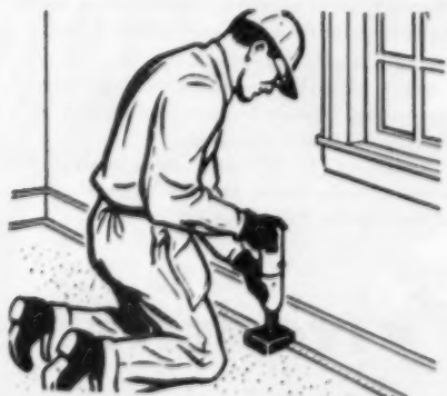
Carpet gripper anchored to concrete
