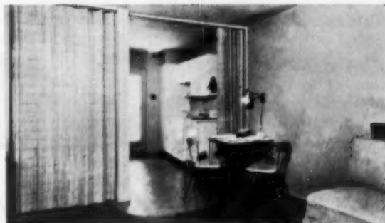
View of kitchen end of typical apartment. Partition walls are of heavy concrete masonry to deaden sound, with precast concrete joist spanning between bearing walls
