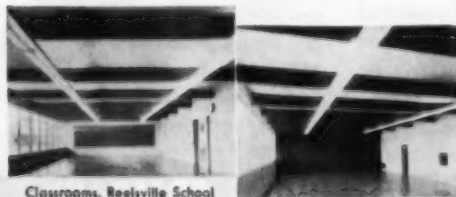
Classrooms, Reelsville School
