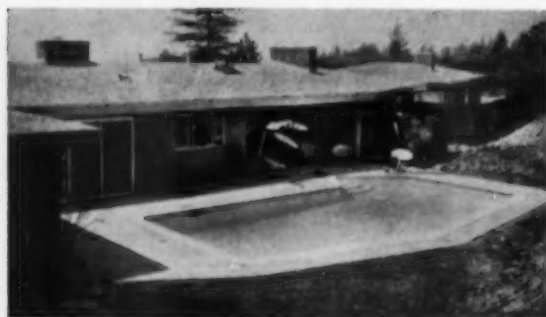
Rough Gunite shell is completed. The coping which is in place is masked off to protect it while the walk areas are installed. Walks must slope 1/4-inch to one-foot away from the pool. Walks can be flagstone, brick or concrete but must be non-slip
