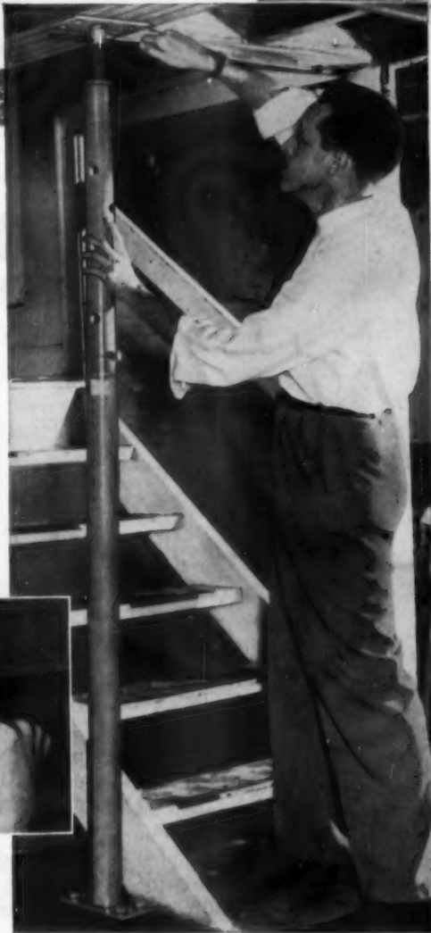
Once TEL-O-POST is mounted in position, just turn the built-in jack to raise the sagging beam. Easier than jacking up your car! After floor has been leveled (per instructions) leave TEL-O-POST permanently in position. Patented locking pin prevents accidents.
