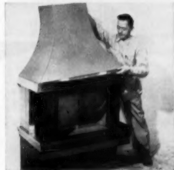
6. HOOD ASSEMBLY is set onto hood support, completing the assembly of fireplace itself
