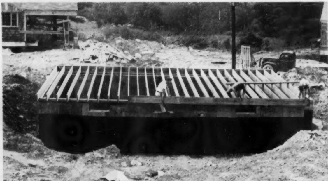
1 Center beams and lally columns are eliminated completely from the houses by using 24-foot long 12-inch floor joists over a 22-foot wide foundation. Three sets of bridging are used for added rigidity.
