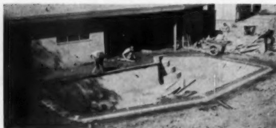
Rough Gunite shell is completed. The coping which is in place is masked off to protect it while the walk areas are installed. Walks must slope 1/4-inch to one-foot away from the pool. Walks can be flagstone, brick or concrete but must be non-slip
