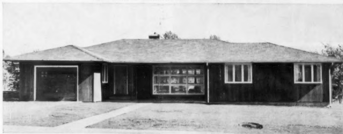
Window wall of awning-type units runs entire width of living-dining area. Each window operates individually for variable ventilation control. House has full basement with fireplace
