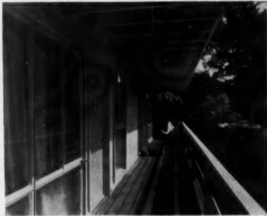
Cantilevered balcony is protected by 5-foot-4-inch overhang, has floor of 2 x 4's.
