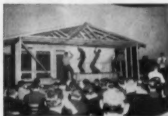
Lu-Re-Co speed: 24x8-ft. section built by four men in 67 minutes during session on components
