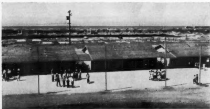
Connecting breezeways will be removed when schoolrooms become homes
