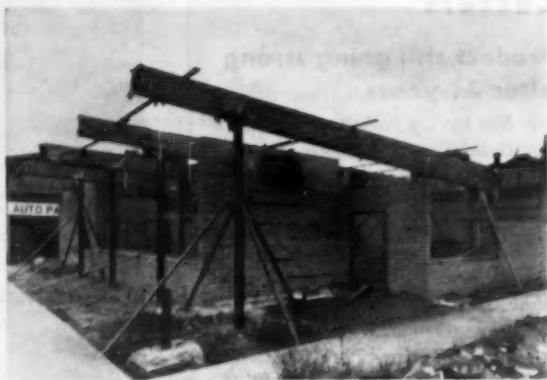
Posts on concrete piers are 6-inch galvanized pipe stanchions spaced 12 feet o.c. Masonry walls are lightweight concrete brick
