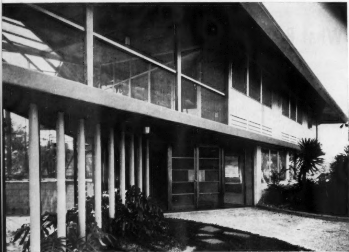
George Ely's houses in St. Petersburg place the main living zone on a concrete slab raised 7 feet off the ground
