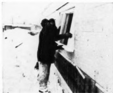
Window frame is pre-primed before cold weather installation
