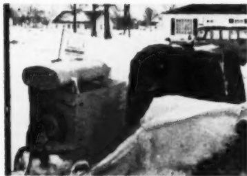
Oil-fired blower heater warms masonry units
