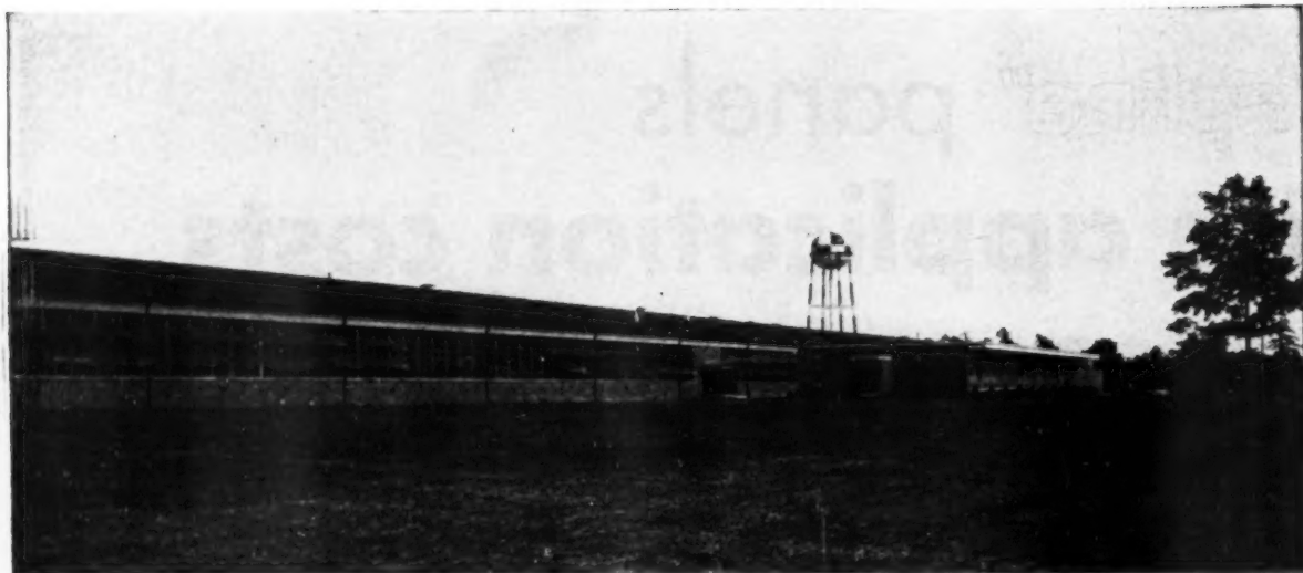
Lenox China Company's new 143,000-sq-ft plant, with attached administrative building, in Atlantic County, New Jersey.
