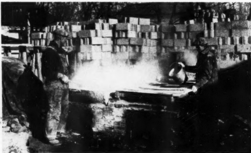
Mortar and masonry need to be warmed when temperature is below 40 degrees
