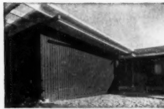
Texture 1-11 meets FHA requirements for combined siding and sheathing which permits major construction economy.
