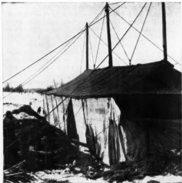
Portable tent covers concrete work in cold or wet weather
