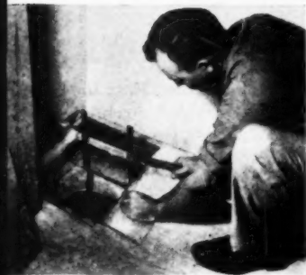
Chimney support with heavy iron support straps is nailed to wood construction members of the floor. Van-Packer installs without special skills.
