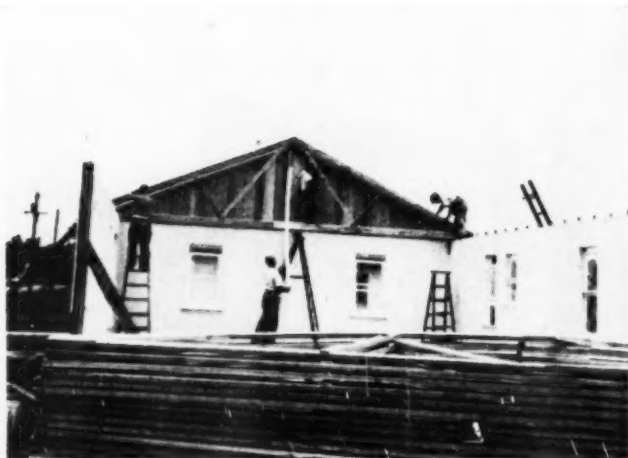
One side of house is left open for easier erection of gable end and trusses. Wall is set up and gable raised after all trusses are positioned
