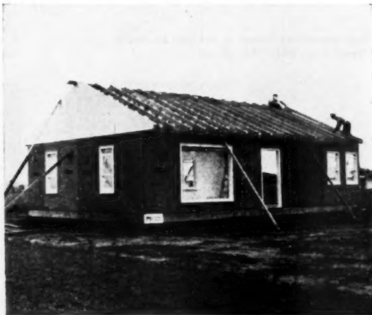
Starting at the subfloor, last truss was put in place after 4½ hours, or 18 man-hours
