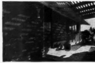
Texture 1-11 siding weathers well, surface texture is enhanced by exposure. Glue is completely weather & waterproof.
