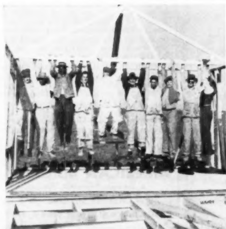
Ten workmen at Inwood Terrace demonstrating strength of truss design used in the 1,500-home addition
