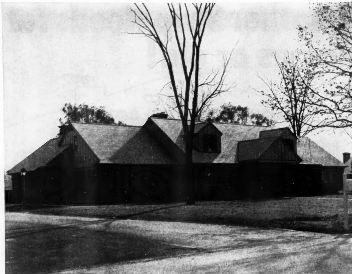
Mr. Allen Dean, one of Toledo's outstanding builders, built this and other prominent homes in Ottawa Hills, Toledo's fine residential area.
