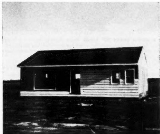
At the end of the second day, or 16 man-hours, most of the roofing and siding is in place
