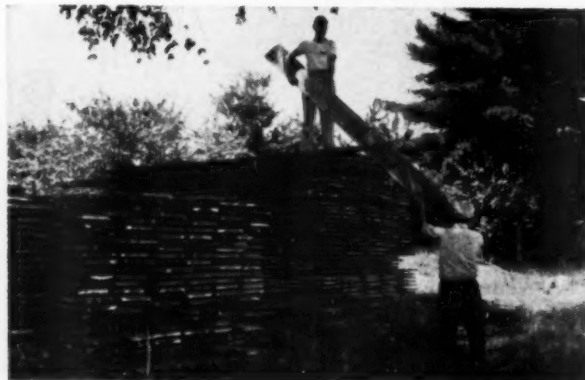
Correct piling of lumber is important in summer. Heat can cause warping
