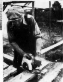
Within 15 1/2 hours after starting to cut the roof rafters for the 92' expanse pictured above, all roof rafters were set and roof boards nailed in place . . . typical of the speed and time-saving made possible by Model 650.
