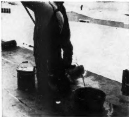
Cold weather application of built-up roof must be on dry surface
