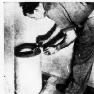
Acid-proof, leak-proof cement joins masonry sections up to desired height. Cement comes in easy-to-use plastic squeeze bags. Each joint is secured with aluminum drawband.
