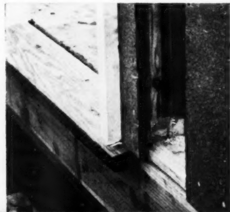
When panels are joined, a 4x4 post is created between each panel (see detail)
