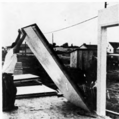
Panels arrive at building site with interior finish already applied and primed
