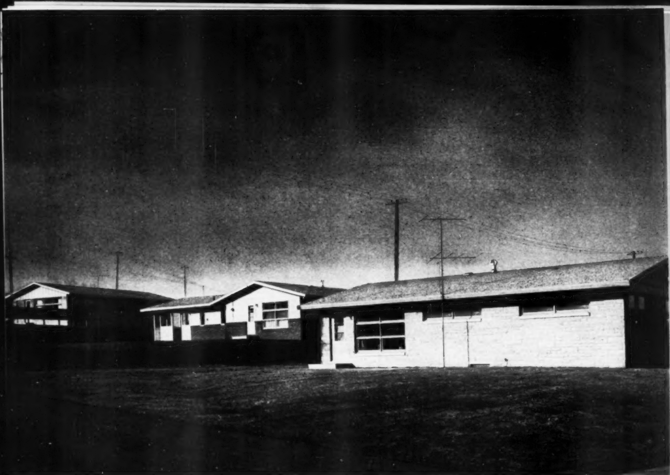
Completed TREND Homes in Strauss Bros. Eastridge Project, Lincoln, Nebraska
