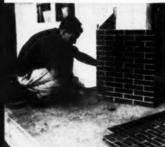
Brick-red cement-asbestos panels are cut to roof pitch, then assembled with corner angle irons and sheet metal screws provided.
