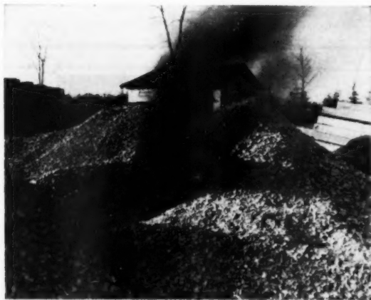
Aggregate must be warmed in cold weather to maintain concrete of 70-80 degrees
