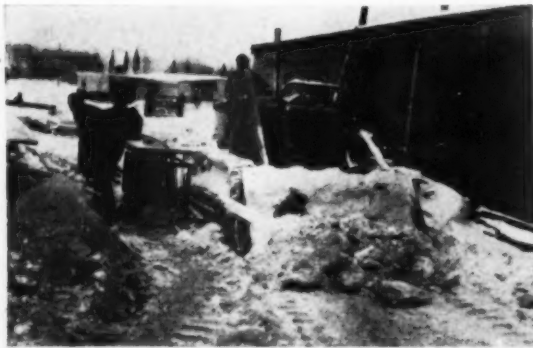
Use your bulldozer to remove snow. Check battery, points, plugs and anti-freeze often in cold weather
