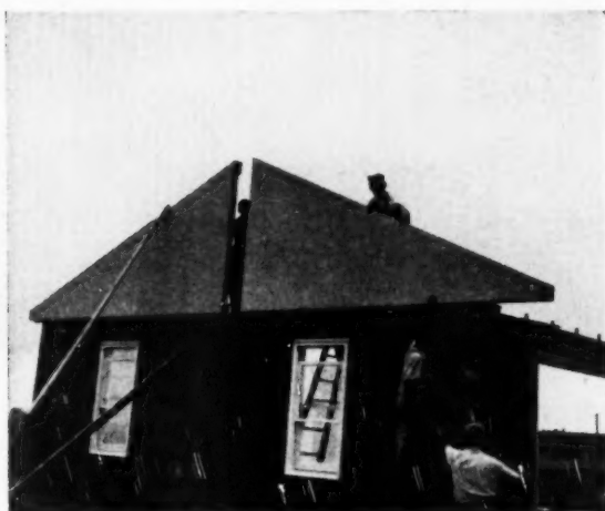
Both gable end units are raised and joined. Gable end units have same chamfered post system as wall panels
