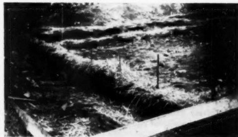
Straw covering protects poured concrete foundations
