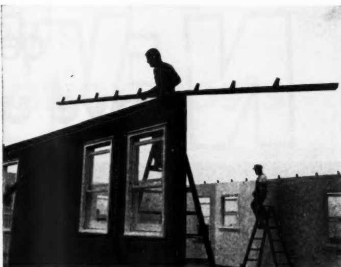
Top plate is shop fabricated with metal fasteners for quick installation of trusses. Hurricane fasteners are positioned 24" o.c.
