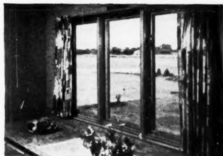
CASEMENT STYLE FLEXIVENT. Sash open outward. Installed in this position Flexivent offers the ideal way to achieve a low-cost casement window.
