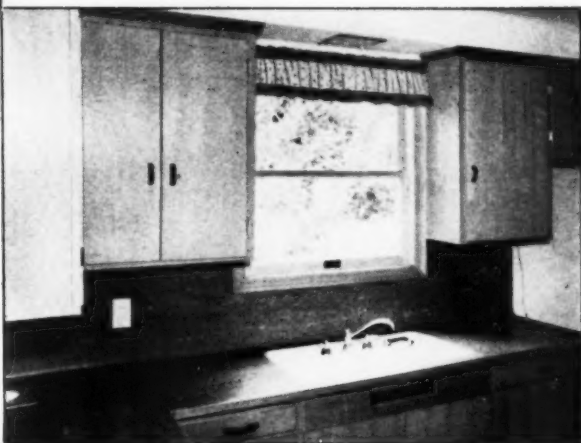
GLUED-UP lumber takes natural finishes very well, and is ideal for a variety of interior uses such as cabinets.
