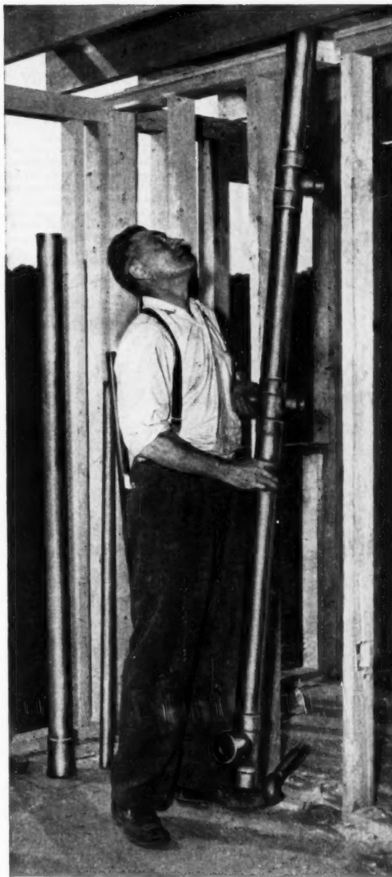
ONE MAN EASILY POSITIONS this 3" prefabricated stack of ANACONDA Type M Copper Tube. The stack fits in a standard width partition.
