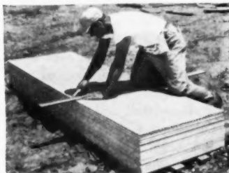
Colorbestos sheets are shipped on a pallet usually containing sufficient material to cover a complete house. Field cutting is kept to a minimum.
