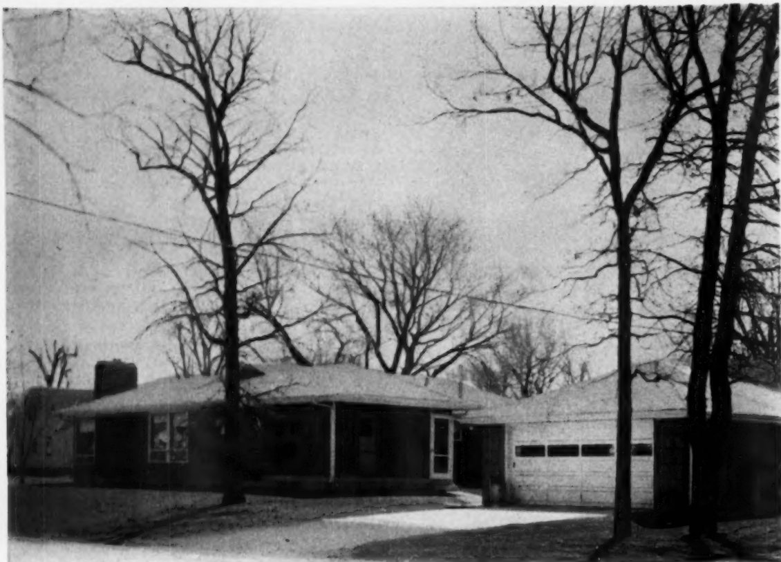
Screened porch placed to rear of kitchen for summer living completes cross of "T"
