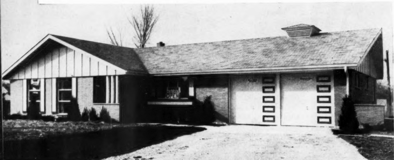
What looks like a model house is a sales office with large material display area and an X-ray exhibit of construction methods
