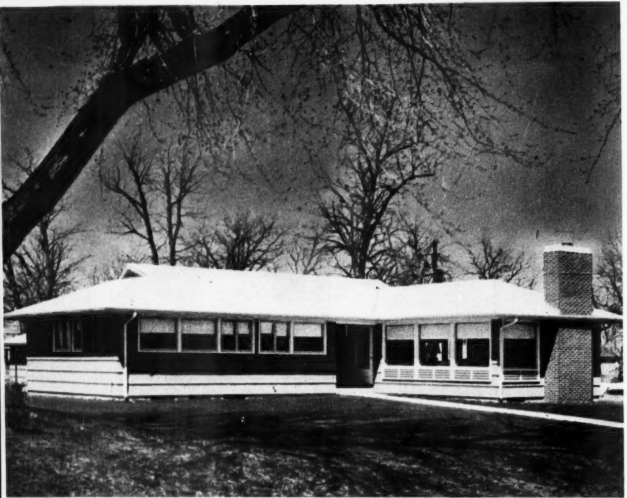
Modularly framed, large glass areas simplify framing. Living room has three exposures
