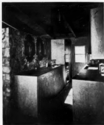
Neatly built-in kitchen has quarry tile counter tops, Thermador range and oven. Soss invisible hinges on cabinets. Note ceiling construction
