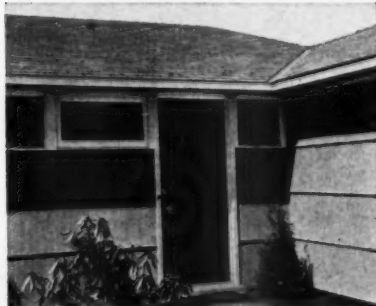
Increasingly popular Weldtex paneling is being used by more and more builders for exteriors, walls and ceilings.
