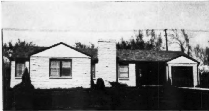
Lincoln, Nebraska builder David Haecker allowed $13,000 for the old house and gave owner 90 days to sell it. The owner sold
