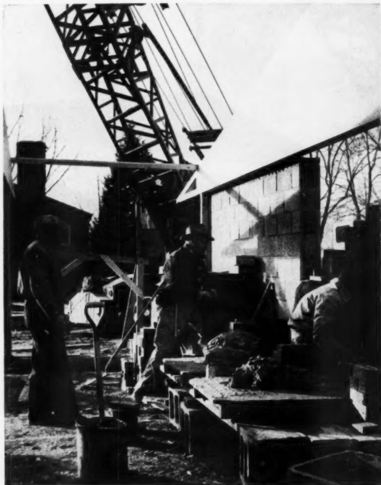
Masonry work is underway while the frames are raised. All trades on the job at the same time reduced construction time
