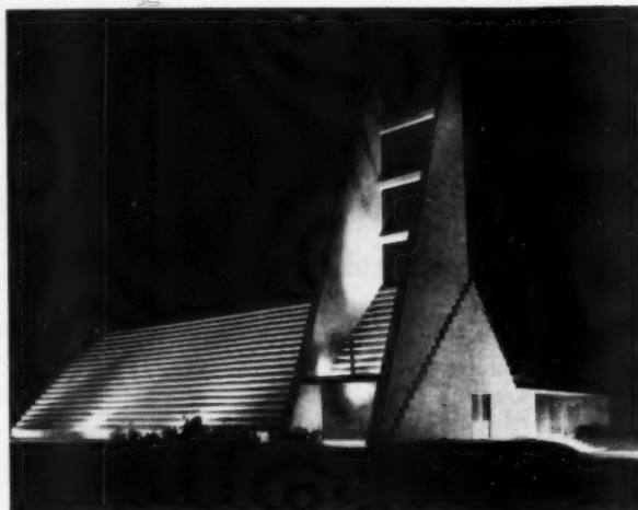
Pylons take the place of the usual steeple
