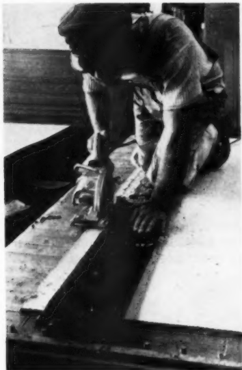
Modules at work. Modular guide pegs speed precutting of dry wall material
