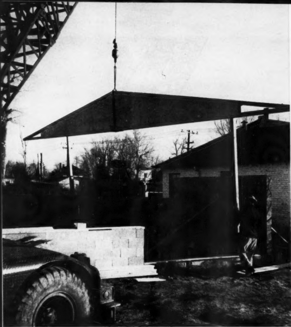
First of the six rigid cantilevered frames is lifted into place. The six units complete structural framing for the entire house. Walls are non-bearing
