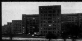
in MULTI APARTMENT UNITS Hunting Tower Apartments, Alexandria, Va. C. H. Tompkins Co., Washington D. C. Contractor
