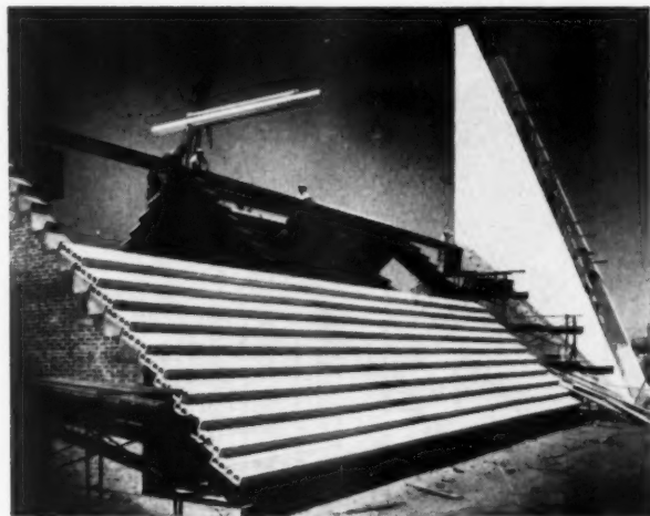
Lifting Flexicore concrete units onto steel trusses spaced 22 feet
