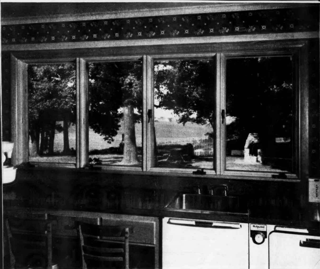
Wide Andersen Casements for both view and ventilation—Charles Klopp, architect, Palatine, Ill.
