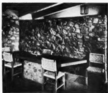
Seven-foot stone wall, laid stone to stone with raked joints, separates kitchen from living space. Table top is hollow core anchored to stone with wood bolts
