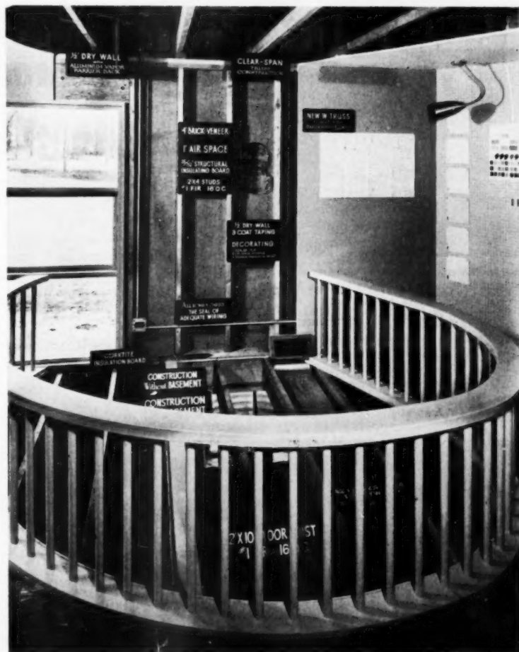
This compact X-ray area exhibits construction methods and building materials used. Walls, floors, ceilings, electrical wiring and heating are shown in X-ray
