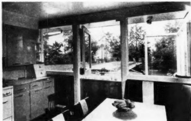
▼ Top panel of Dutch Door maintains continuity of glass wall in kitchen
