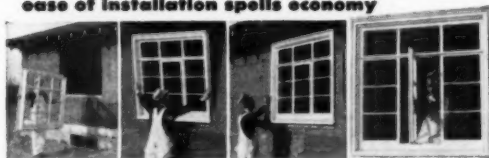
A Complete Window...Ready to Set in the Wall...Nailed in Place...Ready to Use!
