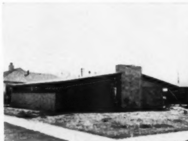
Length of window area in bedrooms shows flexibility of the non-bearing walls
