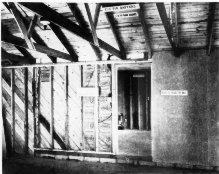
Cutaway in garage shows roof construction, asbestos board fire wall, insulation
