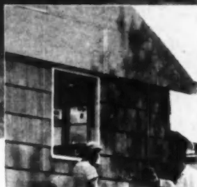
Shingles are applied over fireproof Gold Bond Gypsum Sheathing.
