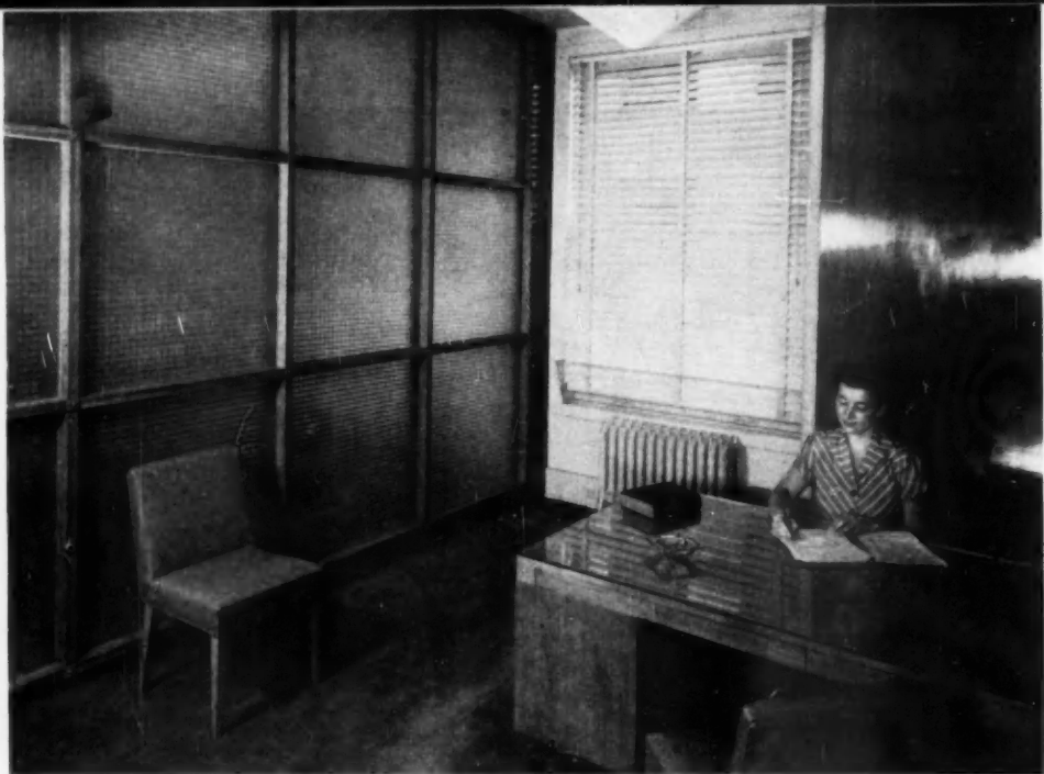
Pre-built to a 3-foot module, assembly would take about a day
