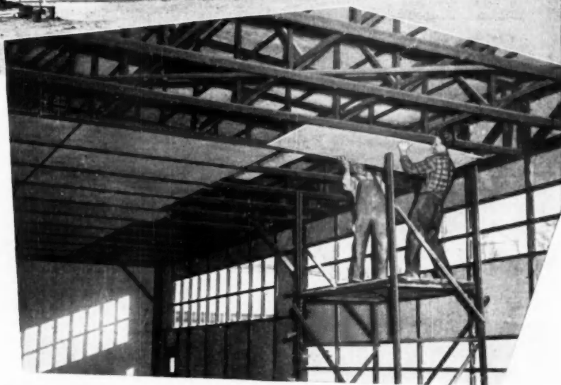
New plant building of the Unistrut Corporation, Wayne, Michigan, where outside and inside walls, ceiling, and roof lining were built of \frac{3}{8} " "Century" APAC asbestos-cement structural sheets.
