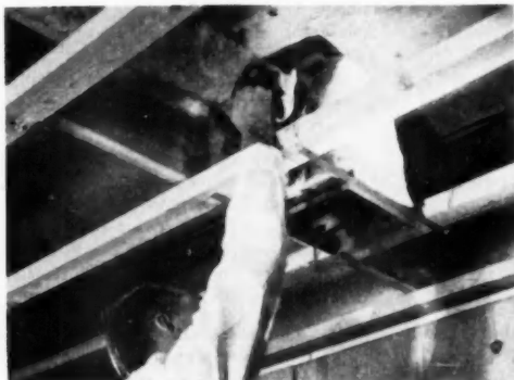
Newest development of system is this ceiling blender. Workman at left is connecting insulated tube and blender box. Air from room is drawn up through long fins of V-shaped grille (right) to join forced heated or cooled air and the resultant mixture is sent back into the room toward large window area
