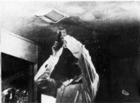
Newest development of system is this ceiling blender. Workman at left is connecting insulated tube and blender box. Air from room is drawn up through long fins of V-shaped grille (right) to join forced heated or cooled air and the resultant mixture is sent back into the room toward large window area
