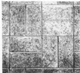
BASKET WEAVE. Laying 8x8x16-in. block in pairs, two vertically and two horizontally, and tooling all the joints results in this woven pattern for interior non-bearing walls.
