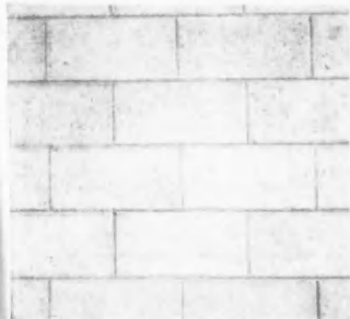
RUNNING BOND. Probably the most widely used pattern of all. Stagger the block in alternate courses so that vertical joints are aligned in every other course. Tool all joints.
