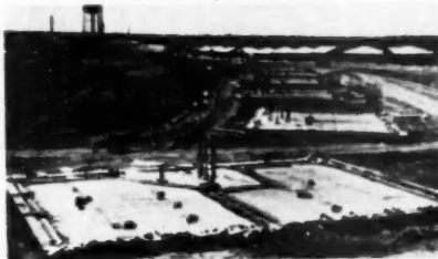
Window units are shown bolted to vertical struts. These are used as jigs for the load bearing walls
