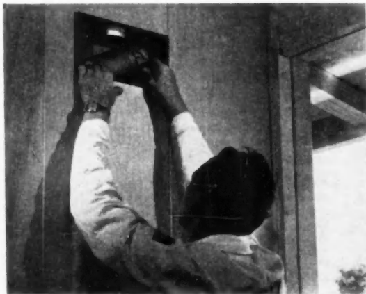
Connecting heat tube to a wall blender before installing grille
