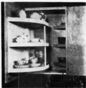
Waste space is eliminated by swing shelves in both wall and base units
