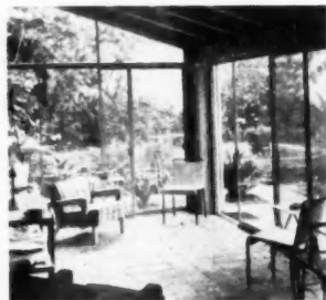
Original studding was removed to make way for Arcadia sliding glass doors, but plates were retained, and corner pillar for support. Fixed crystal was installed above sliding glass at end. Floor is 9 by 9-in. brick tile
