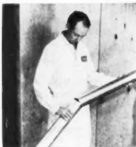
Duct sections of 3½-inch diameter are held together by attached clamps
