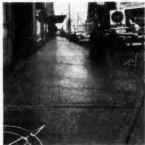
Finished non-skid sidewalk. When its temperature falls to 37 degrees F., the snowmelting system automatically starts working
