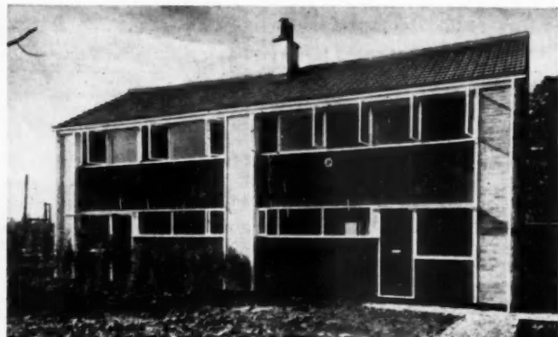
A duplex arrangement. The apron area below first and second floor windows is finished in dark red spatter dash stucco.
