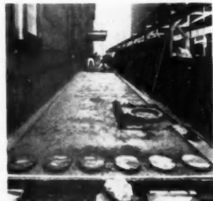
Screeding vermiculite insulating concrete base for the snowmelter which protects the sidewalks around Pittsburgh's William Penn Hotel
