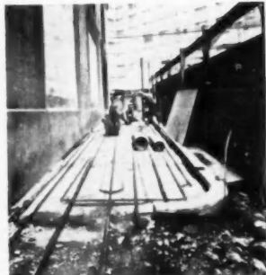
Installing waterproof paper under radiant heat coils
