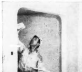
Fireproof Gold Bond Gypsum Lath is finished with Gold Bond Plaster and Finish Lime.
