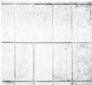
VERTICAL STACKING. Like horizontal stacking except that the block are laid on end. This unusual pattern creates illusion of greater height for interior non-bearing walls.
