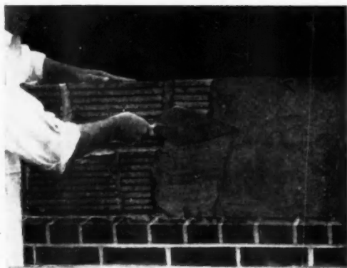
If the back-up units are laid first, the front of the back-up units should be plastered.
