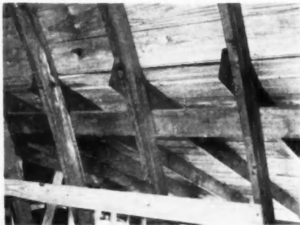
Laminated rafters are 16 inches on center. Ledger strip supports the 2x6 shed roof rafter. Shed rafter is bolted to the laminated rafter. Roof sheathing is 1x6 D&M
