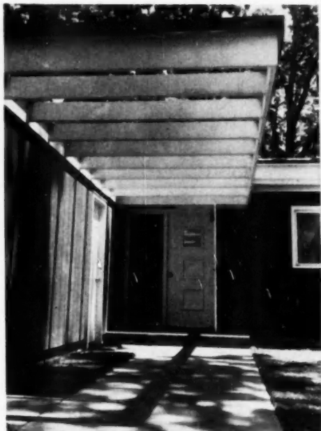
Open canopy, recessed door with look-through mirror, corrugated glass panel lend distinction to entrance. Note garage door at left
