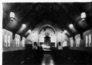
CHURCHES find concrete masonry construction both practical and economical.
