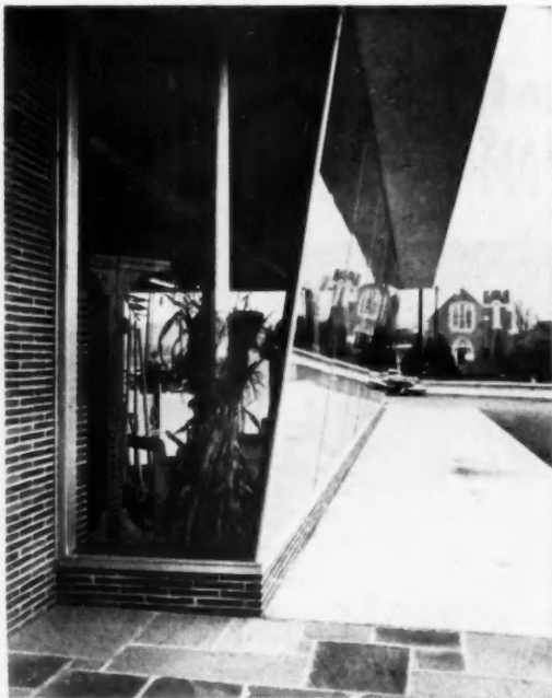
Slanted windows of showroom are 12 feet high, have 9 degree pitch
