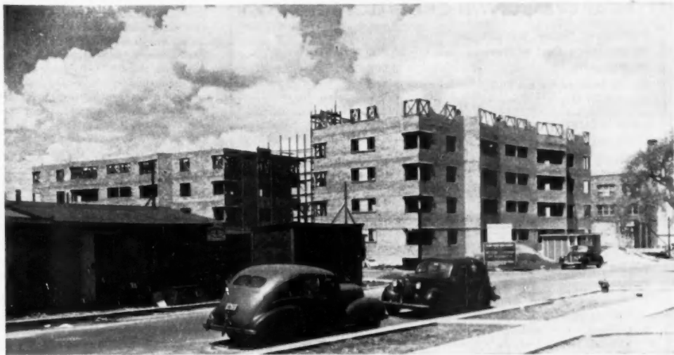
Winchester-Hood apartments in process of construction
