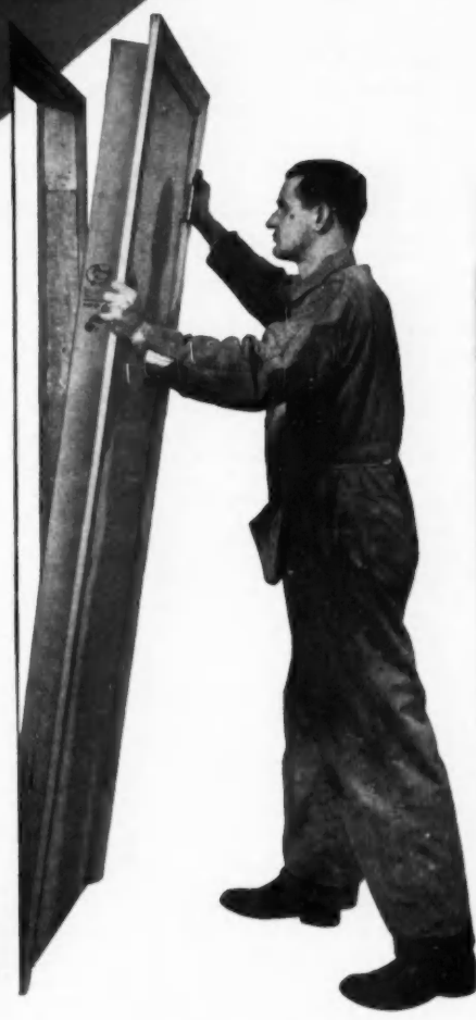
Slide other half into opposite side and nail to wall.
