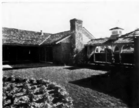
ROOF overhangs the concrete about 10 feet, gives protection from sun and rain yet permits plenty of light for interior. Fencing the passage from house to garage gives privacy from the street
