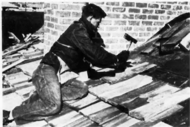
Double coverage is used in the valleys. A regular 18-inch valley roll is laid first. Second, shingles are laid across the valley. Third, shingles are carried to the center of the valley. A chalk line is struck to cut the valley line
