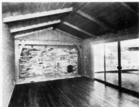
GARDEN wall of den-dining room has Arcadia sliding glass doors with sliding screens outside. Ceiling is 1 x 16 boards lapped with 2 x 6 rafter exposed on 4-foot centers
