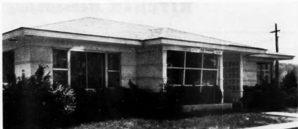
Brick ledge between every two courses of insulated concrete block gives shadow line which emphasizes horizontal lines of the building
