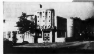
COMMERCIAL ESTABLISHMENTS utilize various types of block to modernize their building.
