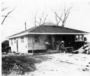
COMPLETING EXTERIOR of House No. 2
