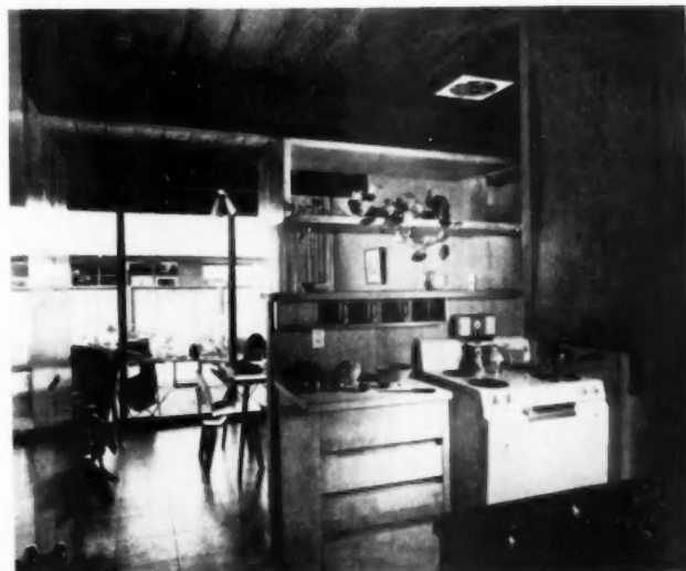
PORTION of kitchen, showing dining space and patio beyond. Kitchens have unusual number of cabinets, in wood, with Formica tops on work counters; ventilating fan
