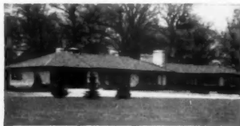
Here is one of builder Chet Bojarski's typical Moduflow-Radiant Heat "combinations"—the beautiful 8-room rambler-type home of Mr. and Mrs. Claude Klingaman, Gary, Indiana. For details see the floor plan on next page.
