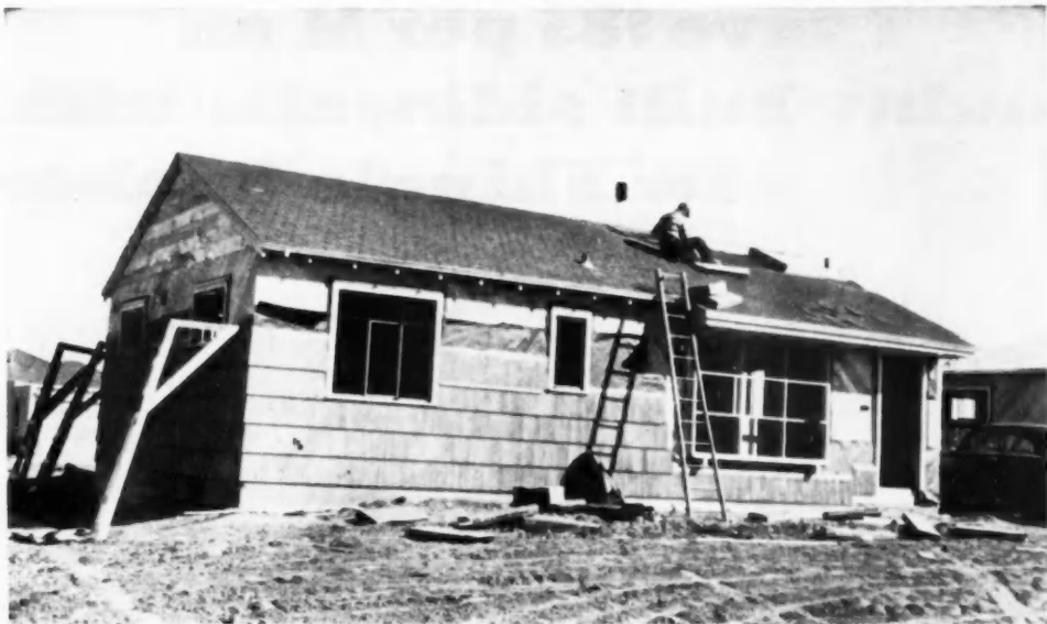
One man roofing a 1000 square foot house in one day. Price for an asbestos siding, asphalt roofing job on a 720 square foot house is $355
