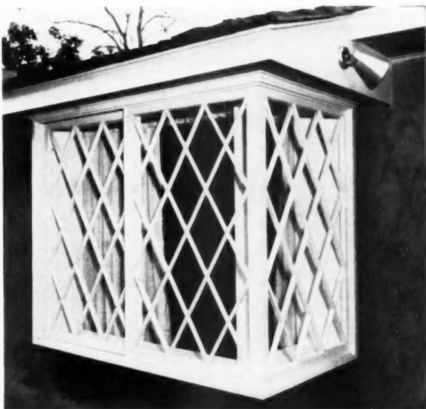
Diagonal mullioned box window in bedroom No. 2 makes a point of unusual interest on the exterior, provides an attractive window seat within
