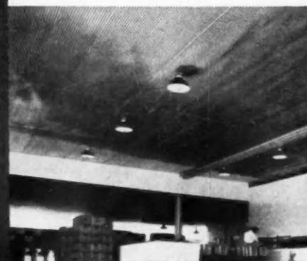
Kaiser Aluminum Roofing is effectively used as a ceiling liner in a Golden State Dairy building at Van Nuys, California. Because it is so easy to clean, aluminum contributes to maximum sanitation. Because it's solid aluminum—not clad or veneered—this ceiling is highly resistant to rust and corrosion. Never requires painting. Virtually maintenance-free. Strong—durable—lasts for years. And because aluminum is so light in weight, it is far easier to install.
