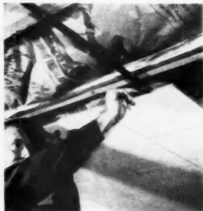
Suspended acoustical tile ceiling system easily spans four feet, through support by concealed T-splines
