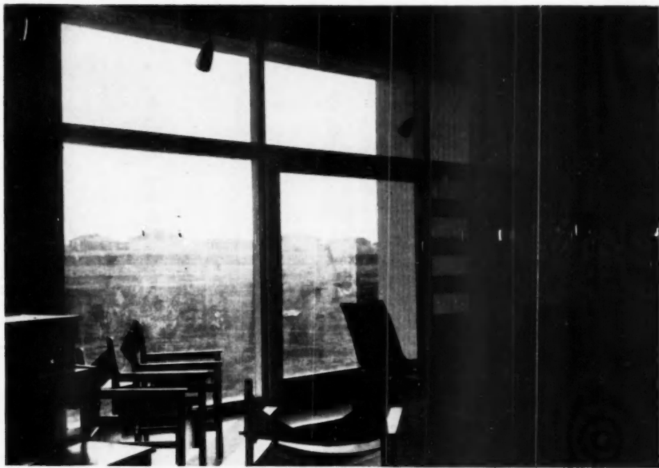
SLIDING WALL arrangement in living room. Large glass area next to utility windows slides on floor track
