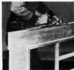
Fitting storm sash.
