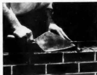
Method 2. A dab of mortar should be spotted on the corner of the brick already in place.
