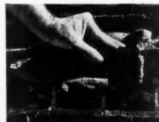
Then the brick should be shoved into this deep bed of mortar.
