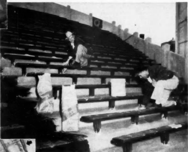
Above photograph shows THOROSEAL FOUNDATION COATING being grouted into upper, or wearing, surface of bleacher seats.
