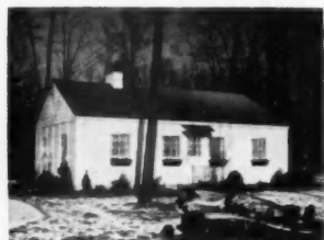
All-steel prefab demonstration house built by Gunnison Homes in Pearl River, N. Y.
