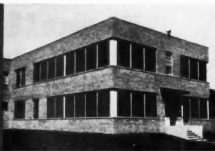
Kaiser Aluminum Shade Screening on New Jersey offices of Chilcote Laboratories made air-conditioning feasible. Tiny louvers stop hot sun rays before they hit the glass, reducing heat to controllable levels. Glare effectively reduced. Soft, adequate illumination lessens eye-fatigue. Anodized finish requires no maintenance, no painting. Hinging makes windows easily accessible for cleaning.
