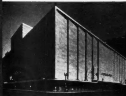
Kaiser Aluminum Ductwork in Foley's Federated Department Store in Houston fabricated on the jobsite. Highly workable, easily joinable by standard methods, aluminum ducts were installed with less worker fatigue, less wear on equipment. Pound for pound, aluminum ductwork has three times the working surface of steel. Uninsulated, it delivers as much heat as insulated galvanized material.
