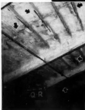
Right photograph shows soffits of concrete seats where concrete has blistered away from reinforcing rods. Rods were sand-blasted and sealed with THORITE Patching Mortar and entire undersurface sealed with THOROSEAL.
