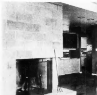
SIMPLE FIREPLACE of concrete block has modern lines. Hearth is built up eight inches. Kitchen area is at right. Rear of fireplace has a built-in wood box. Hall opens to den
