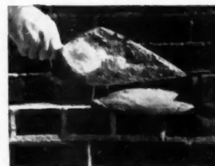
Method 3. A full trowel of mortar should be thrown on the wall.
