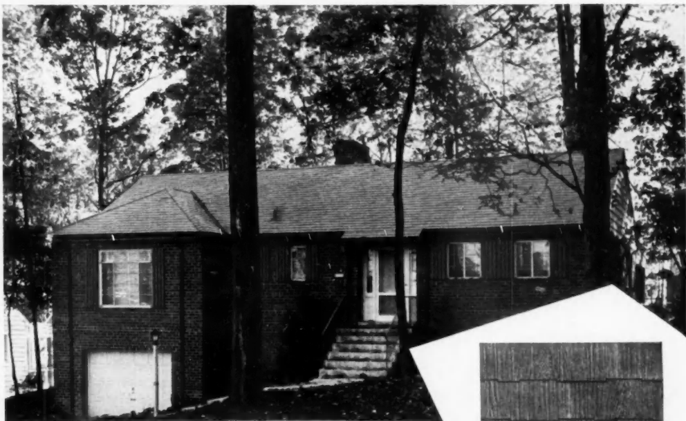
New Silver Spring, Md. residence roofed with "Century" No. 5 Spanish Red Asbestos Shingles. APPLICATOR: L. A. Lee and ARCHITECT: Louis R. Moss, both of Washington, D. C.
