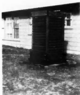
ATMOSPHERE TOWER is housed in the rear yard. This unit dissipates heat built up by the air conditioning equipment. Below, atmosphere tower schematic diagram showing operation and parts
