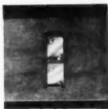
Simple floor guides, installed flush with finished floor, eliminate need for floor track.
