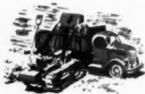
Loading out scrap material
