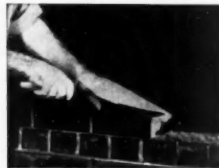
Then plenty of mortar should be thrown on the end of the brick already in place.
