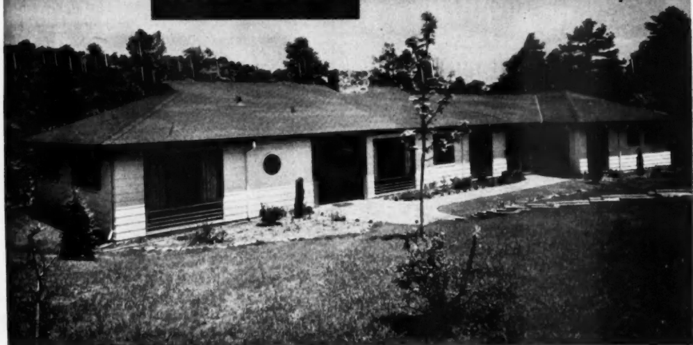
This Knoxville house designed by Mr. Bartling and built by Fonde-Bartling, has exterior of weatherboard concrete block, electric ceiling radiant heat, and louver type sash. And the two water heaters . . . of course, they're ELECTRIC!
