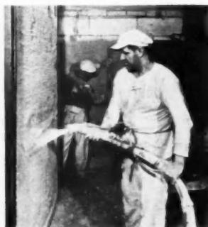
PLASTER spray gun application
