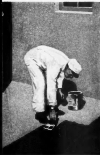
PAINTING INTERIOR MASONRY
