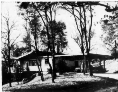
Architect: Chloethiel W. Smith General Contractors: Manning-Winthrop Corp.
