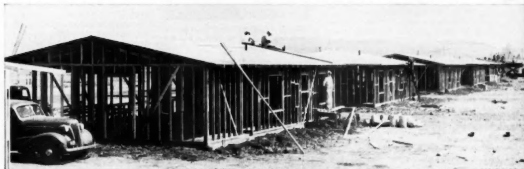
SPECIALIZED WORKING CREWS of four members each move from house to house, one man in each crew acted as its foreman
