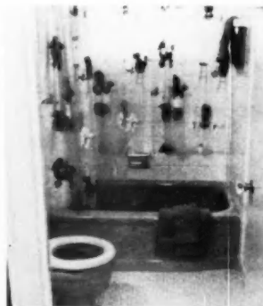
CLAY TILE floor and wainscoting in the bath are standard in all houses
