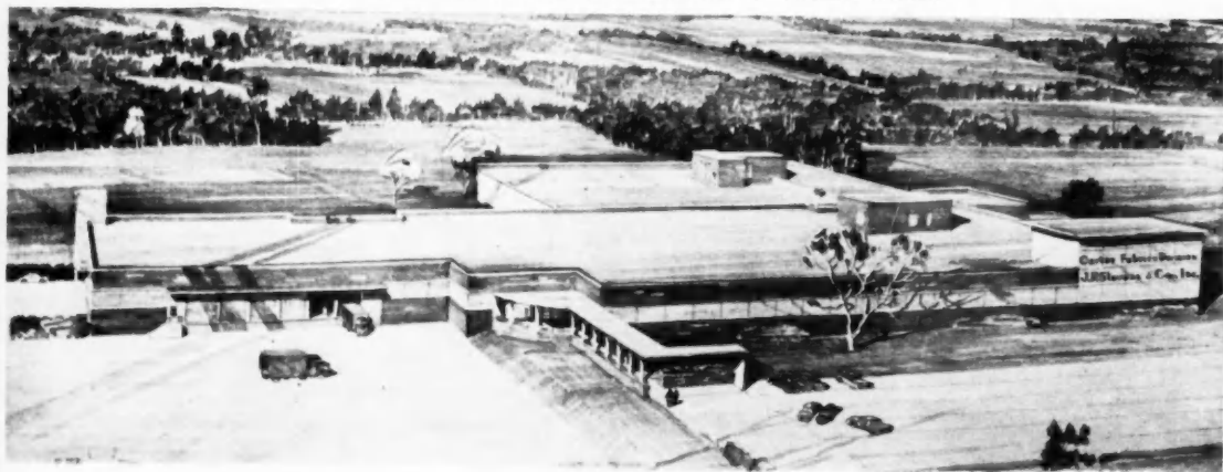
Carter Fabrics Division plant of J. P. Stevens & Co., Inc. at Wallace, North Carolina, a completely modular structure designed by Charles C. Hartmann, A.I.A.
