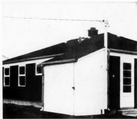
STORAGE ROOM at rear of house included in the 1952 model. It is designed to accommodate large items
