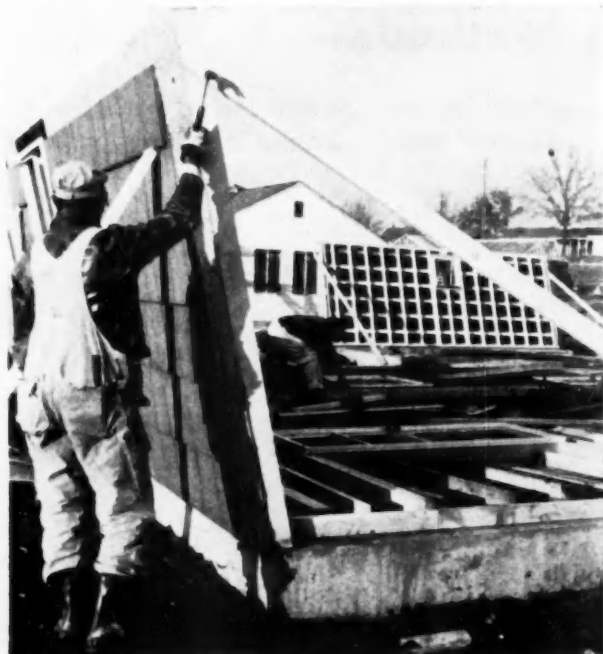
COMPLETE WALL was built in the horizontal position and raised
