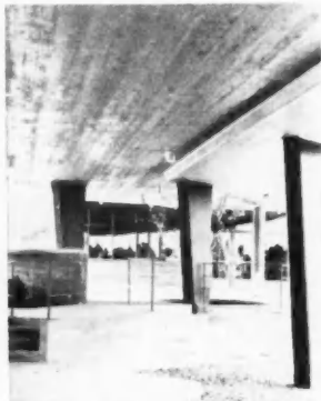
CLOSE-UP of canopied main entrance shows its interesting construction details
