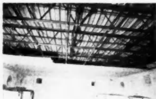
SHOWN HERE is construction of gypsum lath-lightweight gypsum plaster fireproofing for fire tests conducted at the National Bureau
