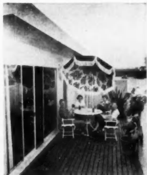
SUN DECK adjoining the new director's room built on the roof of old bank building
