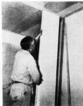
PARTITIONS are laminated T & G fiber-board placed in quarter round channels
