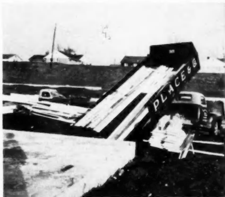
PRECUT and prefabricated units are delivered to the site. All members are marked to speed the building operation
