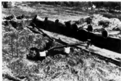
PENCIL ROD runs tie the beam together. The form used for this foundation is a 18-inch highway curb unit
