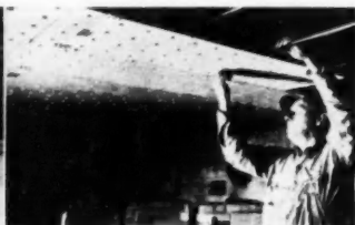
SHOWN HERE is construction of gypsum lath-lightweight gypsum plaster fireproofing for fire tests conducted at the National Bureau
