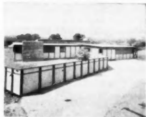
WALLS AND ROOF of this home are vermiculite asbestos; plastic is used throughout
