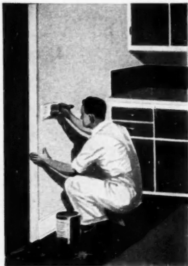
PAINTING INTERIOR WALLS - WOODWORK
