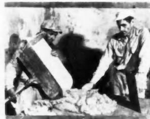
PLASTERERS' magnesium hod and hawk are also characterized by light weight
