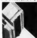
1/2" outside sheathing and 3/4" dry-wall applied over 1/2" insulation board on 2x4's, cut-off rib on blind stop.
