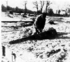
FORM that held the vapor barrier, insulation, and ducts is removed
