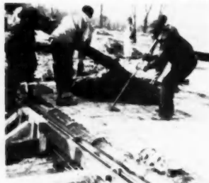
CONCRETE FOR FLOOR. beam, and stoops is poured at one time
