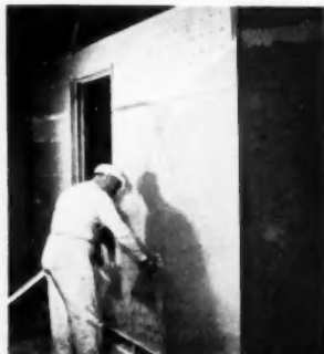
BROWN COAT goes over scratch coat
