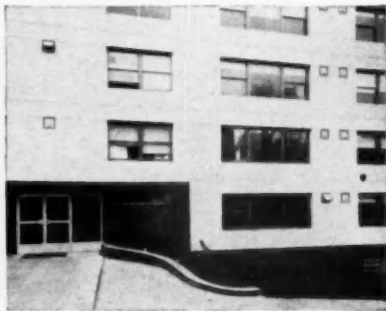
Illustrated at the right is the $1,200,000 Queensborough Apartments of Seattle, Washington . . . equipped with NuTone. (Notice the NuTone Ventilating Fan heads for each apartment.)
