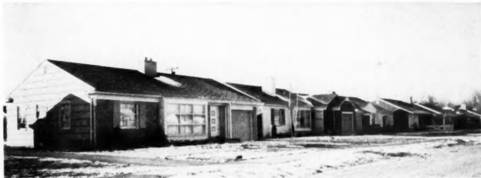
TYPICAL STREET of Lockwood homes showing good exterior variations gained from using 6 plans with 4 elevations for each plan
