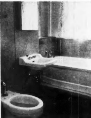
BATH fixtures are movable. Tub is on casters. Core walls are asbestos cement
