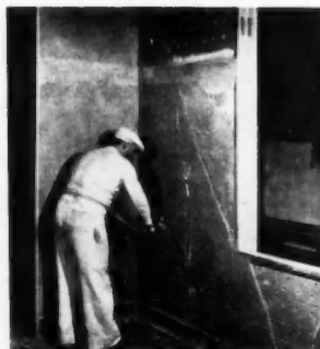
TWO-COAT application; scratch coat omitted
