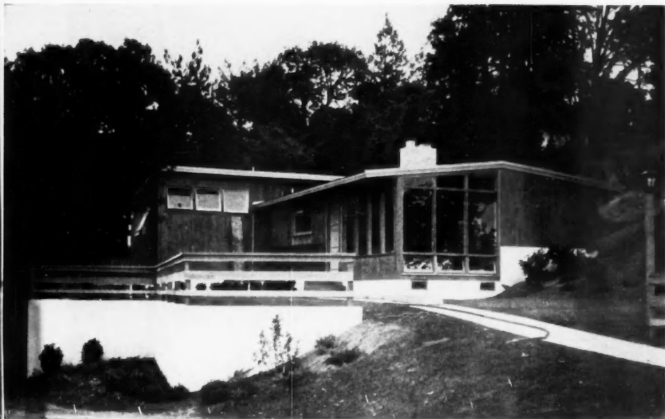
THIS HOUSE with its interesting grouping of levels and retaining wall nestles snugly into the side of hill
