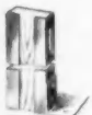
Above: Wood filler strips in metal frame allow plaster base, stops and trim to be nailed or screwed in usual manner.
