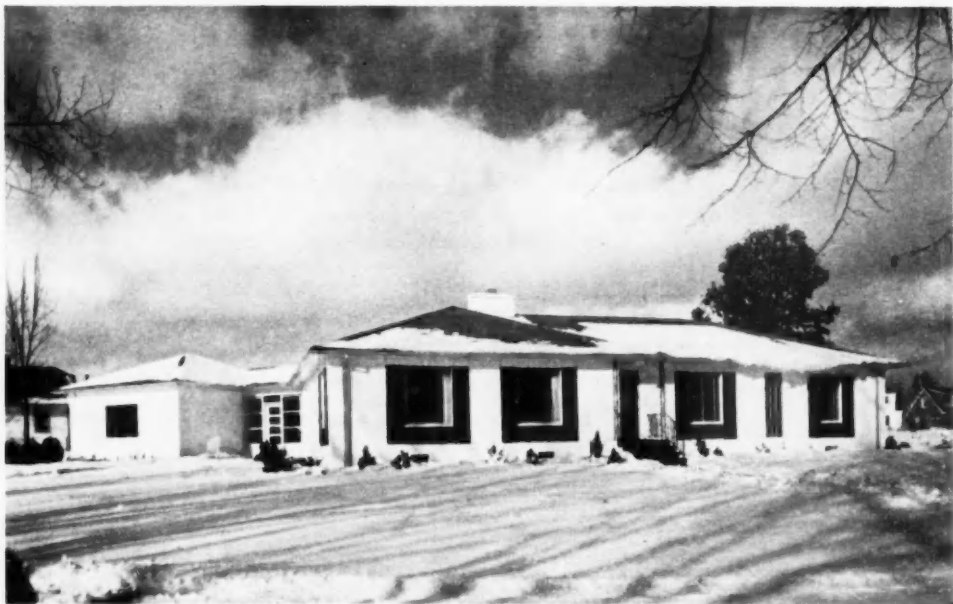
WHITE-PAINTED walls with red asbestos cement roof and red shutters spark exterior of this Elkhart, Indiana, tilt-up concrete home
