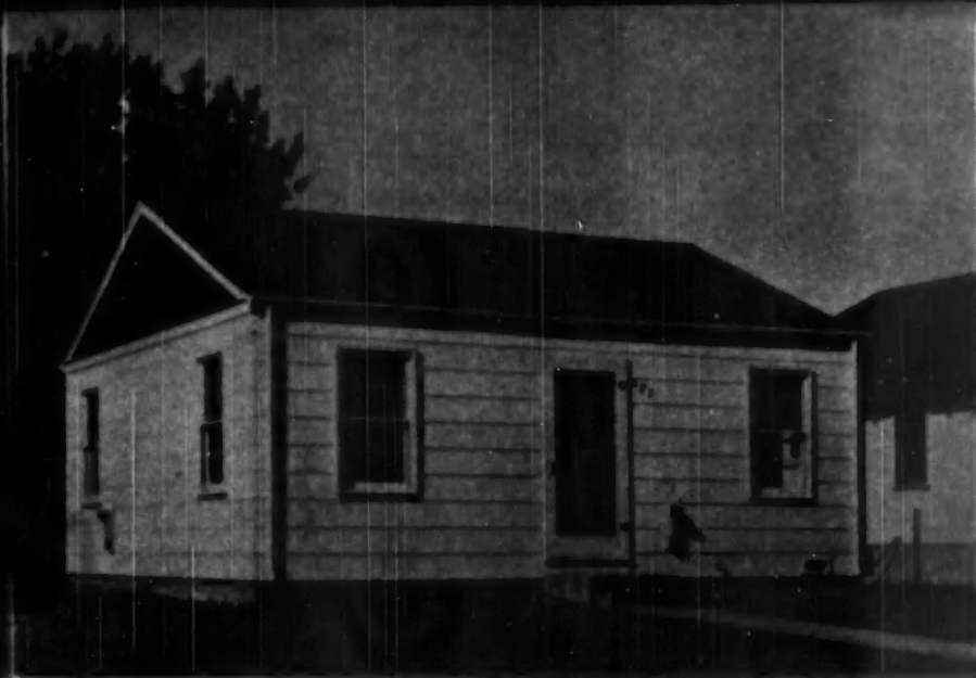
FRAN-MINI house of D. C. Burns Realty and Trust Co. contains 591 square feet of floor space. Two wall-type floor furnaces with 17,000 B.T.U. capacity each provide heat. Siding, asbestos shingles.
