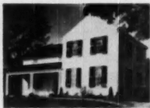
2. CHIEF improvements included raising roof of wing, applying fresh white siding and a new roof of green asphalt shingles, and trimming overhang at the rakes and eaves.
