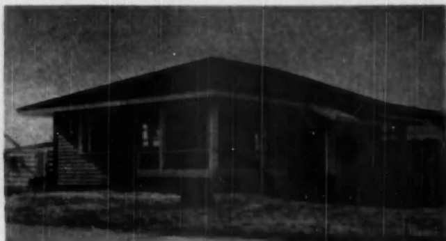
THIS house with its unique corner window won National Association of Home Builders Best place regional award. Steel casements at side of stationary units furnish ventilation
