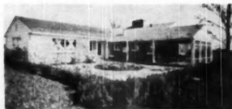
TERRACE affords privacy; is easily reached from kitchen, porch, bedrooms. Overhang protects passage from house to garage
