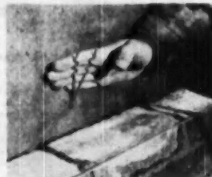
TIE is bent over to required angle as the brick wall is brought to proper level
