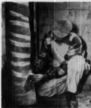
NEW METHOD of covering roof drain pipes with Fiberglas Aerocor insulation, being used at St. Vincent's Hospital, Toledo, Ohio.
