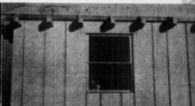
FARGET or cement grout is used to finish bottom of panels, left. Wood roof framing members are used with panels, right. Lintel and different width panels for lower part of window are provided. Modern-Crete is nailable aggregate and may be easily sawed
