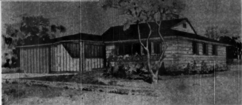
REAR yard living is emphasized in this medium-size, all-frame house. Splayed rake at gable ends adds interest
