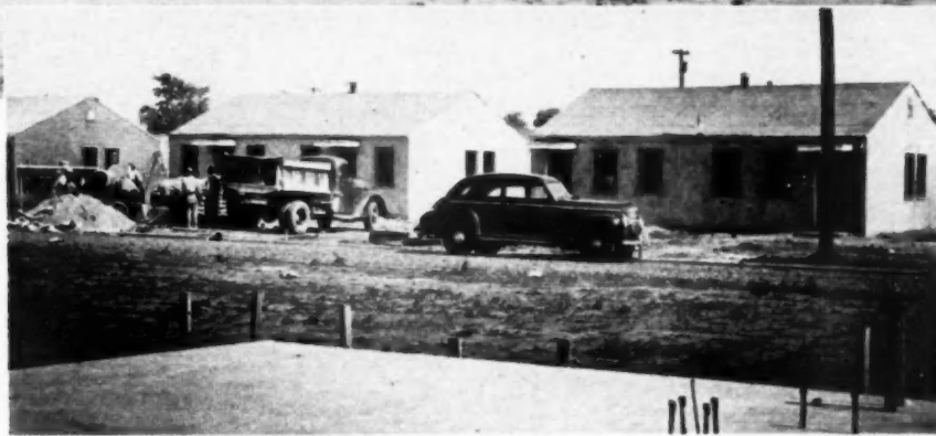
A STREET of completed homes shown above. Variations in the houses occur in the color of stucco and roof shingles. Construction of concrete mat in foreground. Plumbing assembly is in a direct line with fixtures of each unit placed back-to-back
