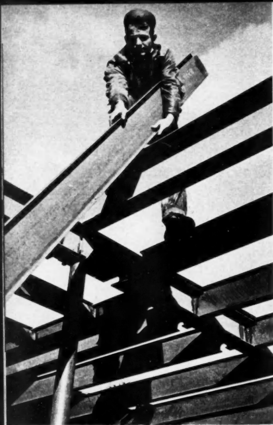
JUNIOR I-beams hold lath and plaster by means of furring clips, as shown below
