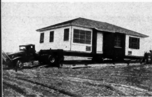
HOUSE is lowered by jacks to foundation
