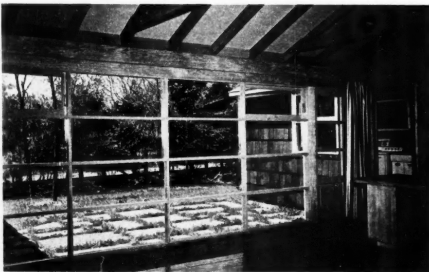
INTERIOR of living room in $18,000 Sun Ranch home looking through large window onto terrace. Note open ceiling with exposed rafters. Walls are gypsum board
