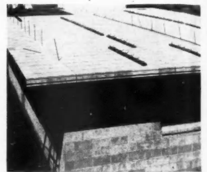
STRESTCRETE roof on Sacramento home
