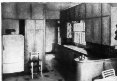
Cabinets, built-ins, storage-walls, sliding doors—whether shop-fabricated, built on-the-job, or constructed by the home owner—all can utilize stock plywood panel sizes.
