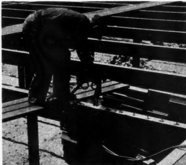
STUD welded fasteners are used to install metal roof deck of power plant building
