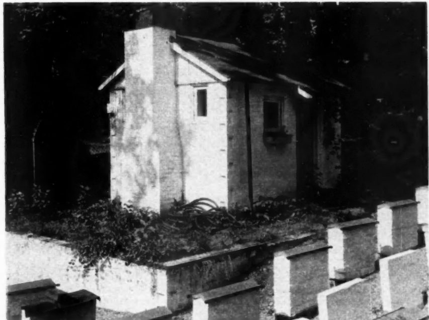
THIS cinder block test house finished with two coats of grout and two coats of rubber base paint showed no evidence of leakage after six years of service. Tests conducted by National Bureau of Standards were also made upon cinder block retaining wall
