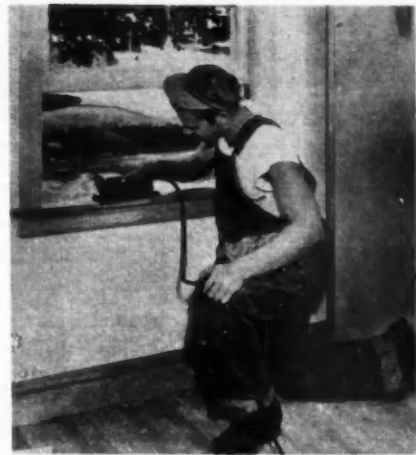
LIGHT sanding of trim between finish coats
