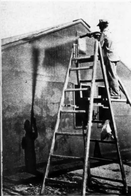
JETCRETE operator applying final stucco over base of Steeltex reinforcing mesh
