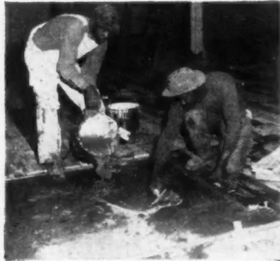
WORKMEN apply adhesive for cementing sub-base planking to concrete slab
