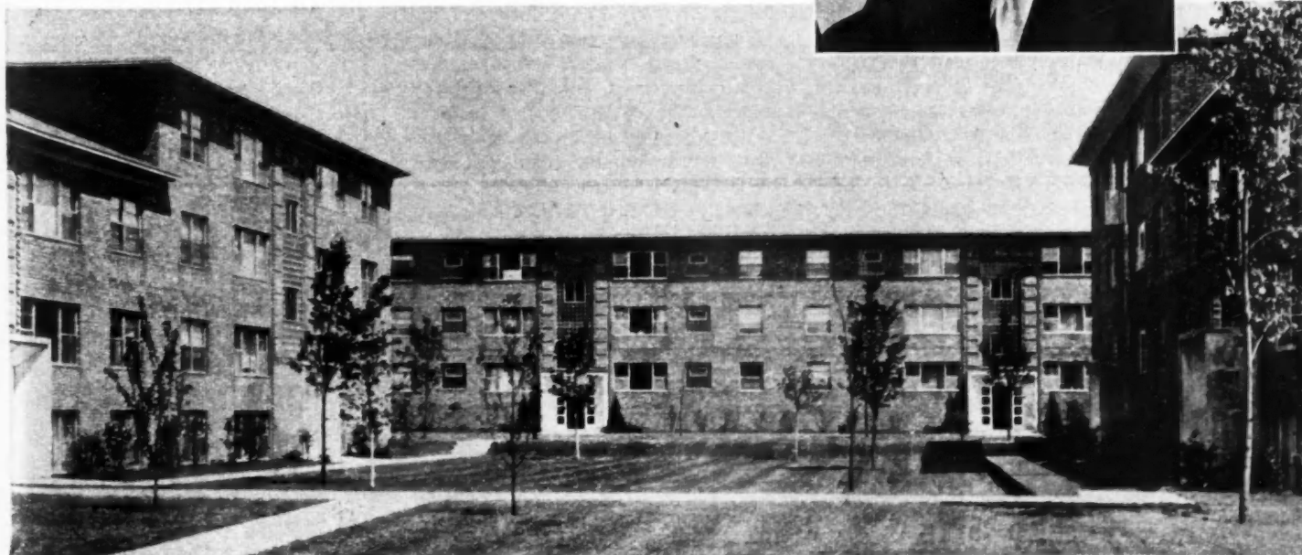
ONE of the five courts around which the 19 buildings are located. Arrangement permits light and air on both sides of each apartment
