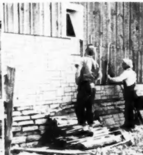
SIDING arrives on the job neatly packaged and easy to handle. Rotten boards and timbers were replaced to give firm nailing
