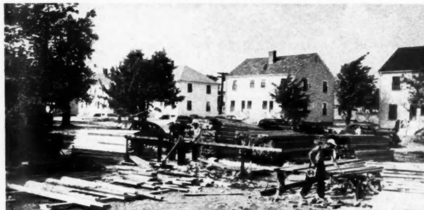
A SITE precutting operation cut construction costs, sped work
