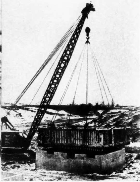
A SYSTEM devised by manufacturer enables builder to strip entire foundation, inside and outside forms, in one operation. This is an example of how improved forms speed up work. These forms are steel
