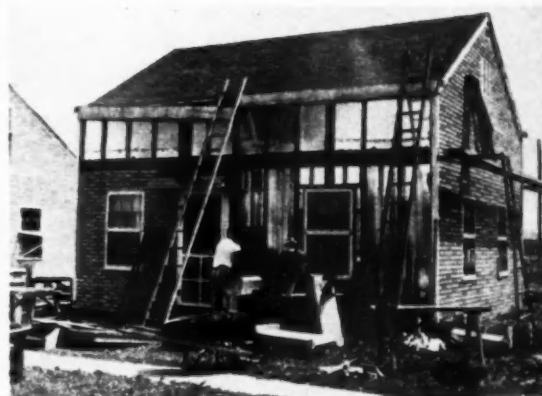
SINGLE-FAMILY two-story temporary units were prefabricated in university armory
