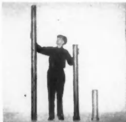
8-foot lengths reduce number of joints to be made.
