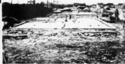
AFTER copper coils for radiant heat are laid, ready-mix concrete is delivered to site for floor slab. Framing begins on slab. Plates, studs, joists, rafters are precut
