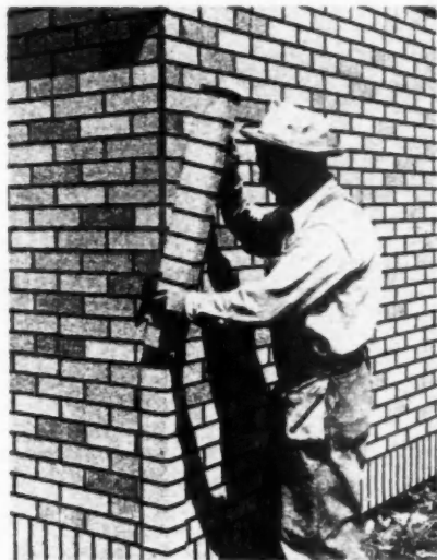
CARPENTER Miller applies corner trim to utility shed. Insulated siding is easily cut with a roofer's or fibre board knife from both the front and the back sides
