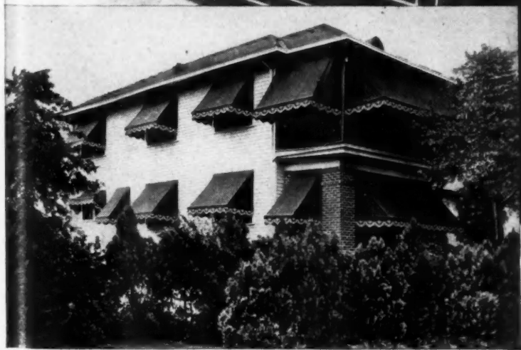
TEXAS. "We keep our home cool all summer and warm all winter with Servel All-Year Air Conditioning," comments Mr. Nelson Waggener, 7700 Mockingbird Lane, Dallas.
