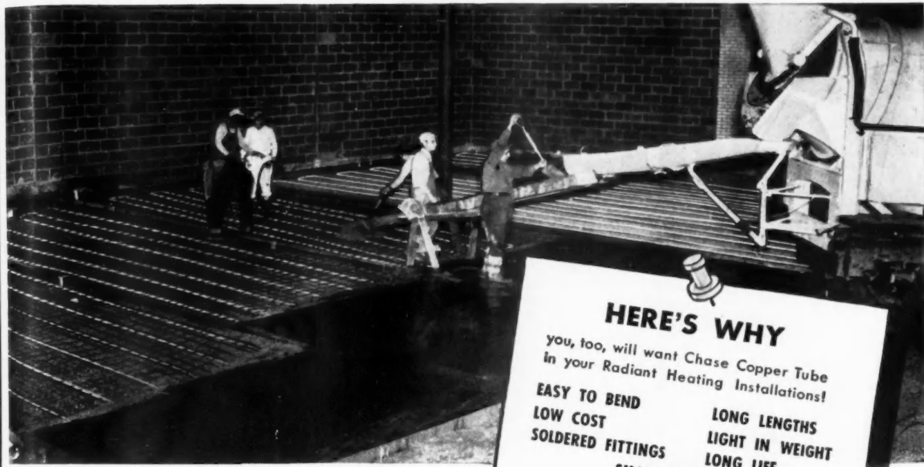
Pouring concrete over 12,000 feet of Chase Copper Tube. Installation also included 5500 feet for office ceiling and 1200 feet for sidewalk and drive snow removal. Architect: Charles A. Maguire & Associates, Providence, R. I. Building Contractor: A. F. Smiley Construction Co., Pawtucket, R. I. Heating Contractor: J. F. Higgins Heating Co., Providence, R. I.
