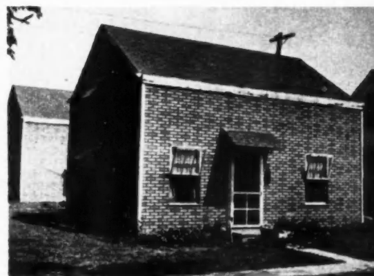
ARRANGEMENT of rooms in units. TEMPORARY exterior paper board covering with 960 square feet of floor area was replaced with fibre glass brick siding
