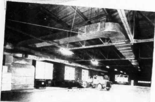
Interior view of one portion of Clare County Road Commission Garage.
