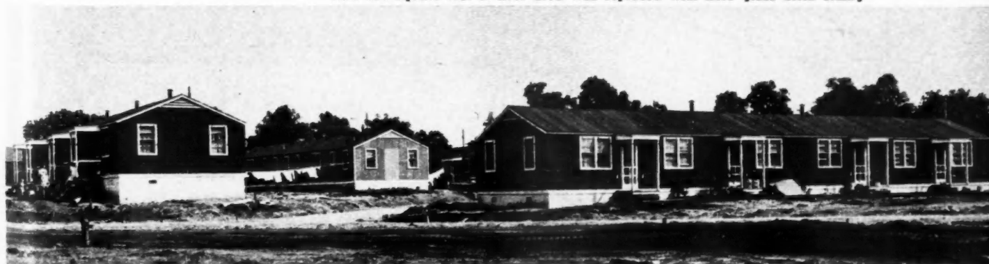
APARTMENT barracks for married veterans with children, which were moved from an army camp and re-erected at Purdue
