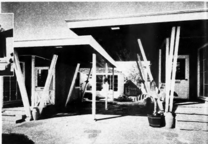
"BEFORE" and "after" buildings had been converted into modern business rentals
