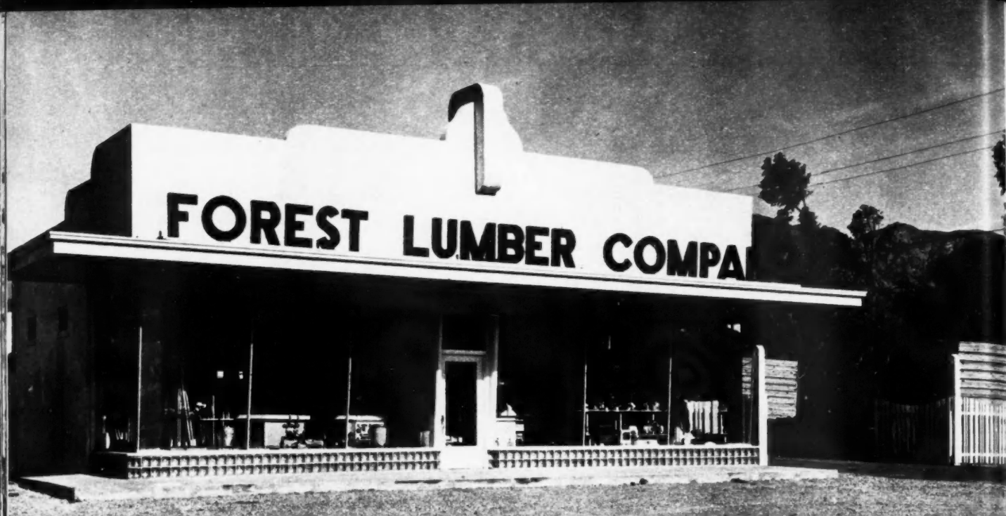
THE name, "Forest Lumber Company," is in black-faced letters, 24 inches high, illuminated at night
