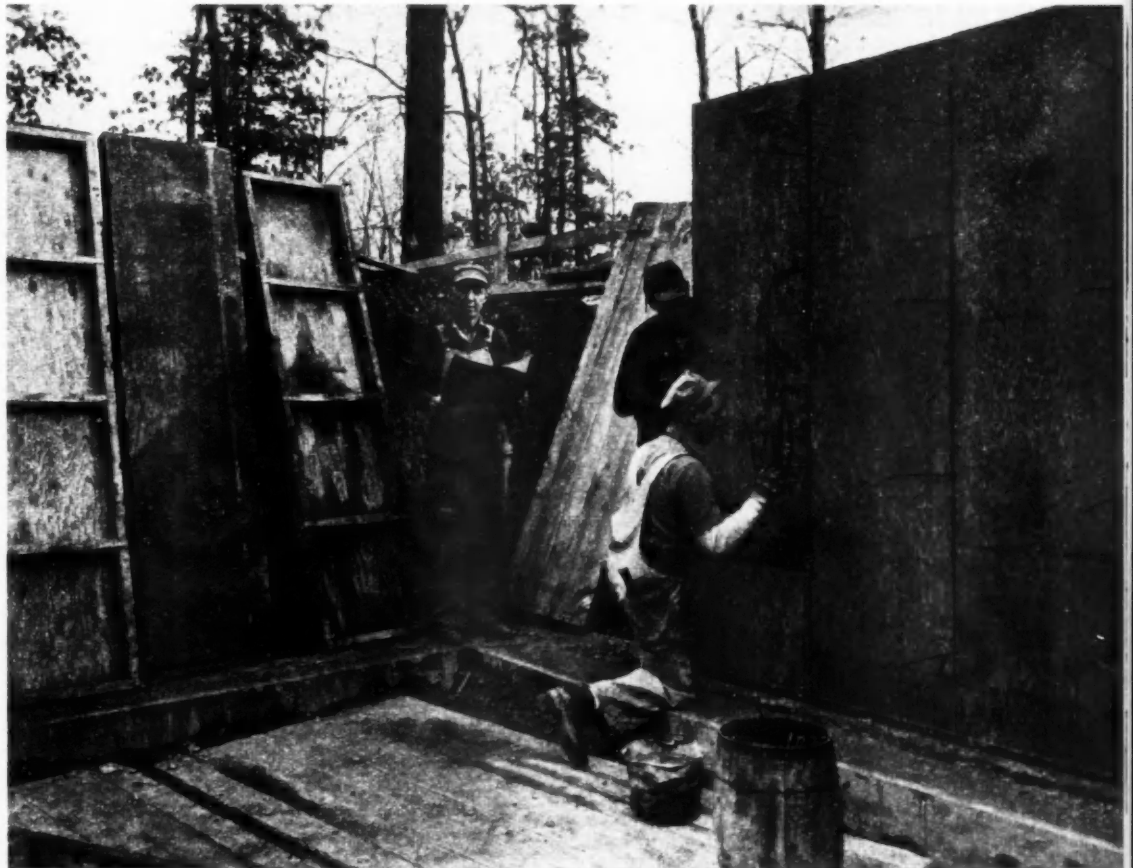
TIE RODS for these forms are anchored from side. When forms are taken down, they may be lifted straight up without disengaging ties. This is another example of what manufacturers are doing to provide simplified hardware for faster handling
