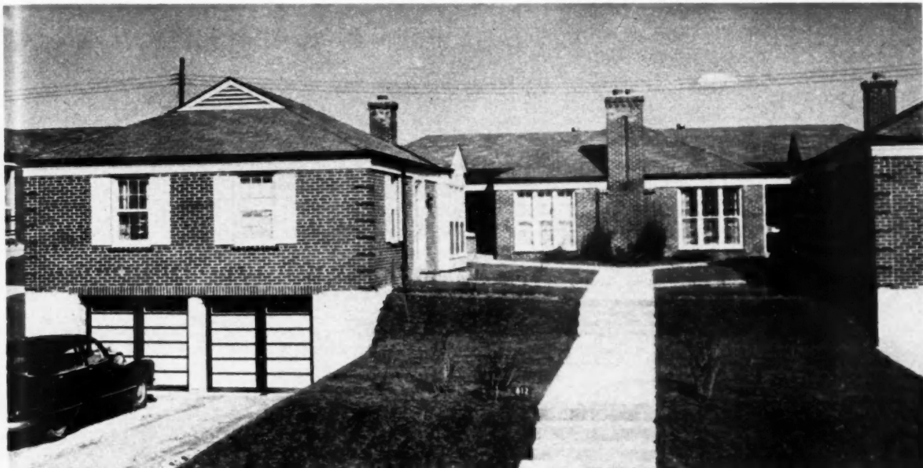
BASEMENT GARAGES in two front apartment units house four cars and heating units.
