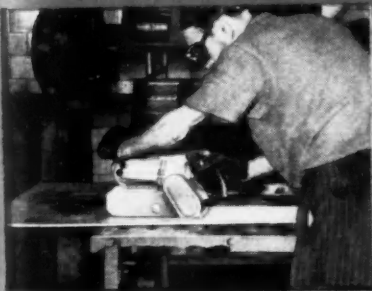
SKIL Belt Sander sands flat or contoured surfaces of all materials . . . wood, metals, stone, tile, concrete and compositions.
