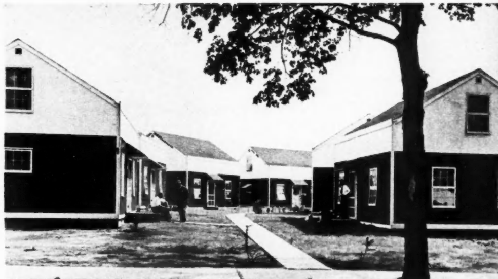
SINGLE-FAMILY two-story temporary units were prefabricated in university armory
