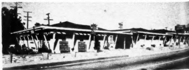
TILTED posts supporting overhangs are attention-getting feature. Method of attaching posts to overhangs are shown in drawing detail. Flagstone wall is an added embellishment
