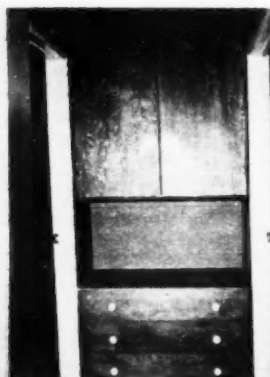
BATHROOM has walls of linoleum-covered plywood, asphalt tile floor. Cabinets and built-in drawers serve as linen closet between bedroom doors, center. Notice shelf space
