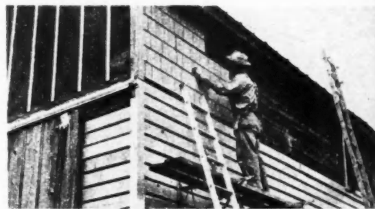
CARPENTER Miller applies corner trim to utility shed. Insulated siding is easily cut with a roofer's or fibre board knife from both the front and the back sides
