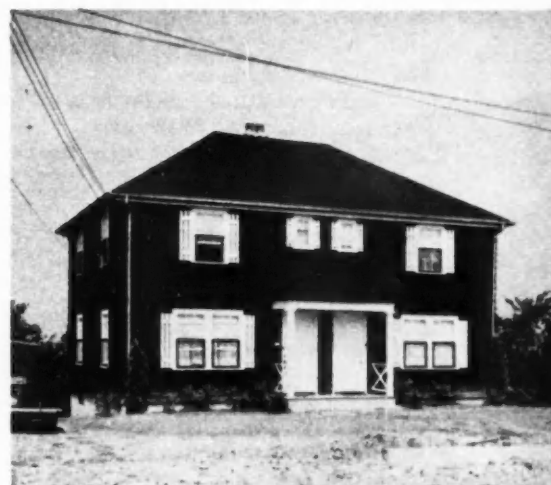
HIP ROOF variation of same floor plan avoids monotonous appearance in project
