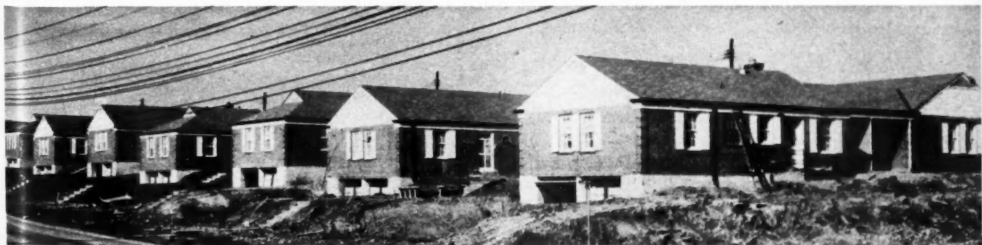
APARTMENT units in this Clayton, Mo., project are on 100 x 135 foot lots
