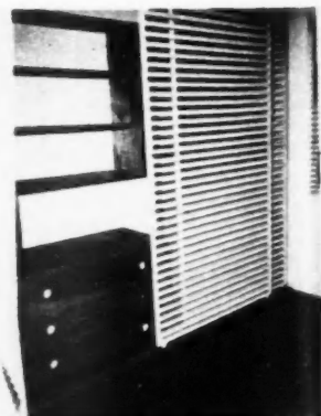
BATHROOM has walls of linoleum-covered plywood, asphalt tile floor. Cabinets and built-in drawers serve as linen closet between bedroom doors, center. Notice shelf space
