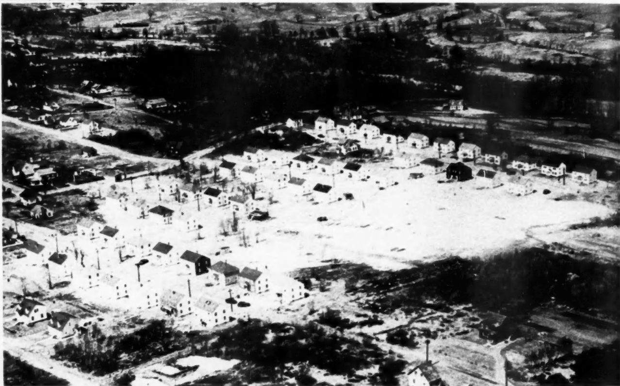
AERIAL view shows completed homes, occupied within a year after trust was formed. Foundations are of 12-inch concrete
