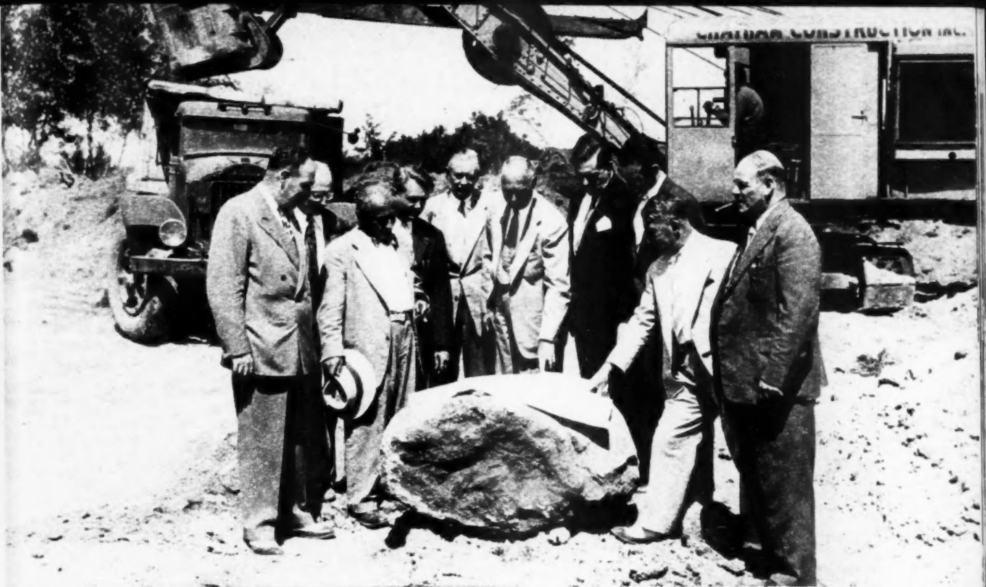
BUILDERS. finance men and public officials gathered with little fanfare for ground breaking ceremonies in mid-1947.
