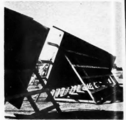
ABOVE: EASELS on which concrete forms are completely assembled
