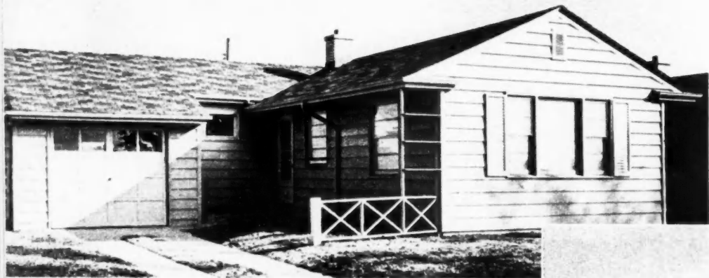
TWO HOUSES from the same basic floor plan built by Forman Construction Co., priced to sell for about $13,800. Exterior of the one below is finished with waterproof striated plywood. Interiors of both houses are dry wall with gypsum board joints taped in regular manner
