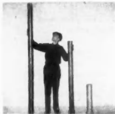
8-foot lengths reduce number of joints to be made.
