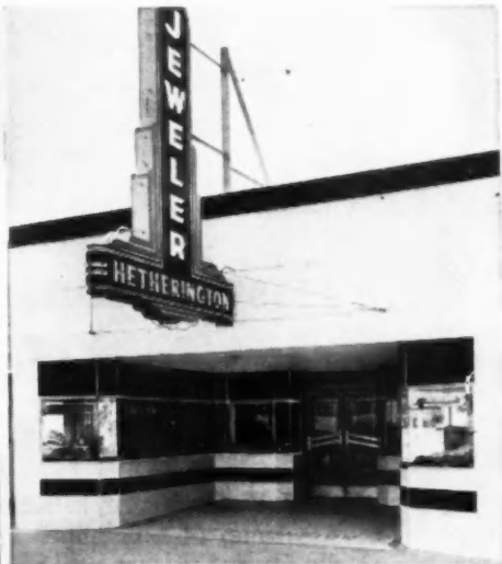
TEXAS. "I am well pleased with my Servel unit," states J. W. Hetherington, jeweler, of Texas City, Texas. "People prefer to shop where the temperature is normal and the air pure and clean."
