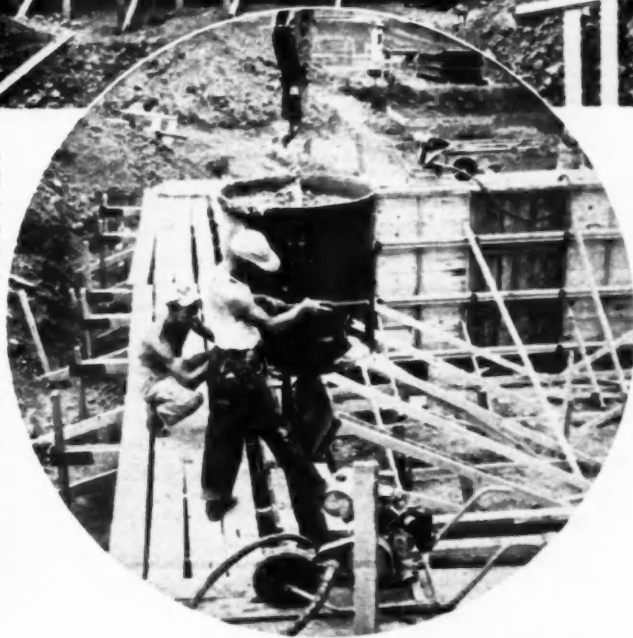
CLOSE UP view of bucket showing concrete released into forms. Plot plan below
