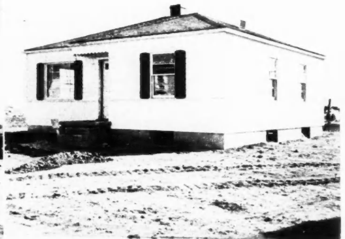
ANOTHER version of the typical one-story house, employing a skirting of bonded plywood on the house exterior
