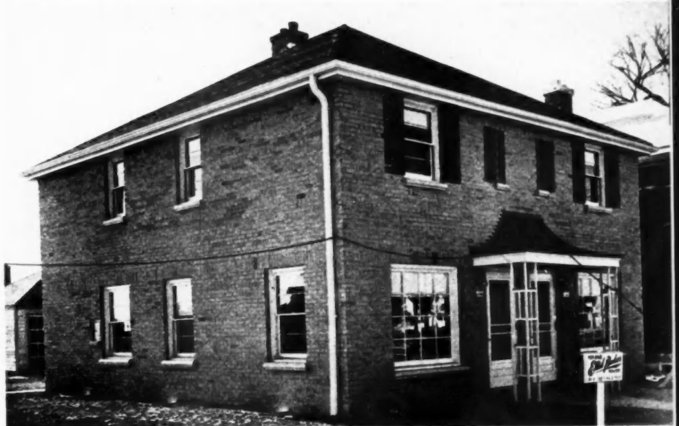
THE ONLY multi-family structure in the "Parade of Homes" is this 2-story, 2-family brick veneer built by James R. Baer, at a cost per unit under the $12,000 ceiling
