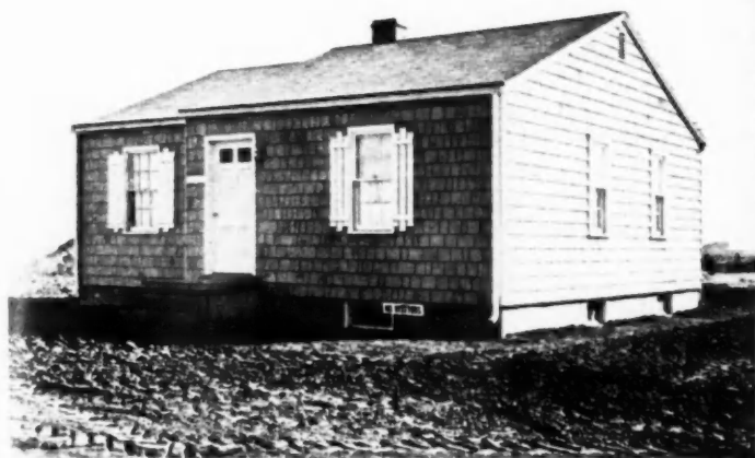
A SLIGHT variation to the typical two-bedroom plan is used in this house. Wood shingles used as exterior facing
