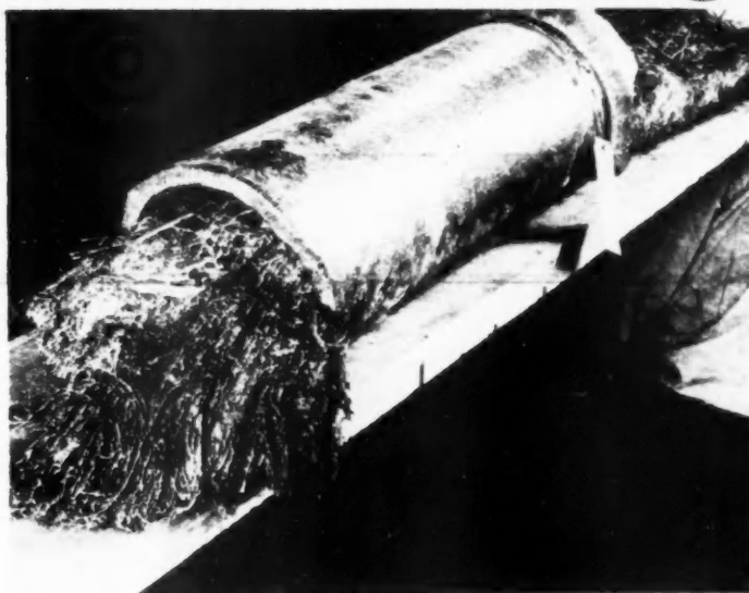
EXAMPLE shows how cracked cement joints in sewer attract roots
