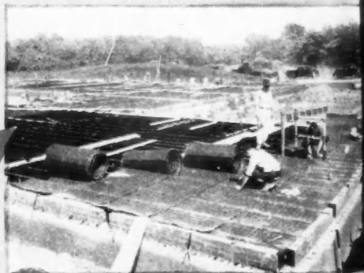
2 Fibre-backed steel mesh is nailed directly to Stran-Steel joists.
