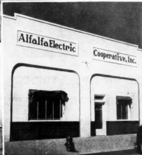
OKLAHOMA. "The Servel installation has contributed much toward the efficiency of our staff," reports Clarence R. Green, Manager of the Alfalfa Electric Cooperative, Inc., of Cherokee, Okla.
