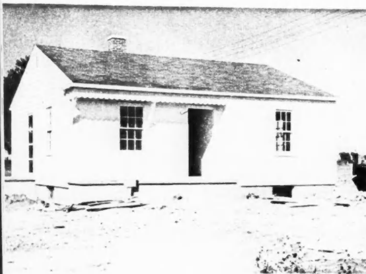
TWO-BEDROOM one-story house with facing of bevelled siding, typical of this mass housing project, is pictured above
