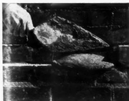
Method 3. A full trowel of mortar should be thrown on the wall.
