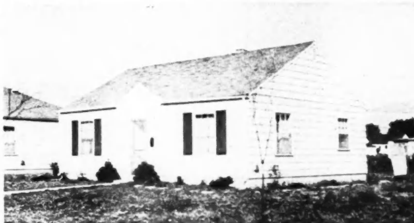
TWO-BEDROOM houses, which could be sold for $6,750, are rented for $50 a month. Maintenance of interiors is done by tenant, exteriors by home builder
