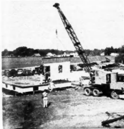
LARGE crane with special hook rigging placing wall section in position
