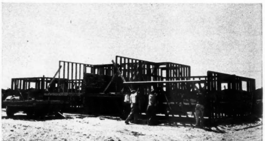
HERE EXTERIOR wall sections are put in place. Sheathing crew will come on next
