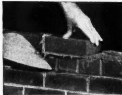
So there will be more than enough mortar to fill the joint completely when the next brick is pushed into place.
