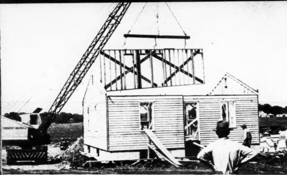
AFTER side and end walls are placed in position on house, then interior partitions, which are also built on a "jig", are installed. Sections are tightly secured
