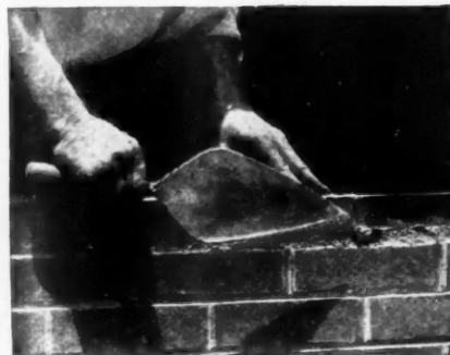
Method 2. A dab of mortar should be spotted on the corner of the brick already in place.
