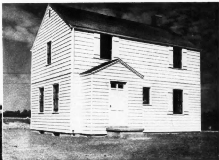
A TYPICAL two-bedroom, two-story house. A combination of wood shingles and bevelled siding used on the exterior
