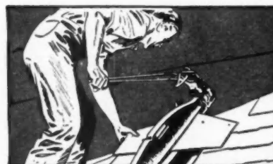
6. CUTTER SPEEDS APPLICATION —When shingles must be cut to fit around valleys, dormers, along the rake, etc., a shingle cutter does the job easily, quickly—right on the roof.
