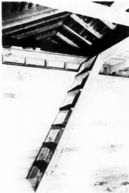
THIS access stair, built in garage, to storage space in attic is a popular feature.
