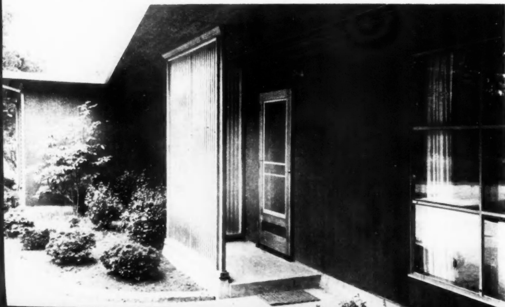
DETAIL view of roof soffit with continuous screened strip for ventilating this area.
