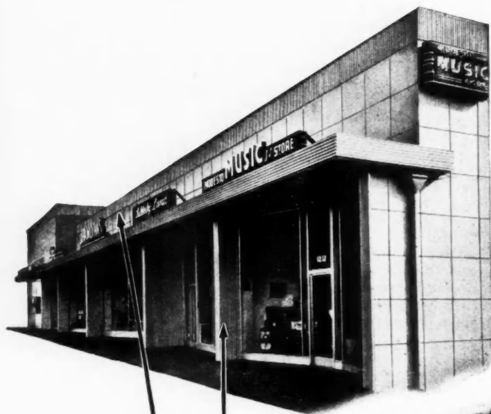
This modern shopping center in Modesto, California, makes use of Zourite as a facing for the walls which separate the stores and as a decorative covering for the cornice.
