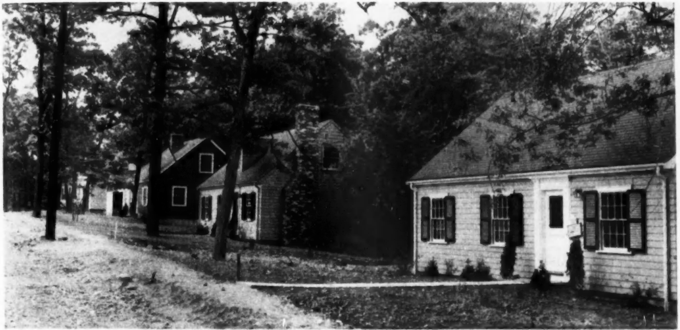
HOMES built primarily for veterans are also placed in the midst of all the natural beauties that surround Oak Hill Village.
