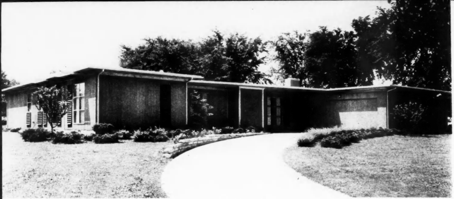
LOW sweeping, horizontal lines with just enough vertical emphasis in the windows and louvers produce a pleasing exterior.
