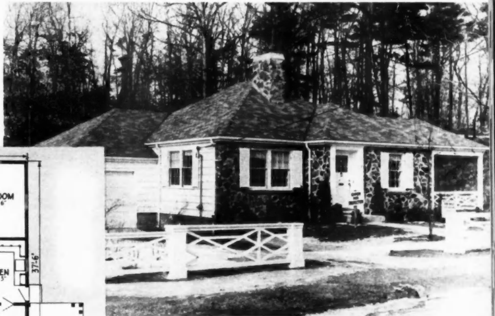
NATIVE stone excavated on site was used by builder in facing the front wall of this attractive one-story, five room design.
