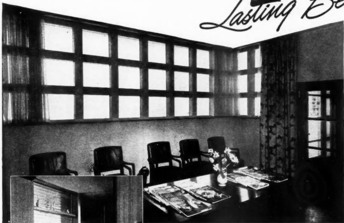
Thermopane units made with Flutex in crossed pattern achieve privacy plus cheerful light. Office of Dr. Carl T. Moore, Kansas City, Mo. Architects: Carroll & Dean.
