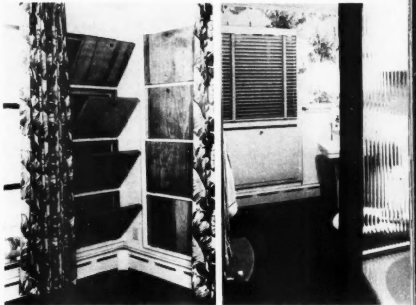
DETAIL of panels in back of louvres.
