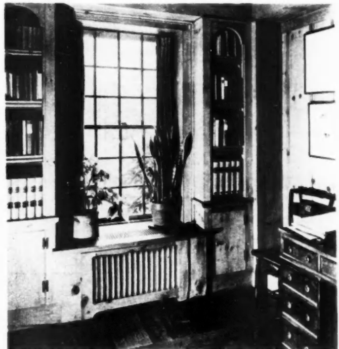
PINE paneling which makes the walls of this room so attractive was also used to build a grille around hot water radiator.
