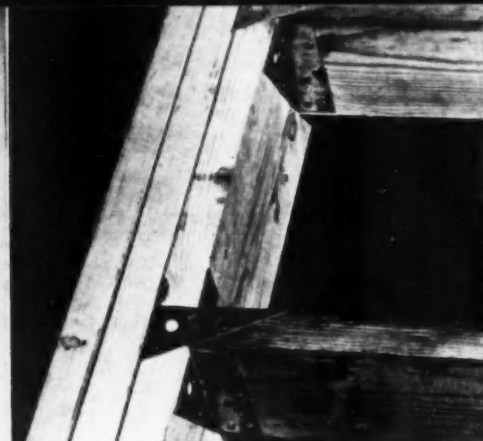
C and B—joist to beam or header.
