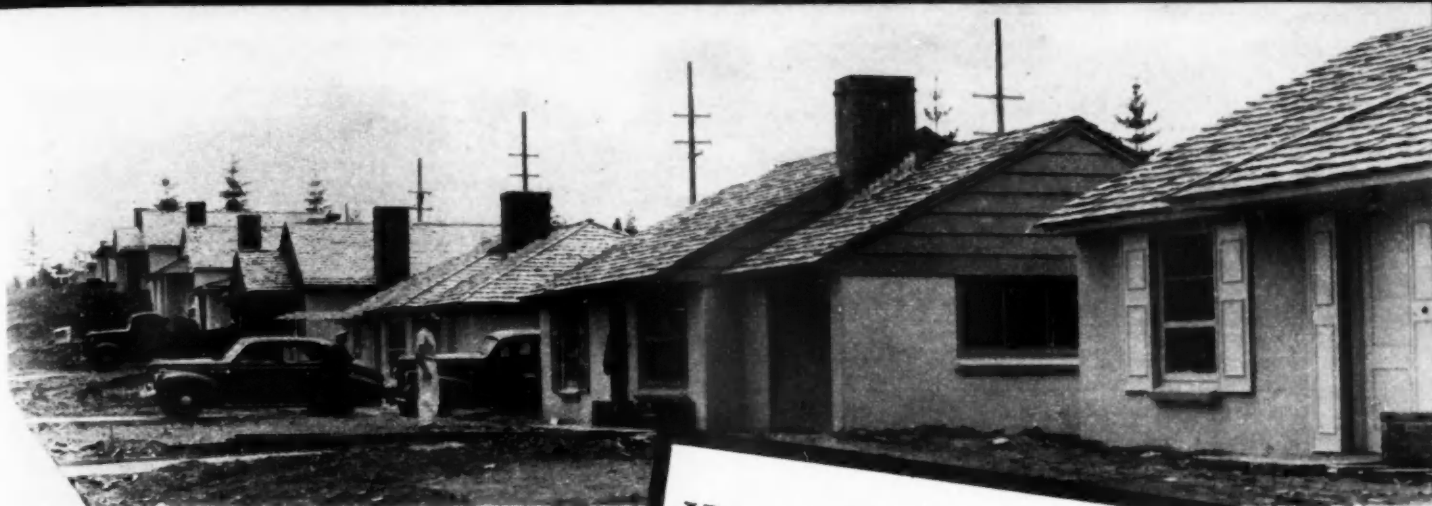
MINIMUM lot size for these fully-equipped radiant heated two and three bedroom concrete block houses is 65x175 feet.
