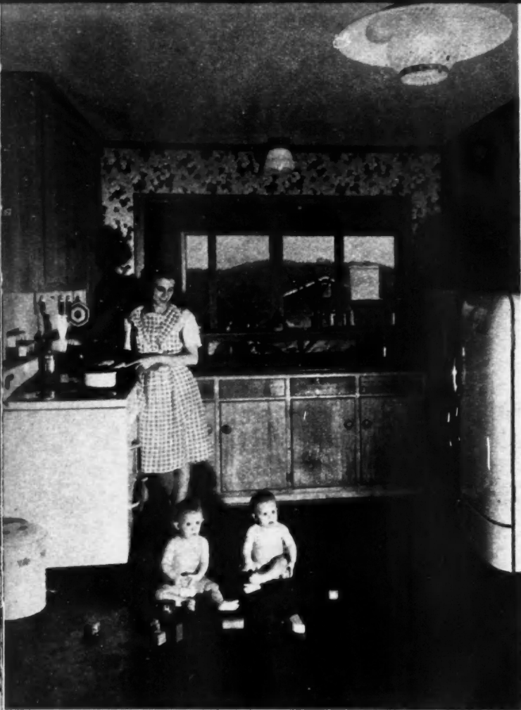
ELECTRIFIED ceilings in this house in Knoxville, Tenn., make the rooms comfortable in winter regardless of outdoor temperatures.
