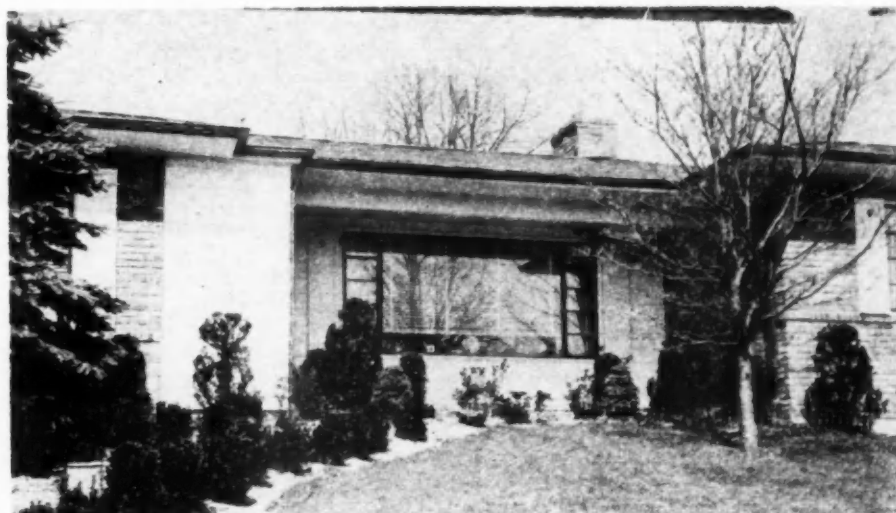
DETAIL view of portion of street elevation. Frame vestibule extension adds interest.
