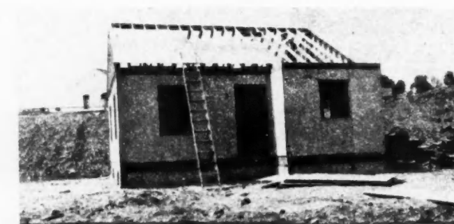
2:25 P.M.—Sheathing already covers part of structure.
