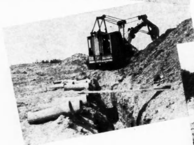
HEAVY earth-moving equipment, all owned by the contractor, leveled ground, excavated for footings and utilities, preparatory to above ground operations.
