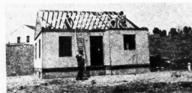
2:15 P.M.—Last section of roof framing is put in place.
