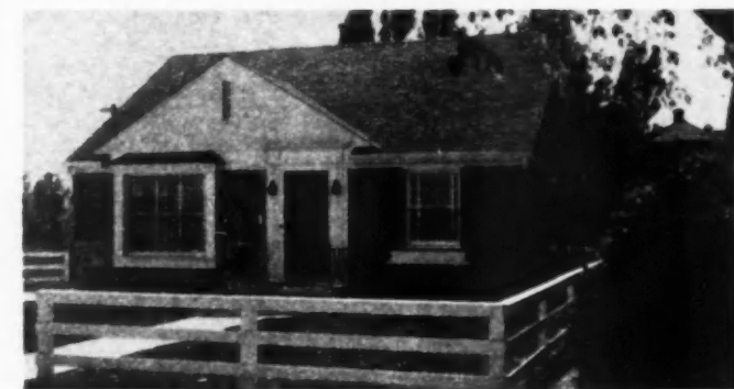
FRONT view of Ebenreiter demonstration home at time of open house.
