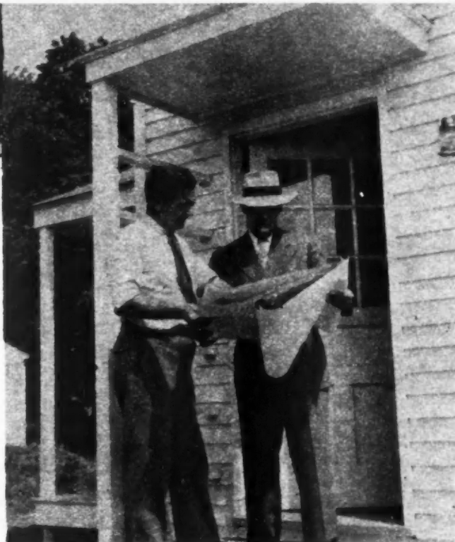
RIGHT: Donald L. Walsh, president of Bay State Precision Builders, Inc., (right) checks plans with Construction Superintendent William H. Ross.
