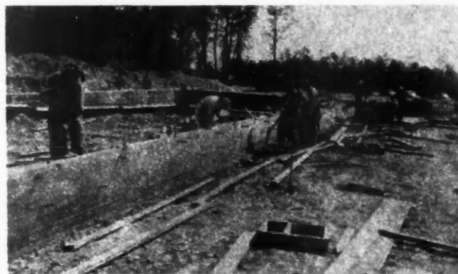
WORKMEN strip concrete forms and clean up foundation walls.
