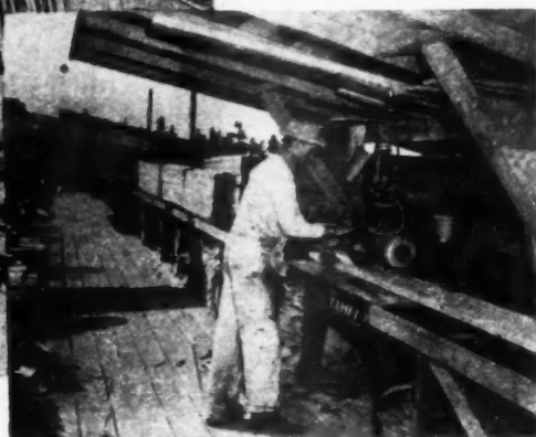
Mass production building efficiency and economy are being utilized on this large multi-family housing project. Framing lumber is pre-cut and then assembled on jigs in workshops located on the project site.
