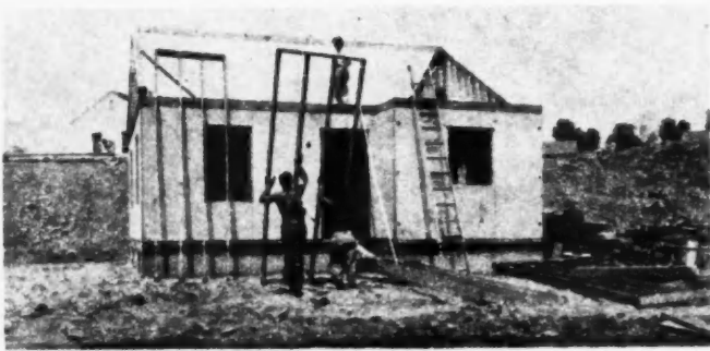
1:30 P.M.—Roof sections are being hoisted into place.
