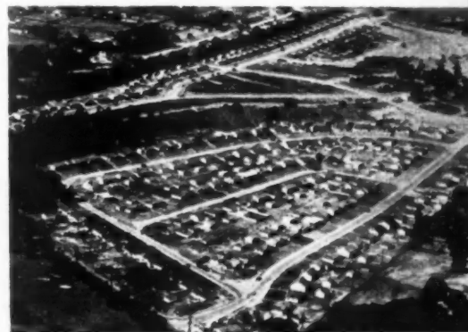
AIR VIEW of Kenneth P. Schmidt's tract development, Rancho La Canada, in La Canada.
