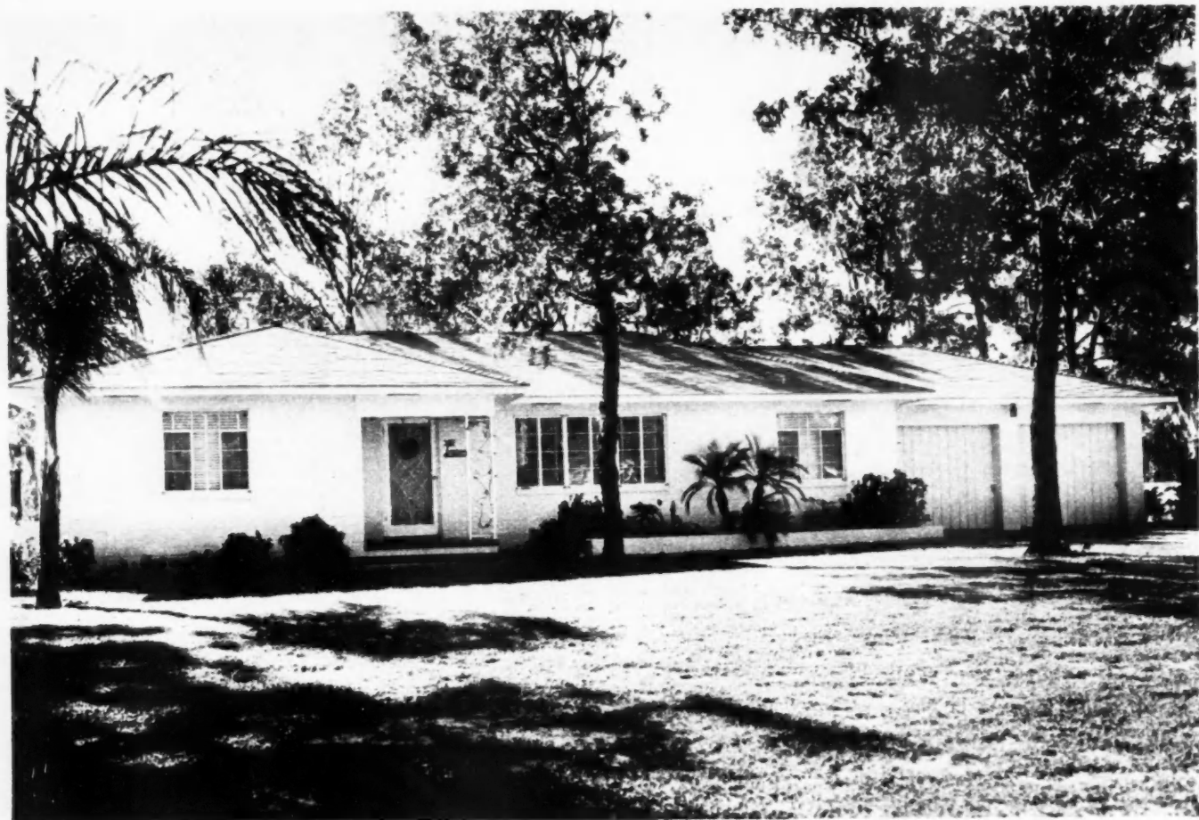
THIS beautiful ranch-type concrete block house was built by Robert Rise, home builder in St. Petersburg, Florida.
