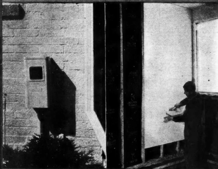
AT LEFT is one of the meters used in research on the Sloan house. Photograph at right shows workman nailing Sheetrock to conventional wood studding.
