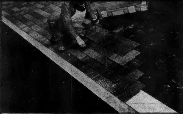
ABOVE the floor line the Sloan all-sealed house is of conventional construction. Here workmen are shown, when the house was being built, laying USG asphalt shingles over USG roof boards nailed to wood rafters.
