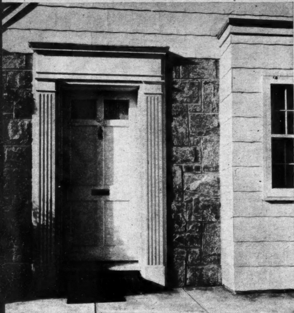
ABOVE is shown the detail of front entrance of house below. A combination of materials including native stone, brick and asbestos shingles has been successfully employed.
