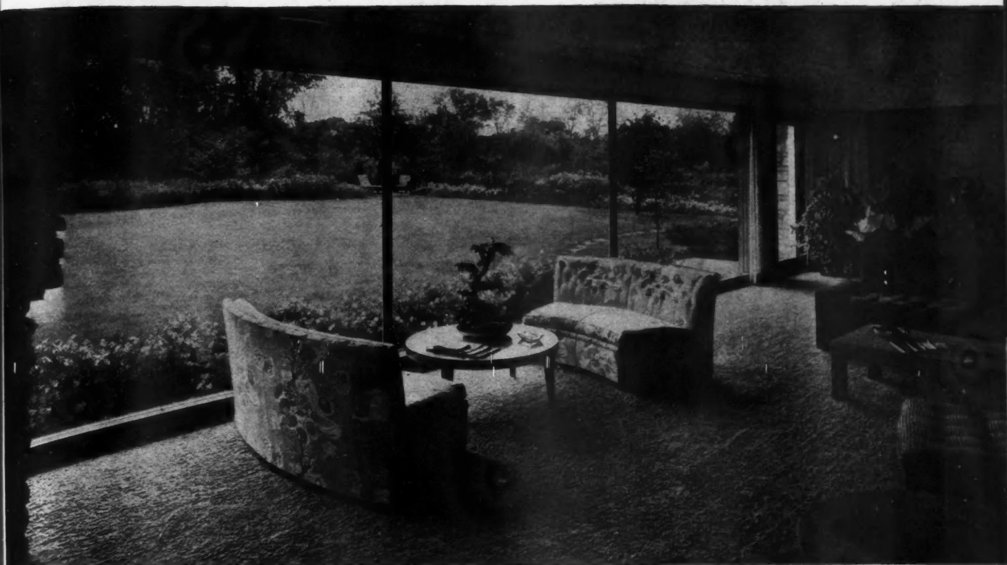
THREE Thermopane windows seven feet high and nine feet long make a total glass area of 27 feet long and seven feet high on the south side of the living-dining room exposed to the sun during winter months.
