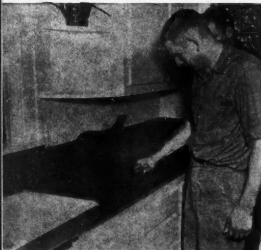
WORKMAN quickly and permanently bonds linoleum sink top with Miracle adhesive.
