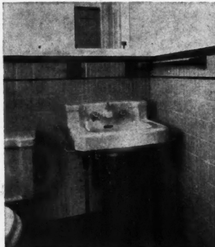
A COMMON application of Sparamics direct-adhesion tiling is shown in bathroom.
