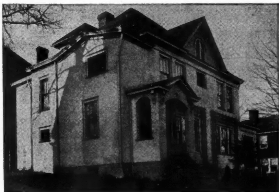
The above photograph shows the same stucco home after it received one heavy application of THOROSEAL, which, after being applied for one year, shows no leakage or dampness on the interior of the building.
