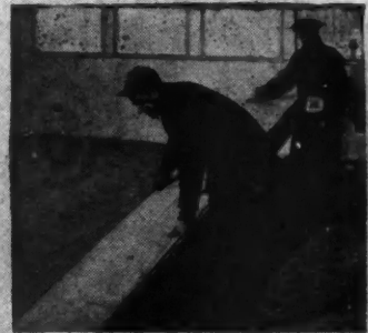
Fenestra Panels are quickly laid to provide an ideal subfloor.
