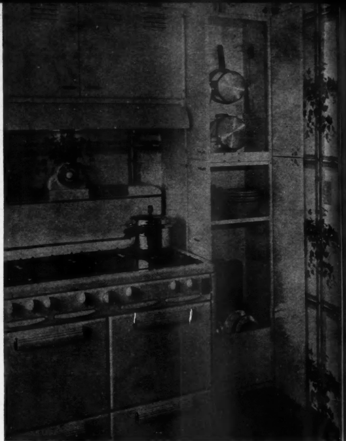
SERVEL air-control cabinets above kitchen range remove steam, cooking odors, etc. Blower starts when the hood is lifted.
