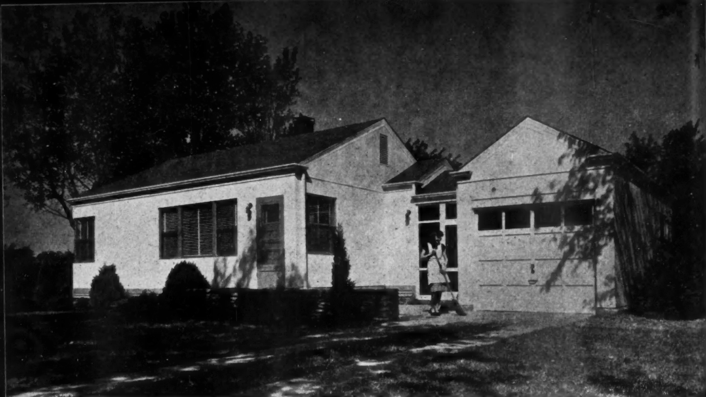
OVERALL dimensions of basic Butler two-bedroom aluminum house are 24 x 33 feet. Garage equipped with Ro-Way upward-acting door.
