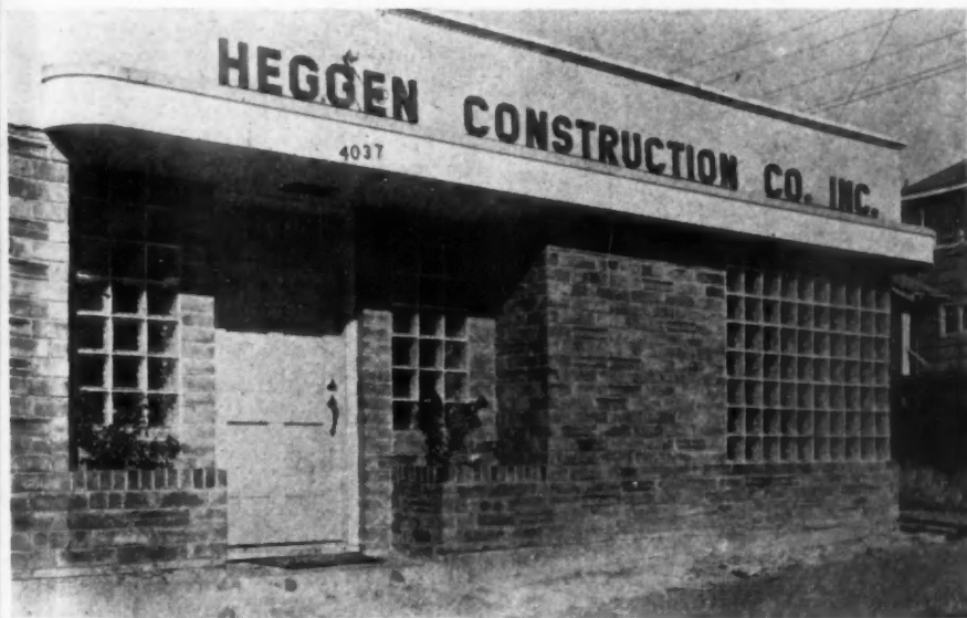
ENTRANCE view of Heggen brick veneer and glass block building, and floor plans, below.
