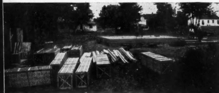
ALUMINUM panels and other house parts arrive on site in crates. BELOW: Exterior walls are in place, interior partitions being set.
