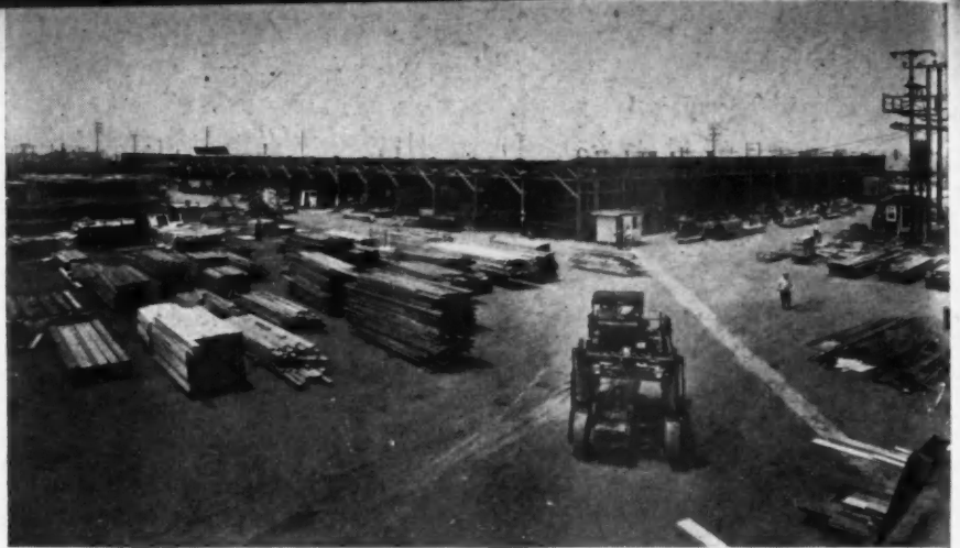
THIS is a view of the main Kaiser-Burns plant building and extensive material storage yard.
