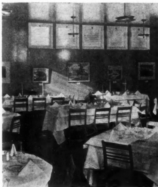
MAIN dining room. Note pictures below high windows.
