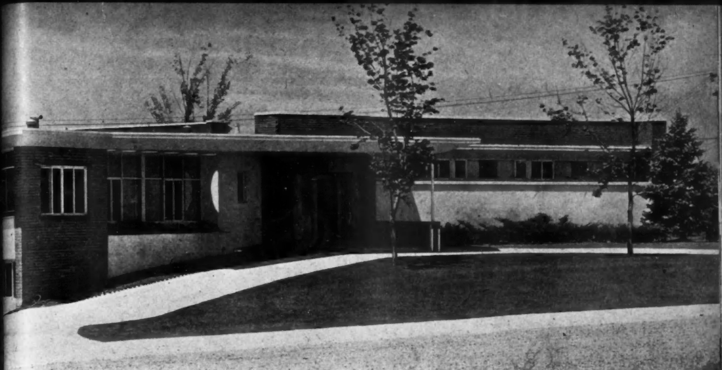
effect is obtained through a combination of brick and stucco. Circular openings in roof projection over sunroom windows add interest.
