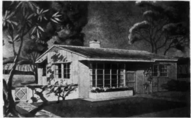
THIS house with all-metal frame will vary in cost from $3,000 to $5,000. Half-inch insulation board is used for interior finish. It will be marketed through operative builders and contractors.
