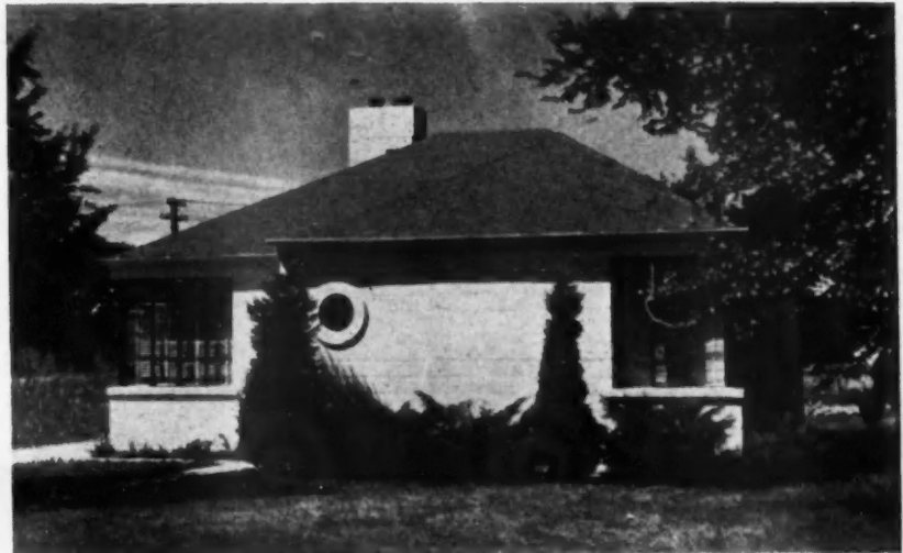
LARGE corner windows assure an abundance of light and air.
