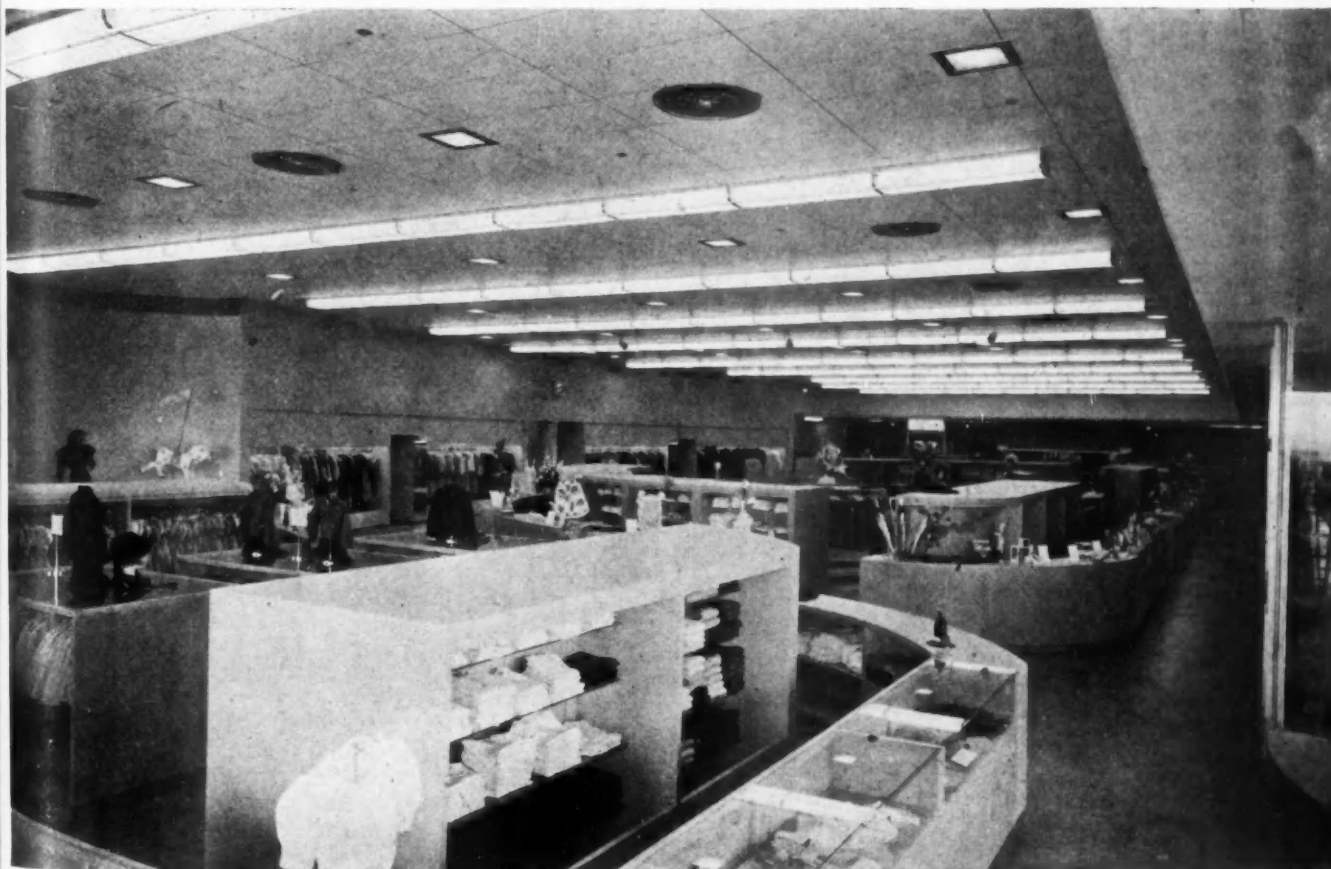
INTERIOR VIEW of department store. Absence of columns in main sales area is noteworthy. Fluorescent tubes provide balanced lighting.
