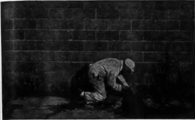
THIS IS A WET BASEMENT PROBLEM TO THE BUILDER AND HOMEOWNER
