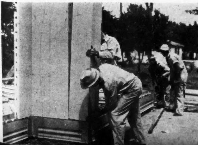
STARTING erection of exterior wall with special corner panels.
