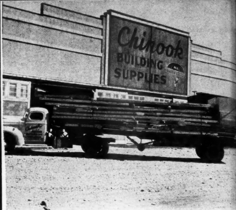
CHINOOK uses trucks to transport prefabricated sections to site.
