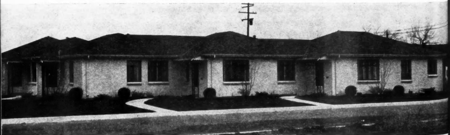
BELOW is a view on side street, following a similar pattern obtaining on opposite side, providing a large interior service court.
