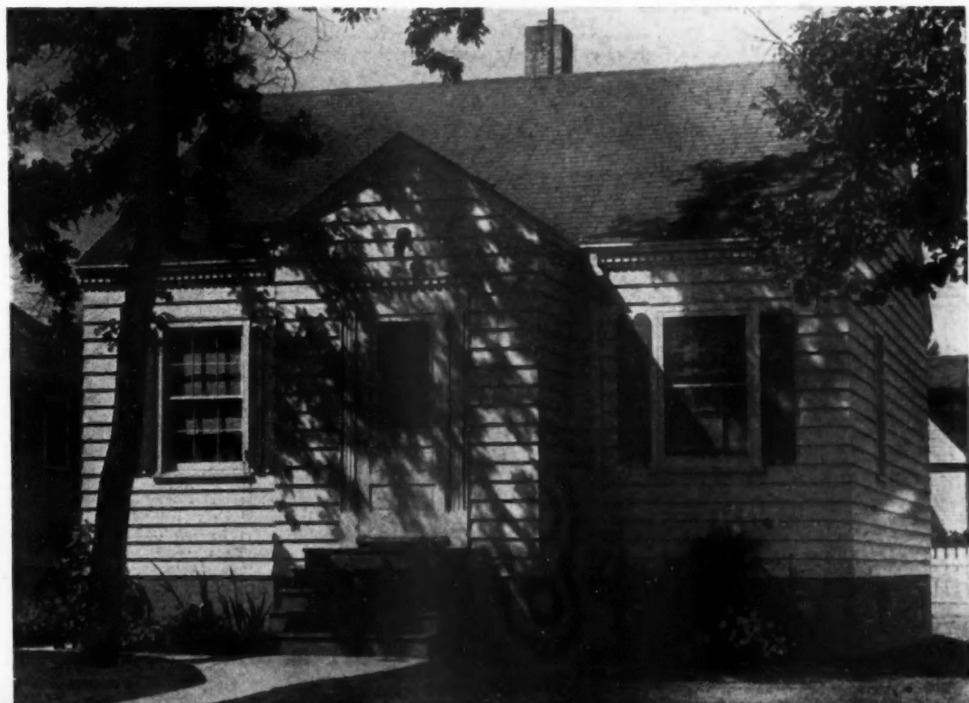
RIGHT: One of the hundreds of "Precision-Made" homes prefabricated before the war by North American Buildings, Ltd. Manufactured in four sizes, each with several floor plans, "Precision-Made" homes utilize room-length panels for exterior walls, and usually have full basements.
