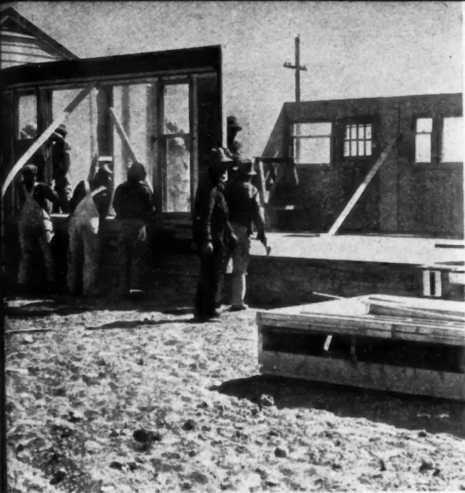
ON-SITE assembly of Chinook wall panels is speedily accomplished.
