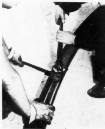
AB2641 *—This close-up view shows the assembly of a semi-circular rib unit of Stran-Steel's arch-rib framing. Developed by the Great Lakes Steel Corporation, Stran-Steel Division, this construction permits economies, and unique flexibility.
