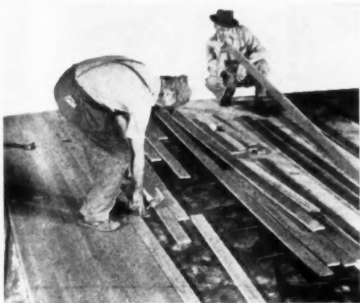
AB 2615—Shown above, Bradley pre-finished straight-line flooring is manufactured in oak, beech and pecan. Factory finishing by assembly line methods supplies a floor of amazingly superior workmanship and appearance at a very definite saving in time and in cost over hand-laying and hand-finishing on the job.
