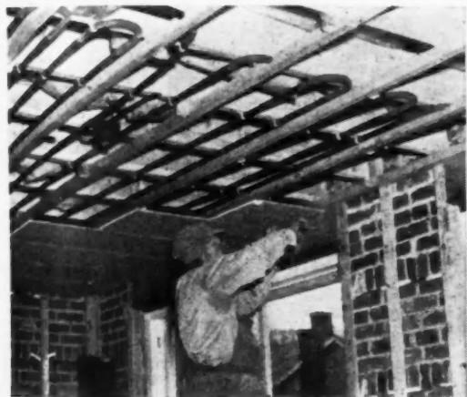
AB 2617—Bethlehem Steel Company's Ammonduct pipe, originally designed for the refrigeration industry, offers distinct advantages in radiant heating installations like the above due to its unusual bending properties.
