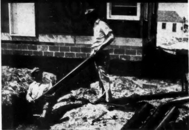
ORANGEBURG PIPE being installed in a 75 home housing project in Indiana
