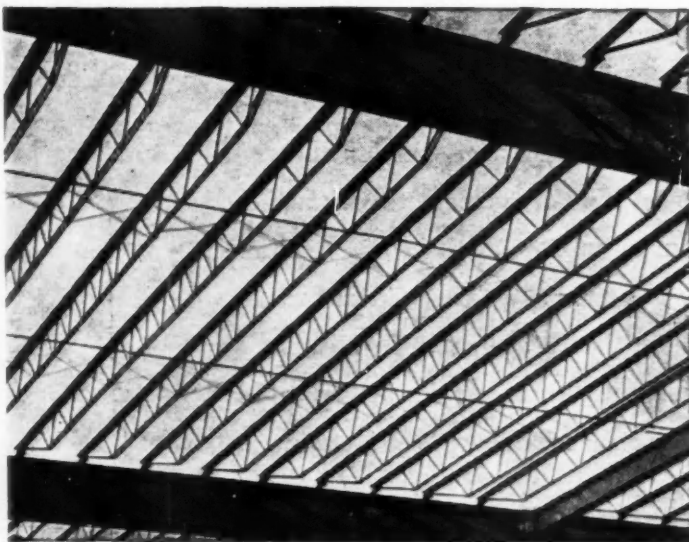
Simplicity of construction is made possible by Ceco steel joists. No skill is needed in placing them. They are easily moved into position and quickly spaced. After bridging, floor and ceiling are installed.
