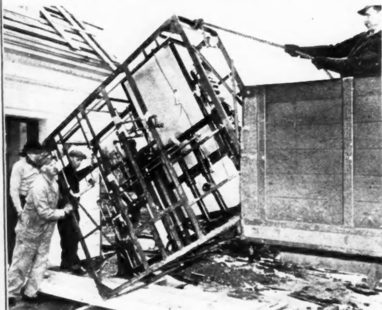
IN seven minutes, unloading crew of four men lowers Ingersoll utility unit core to a prepared position on the ground floor of one of the homes in the Ingersoll subdivision at Kalamazoo, Mich.
