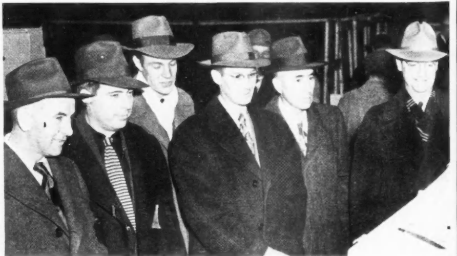
WATCHING production of kitchen cabinets are the following Cleveland builders: Charles Keyes, James K. Chandler, Peter Kleist, Will Marquard, Alex Truehaft and Hugh Selby.
