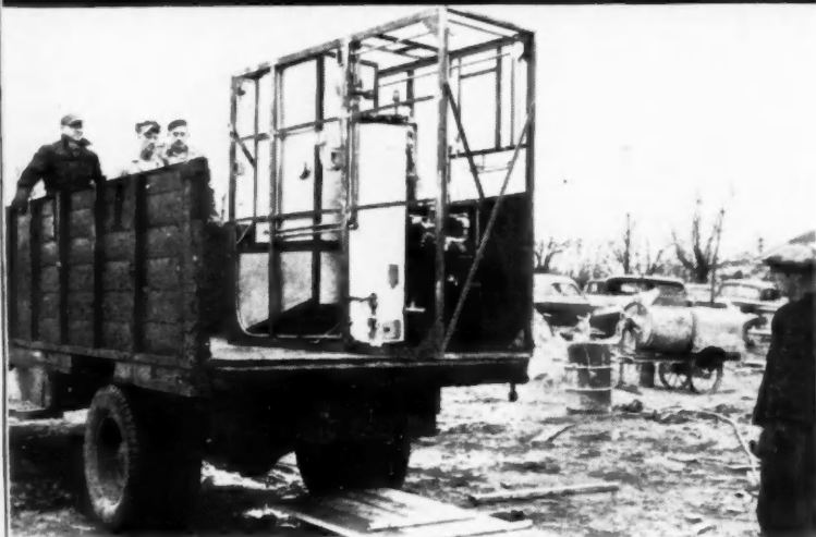
INGERSOLL UTILITY UNIT core ready to unload at front door as it comes from factory. Already installed in this one compact frame are: furnace, hot water heater, plumbing and sewer connections, copper gas and water lines, electrical conduits and control boxes.
