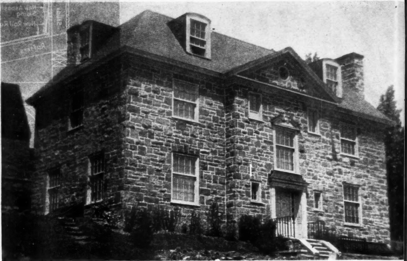
DISTINGUISHING characteristics of the pure Georgian type are illustrated in the large house above. Front entrance in exact center of elevation, windows grouped symmetrically around it—an arrangement which sets it apart from less formal types.
