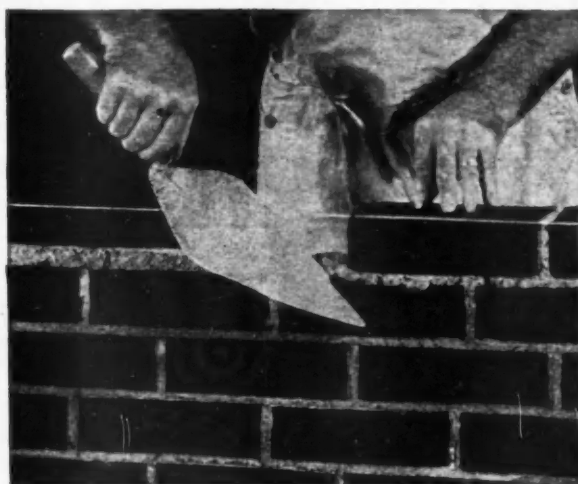
To make a good bond with the brick, mortar must be plastic, and stay plastic until the brick is bedded. The two photographs above show a good comparative test for plasticity—hence for bond. Try this with Brixment mortar!
