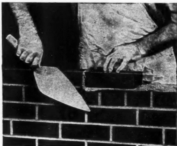
To make a good bond with the brick, mortar must be plastic, and stay plastic until the brick is bedded. The two photographs above show a good comparative test for plasticity—hence for bond. Try this with Brixment mortar!
