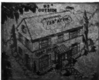
Inside temperature higher than outside. Attic temperature 120 to 130 degrees. No wonder the house is "like a bake-oven."
