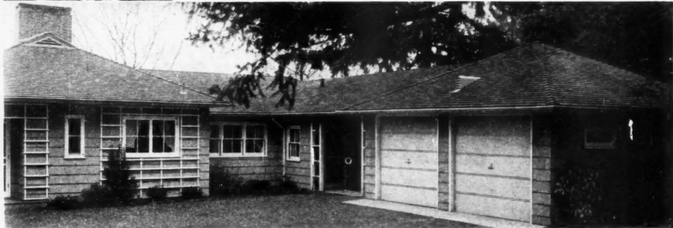
Home of Mrs. W. T. Patten, Vancouver, Wash. • Glenn Stanton, Architect.
