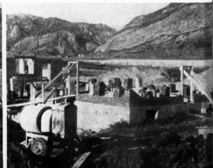
4 MASONS follow along without delay, laying up brick with block back-up. Note progress on next house at left. 5
