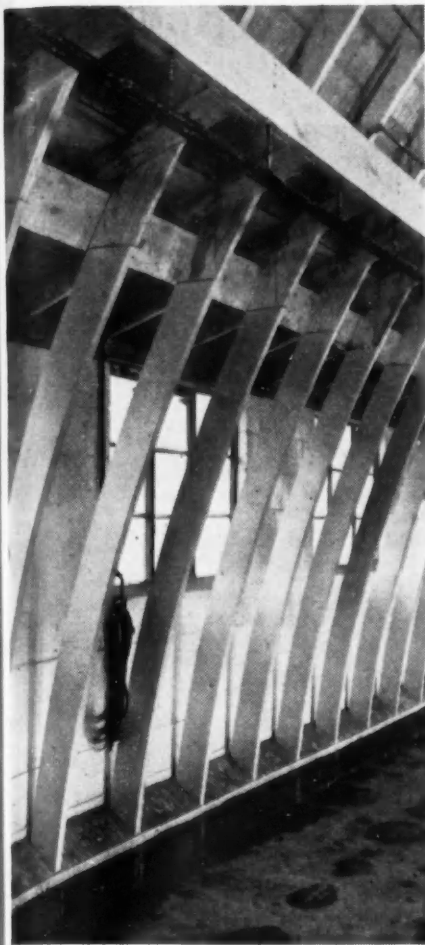
CLOSE UP of side-wall construction showing the glued-up laminated barn rafters.
