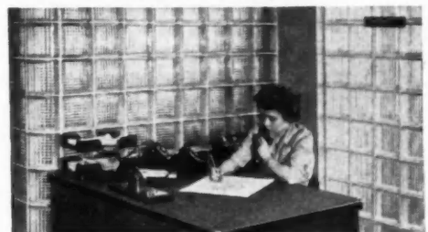
Building Managers use partitions of Insulux to transmit natural daylight from office to office.
