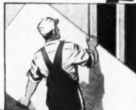
OUTSIDE THE STUDS, Insulite Bildrite Sheathing. The large boards provide a wind-proofed, weather-tight wall. Bildrite Sheathing has a bracing strength four times that of wood sheathing, horizontally applied.
