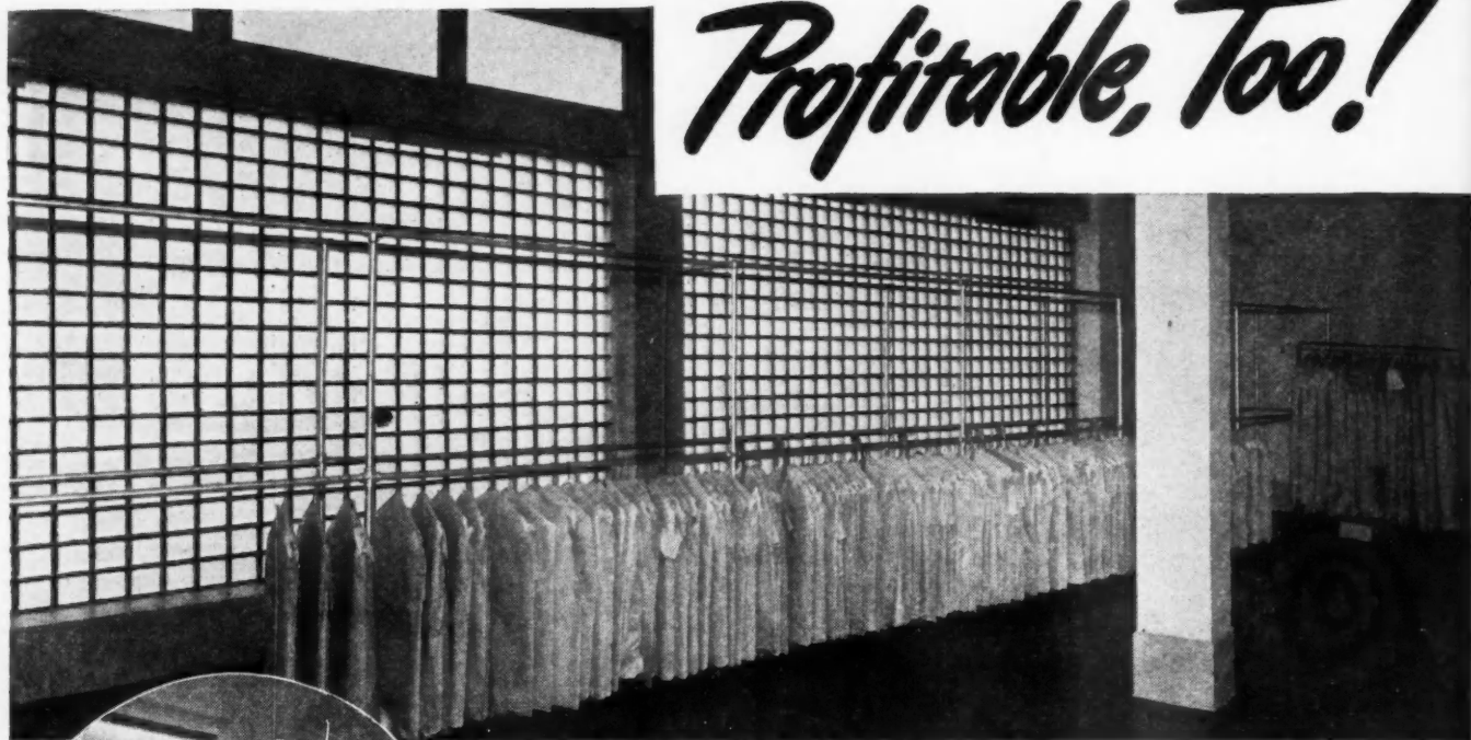
In Stores —Panels of Insulux can give salesrooms controlled natural daylighting.
