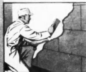
INSIDE THE STUDS, Sealed Lok-Joint Lath, furnishes a second wall of insulation. The patented Lok-Joint provides a strong, rigid plastering surface, prevents joints from opening under trowel pressure.
