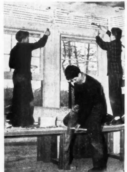
RIGHT: Doing carpentry in one of the rooms are, left to right Jerry Moore, John Bentz and Charles Hoins. Notice the old fashioned wood lath to be replastered.
