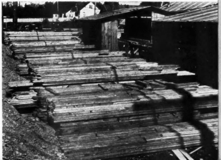
ABOVE: Double set-up of saws and roller bench handles angle cutting at both rafter ends without reversing on Puget Sound Bridge & Dredging housing job. RIGHT, handy lumber buggy (made from an old concreting cart) transfers finished work to stock piles. BELOW, stock piles of cut-to-fit rafters, each unit one complete roof, ready to be trucked as needed.
