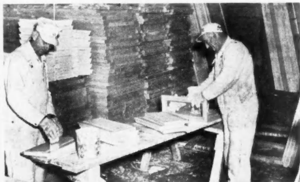
KITCHEN CABINETS, porch brackets and other special millwork are turned out in this temporary power-shop building (above) at the job site. Color priming of vent panels (left) is done under cover in a dry, heated warehouse shed, 24 by 100 feet, where the Curtis Silentite window frames and sash and the Wheeler-Osgood Tru-Sized doors are stored.
