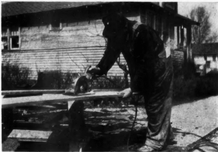
PORTABLE power tools used on remodeling and conversion jobs do much to keep the cost of labor at a minimum. Here is a saw ripping an 18-foot board in 1-20th the time it would have taken by hand sawing.
