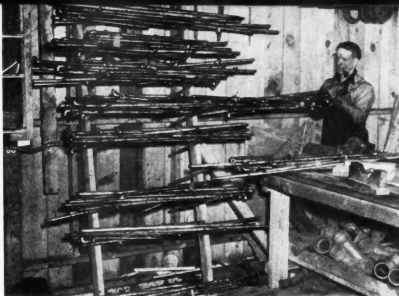
PIPE AND PLUMBING SHOP, with power cutting and threading machine, cuts costs. Each wired bundle on rack (above) contains everything needed for complete water piping for one house. Sanitary piping loops and other pipe assemblies also are made ready in this shop. Window frames are stacked ready for delivery.
