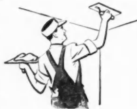
ACOUSTICAL PLASTER FINISH
