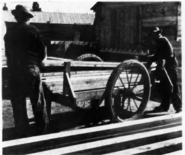
ABOVE: Double set-up of saws and roller bench handles angle cutting at both rafter ends without reversing on Puget Sound Bridge & Dredging housing job. RIGHT, handy lumber buggy (made from an old concreting cart) transfers finished work to stock piles. BELOW, stock piles of cut-to-fit rafters, each unit one complete roof, ready to be trucked as needed.
