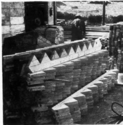
PIPE AND PLUMBING SHOP, with power cutting and threading machine, cuts costs. Each wired bundle on rack (above) contains everything needed for complete water piping for one house. Sanitary piping loops and other pipe assemblies also are made ready in this shop. Window frames are stacked ready for delivery.
