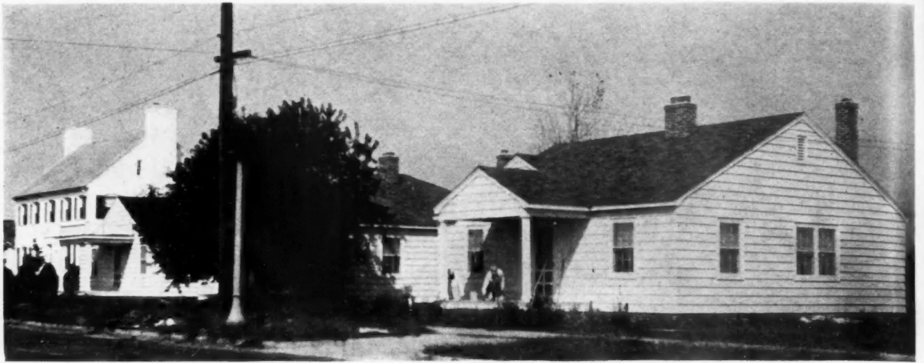
POPULAR small town war homes built by Lex Marsh of Charlotte, N. C., fit into variety of communities. Above, several are shown on an attractive street adjacent to higher priced property.
