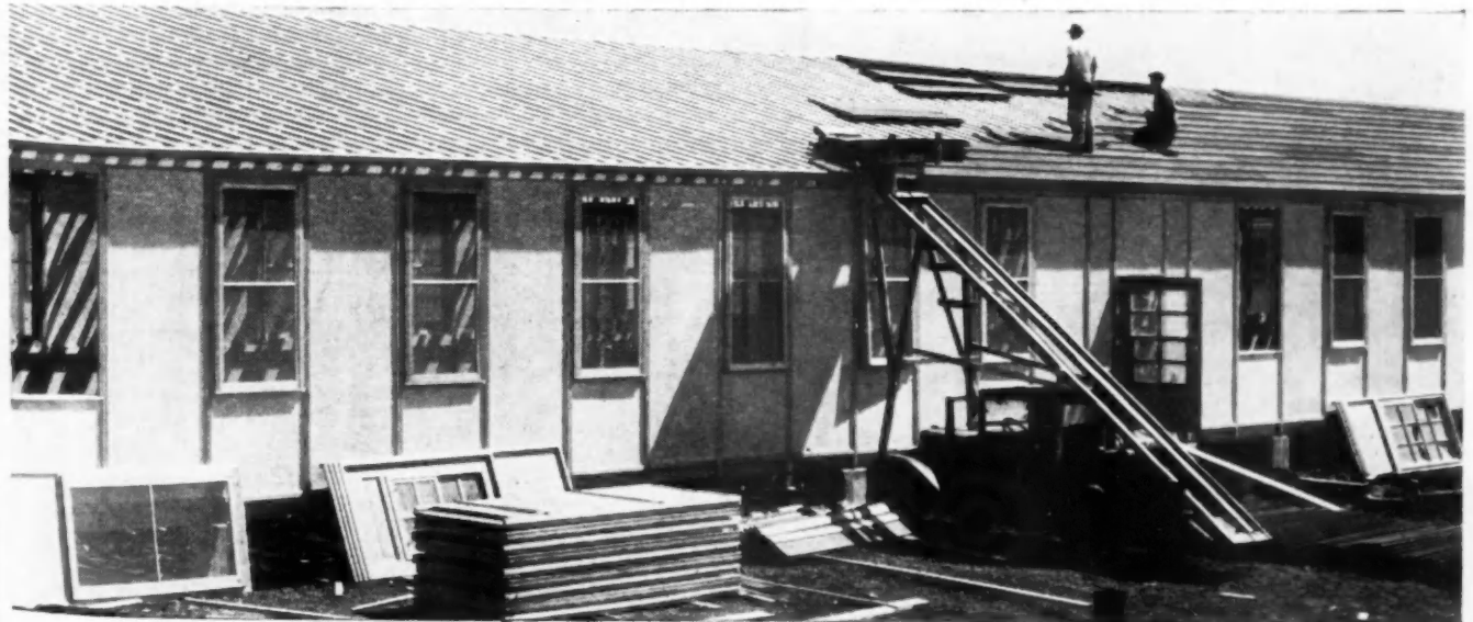
ISOMETRIC DRAWING above shows parts assembly of Modulok system of prefabrication. Details indicate rails at sill and assembly of panels at plate, cornice and roofing units. Below, Navy hospital ward building, 28 by 212 feet, being assembled; panels are ready to be set in place equipped with sash, doors, screens, hardware. Eight-foot shingles are being laid on diagonal sheathing.
