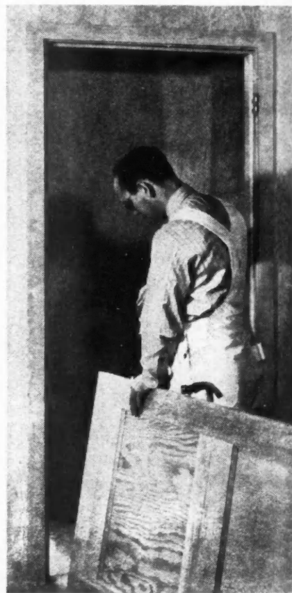
INSTALLING pre-fit "Tru-Sized" door.
