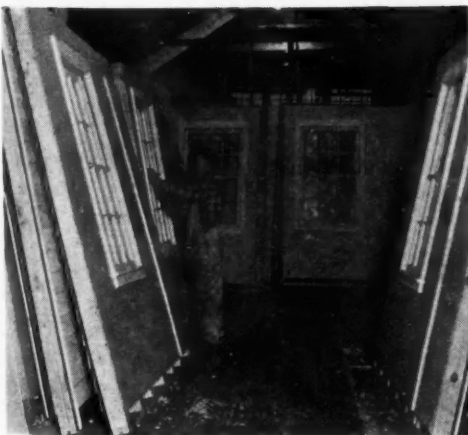
Wall sections are complete in every detail, including wiring. A splined joint and top plate hold them together in rigid form.
