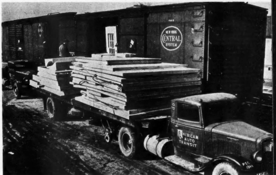
AT DAYTON, O., box car load of house panels is put on trailer truck for delivery to site where they were quickly erected as homes for airport workers.
