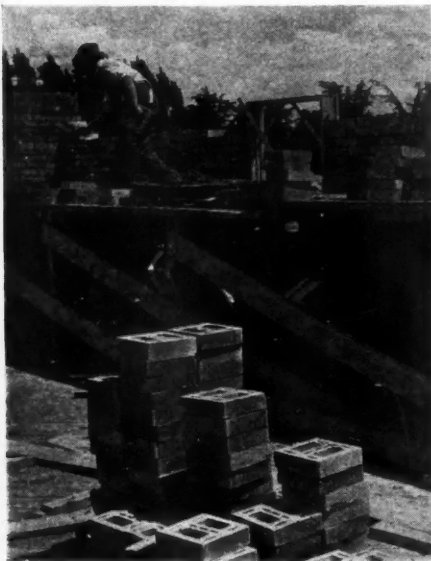
LEFT: Workman laying up masonry walls of a Canadian house in their privately financed program; note 8" x 8" air cell brick used.
