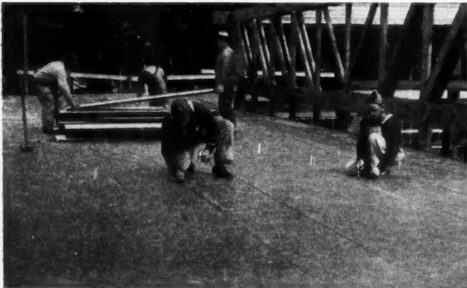
For flat or pitched roof decks. The moment the sturdy gypsum planks are nailed in place, the roofers move in. No waiting for materials to dry!
