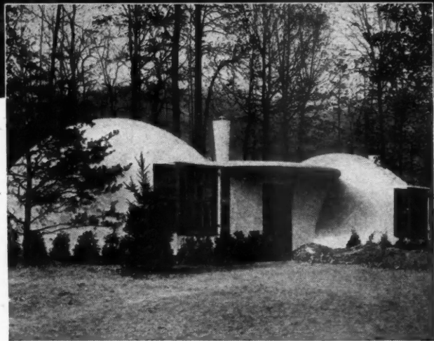
These so-called "bubble houses" at Falls Church, Va., were needed in a hurry. Concrete made with Lehigh Early Strength Cement was shot on inflated balloons with a cement gun. Curing time was saved. Balloons were deflated and re-used in a few hours.
