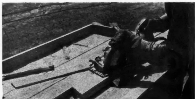
ROLLER TABLES connect saws in Bohannon's cutting yard. Eave end cut and plumb cut at seat are made on saw No. 1. Plumb cut at ridge or jack cut are made on saw No. 2. Rafter seat cut is made on handsaw in foreground, No. 3.
