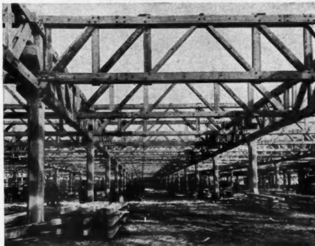
Teco Connector-built trusses in a war plant, Somewhere, South
