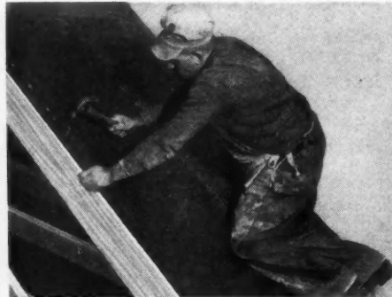
Gold Bond Roof Plank. For flat or pitched roofs. Nails directly to wood joists. Forms perfect base for roofing material. Fireproof. Weatherproofed.
