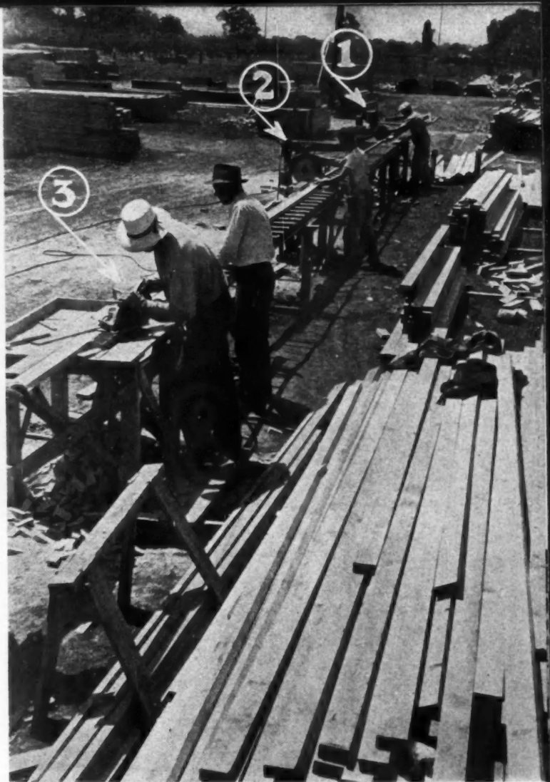
ROLLER TABLES connect saws in Bohannon's cutting yard. Eave end cut and plumb cut at seat are made on saw No. 1. Plumb cut at ridge or jack cut are made on saw No. 2. Rafter seat cut is made on handsaw in foreground, No. 3.
