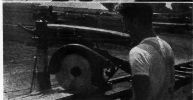
SEAT CUT is made with hand saw (top) guided by template. Plumb cut at ridge is made on saw No. 2. This power saw set-up made a production record, turned out four hundred rafters per hour.
