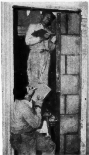
NEW chimney goes in.
