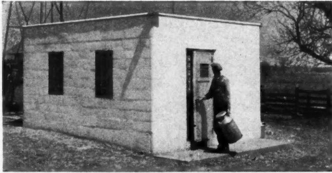
Concrete masonry milk houses and concrete cooling tanks help dairy farmers meet Army sanitation requirements and new, rigid city milk codes.
