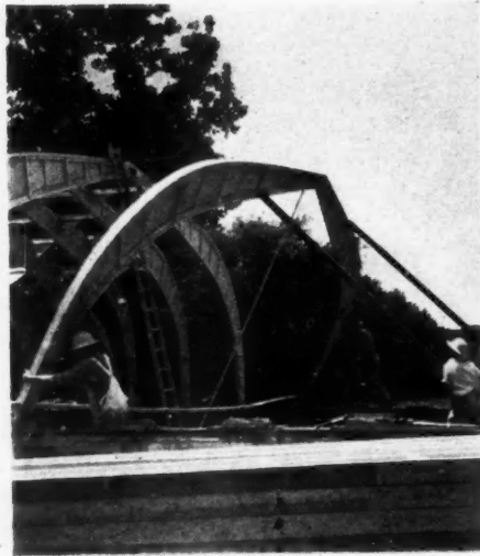
GLUED-UP arch I-beams with laminated cap strips and a plywood web, shown in process of erection for dairy barn.
