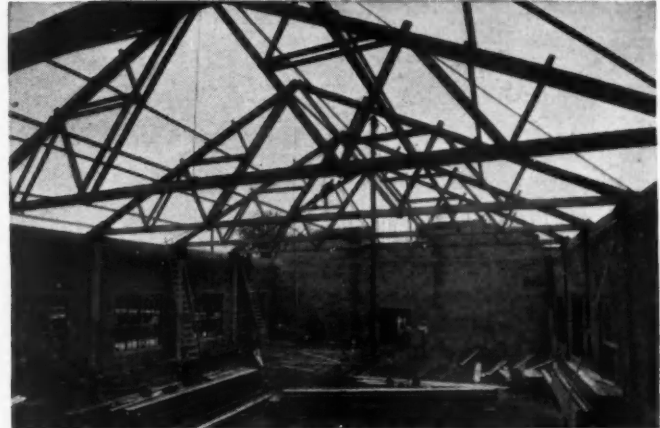
Timber trusses for this Texas structure effected saving of $730.
