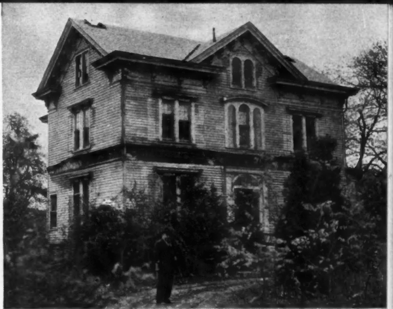
OLD Metuchen, N. J., house was a white elephant until Jake Bass came along and turned it into attractive homes for war workers.
